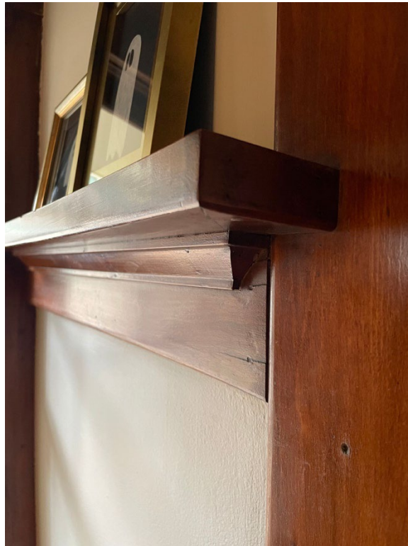
Figure 14: Detail of plate rail in dining room of the Adams House
