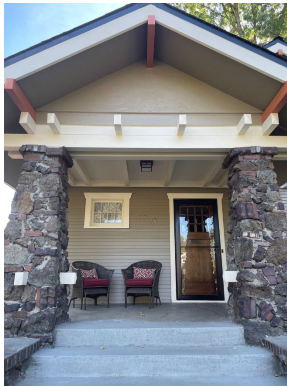
Figure 4: Porch roof and gable in 2024
