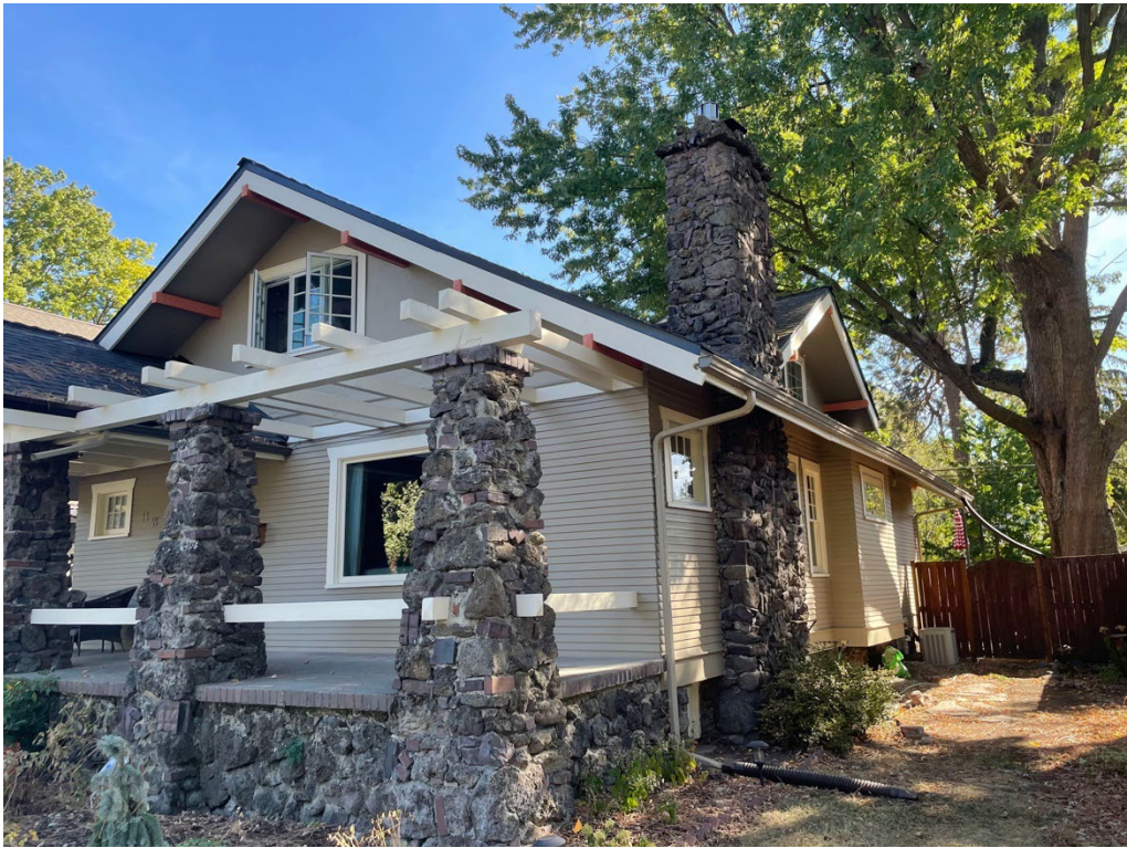
Figure 5: Adams House, northwest corner in 2024. 'Skewered' porch columns visible.
