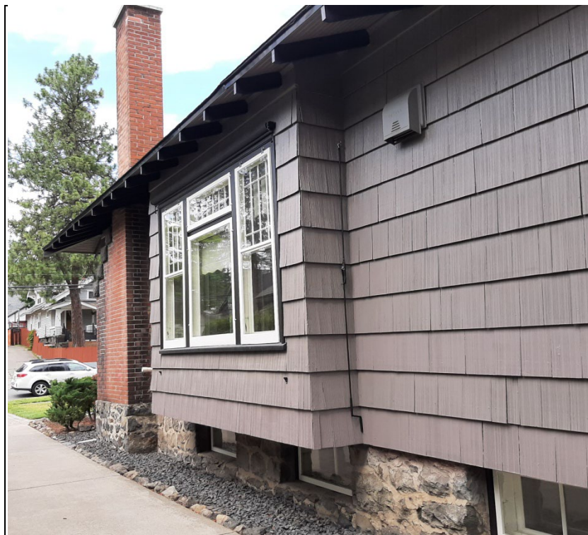
Photo 4 2024 photo of west elevation of house, looking north
