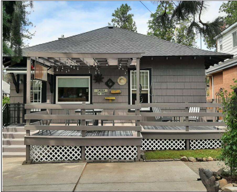
Photo 5 2024 photo of south rear elevation of house and attached wood deck
