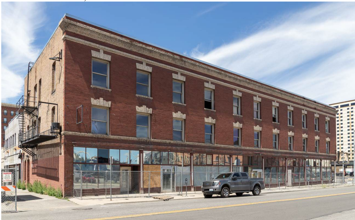
Photo 0004. Exterior, southeast corner.
