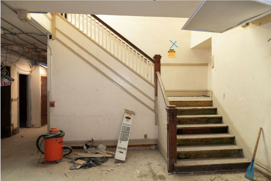
Photo 0024. Second floor, central stairwell, looking north.
