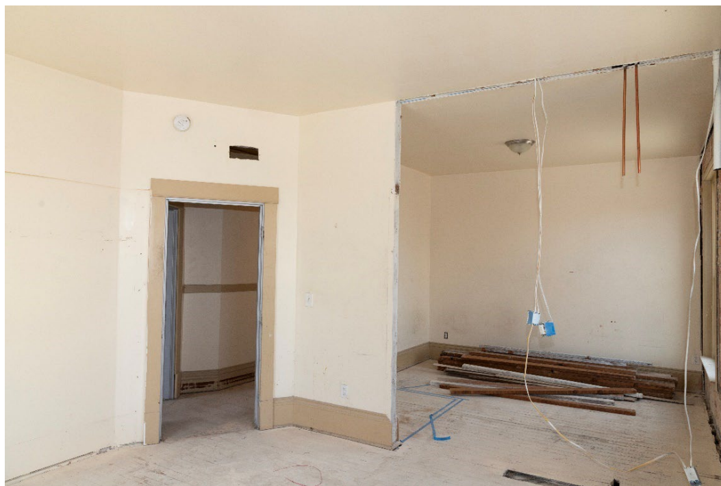
Figure 21. Third floor, showing typical unit finishes.
