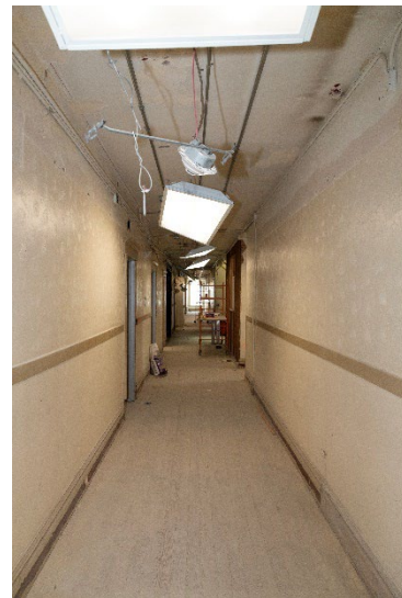
Figure 18. Second floor, main hallway.
