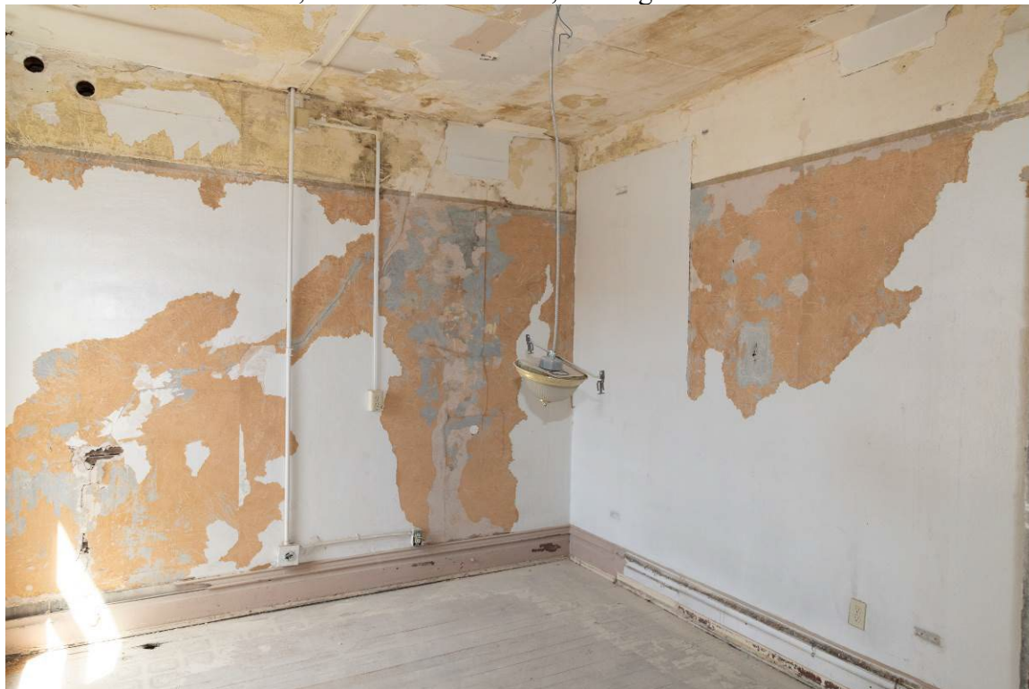
Photo 0034. Second floor, southeast corner unit, looking northwest.
