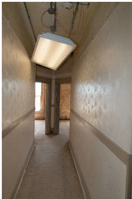
Figure 22. Third floor, typical branch hallway.
