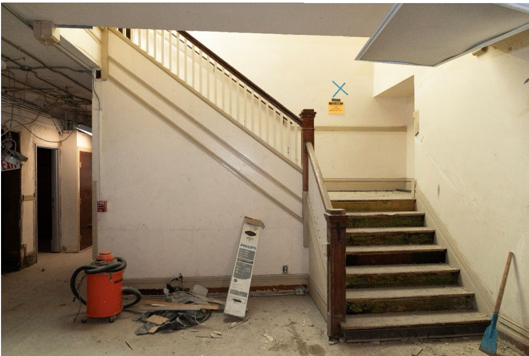
Figure 10. Central stairway, second floor, looking north showing original materials.
