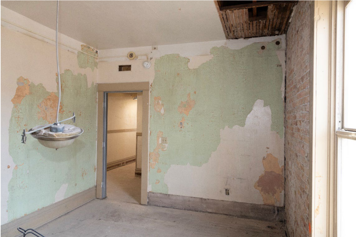
Figure 19. Second floor, showing typical unit finishes.
