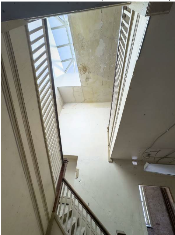
Photo 0026. Second floor, central stairwell, looking east and up.
