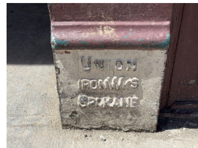
Figure 2. Cast iron pedestal detail showing factory stamp.
