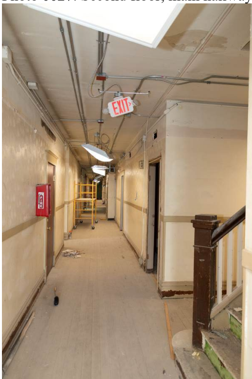
Photo 0027. Second floor, main hallway, looking south.
