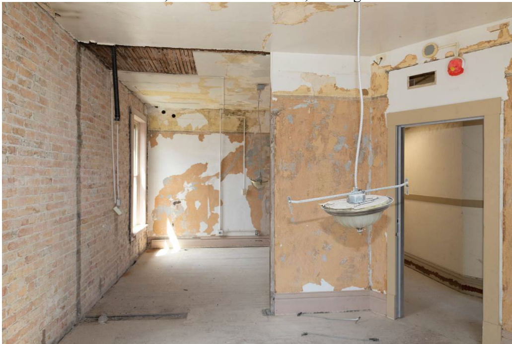
Photo 0033. Second floor, southeast corner unit, looking west.
