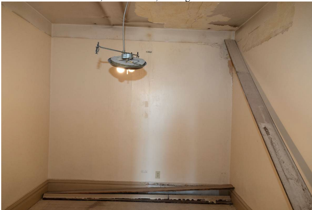
Photo 0036. Second floor, east side unit, looking west.
