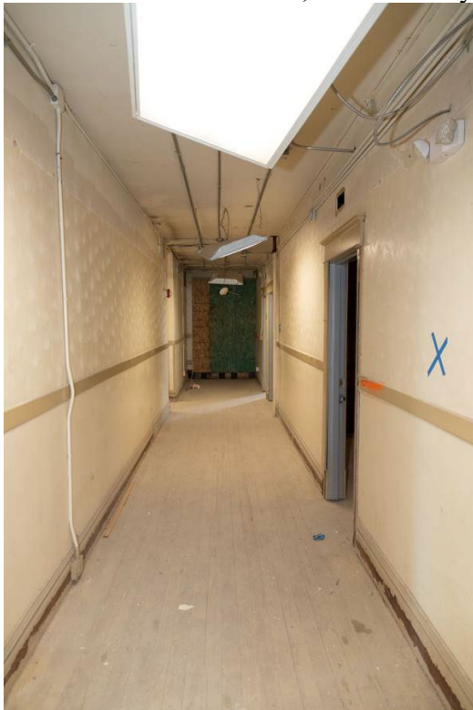
Photo 0028. Second floor, main hallway, looking south.
