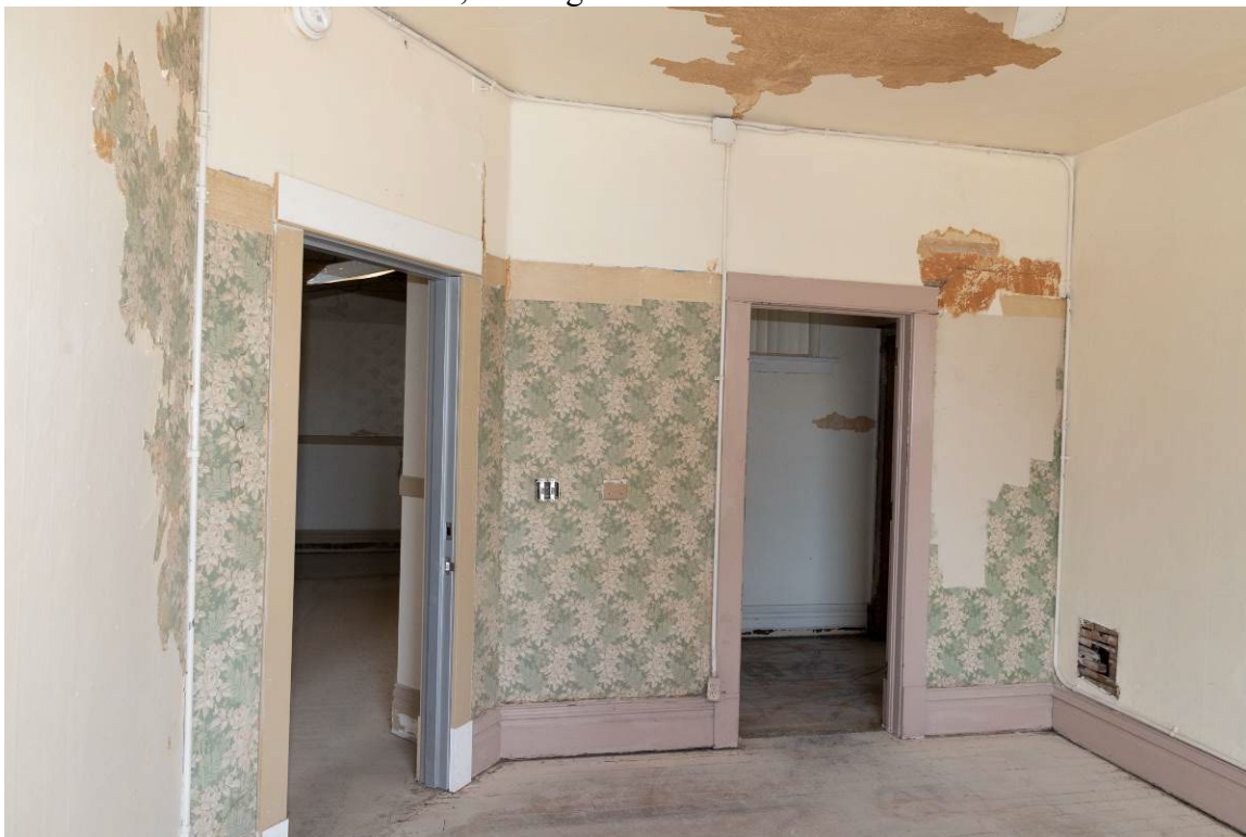
Photo 0052. Third floor east unit, looking west.
