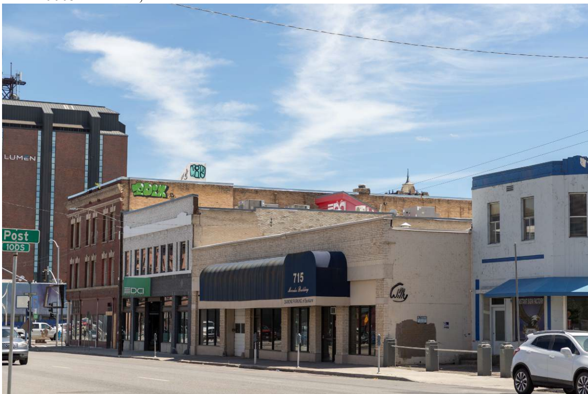
Photo 0005. Exterior, west facade.
