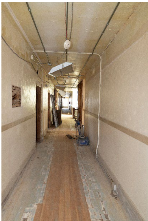
Figure 20. Third floor, main hallway.
