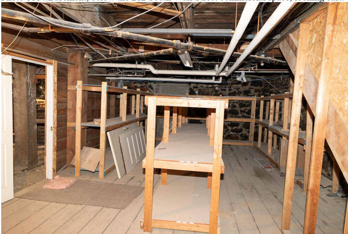
Photo 0014. Basement, below the 212 South Wall Street commercial space, looking east.
