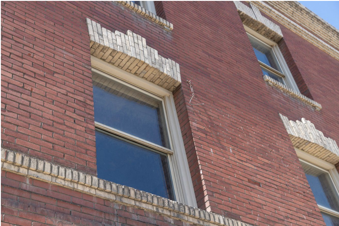
Figure 6. Second and third story windows detail.
