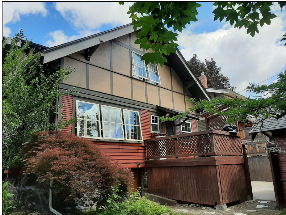
Photo 4 2024 photograph of south rear elevation of house
