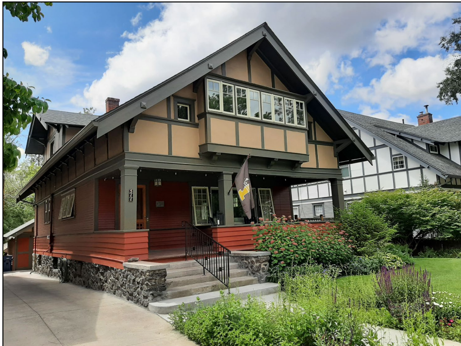
Photo 2 2024 photograph of the Mulligan-Brazeau House and its garage behind house
