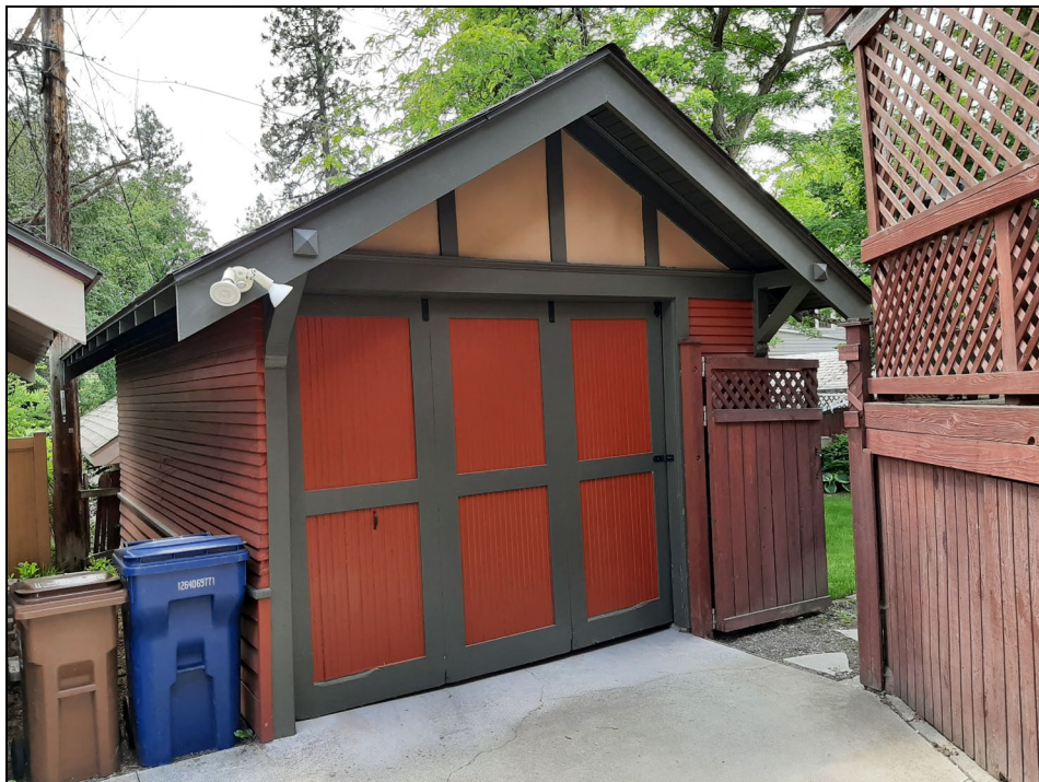
Photo 6 2024 photo of the north face of the garage in southeast corner of property
