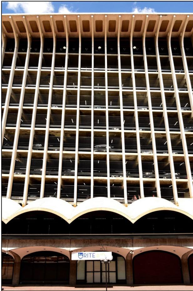
discerned on the south façade as well as the north façade. On the south façade, the edges of the floor decks, the guard rails—steel planks and steel cables, are visible in their upward slope to the west. As described above, the building is terminated with flared precast cavetto brackets supporting a concrete cornice ledge. The hipped roof is set back and only visible from a distance.
