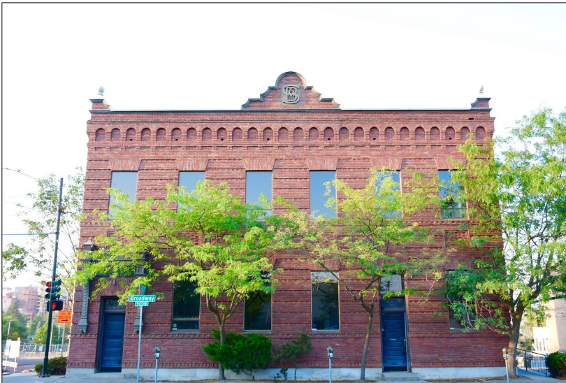
Figure 1: Front (north) facade
