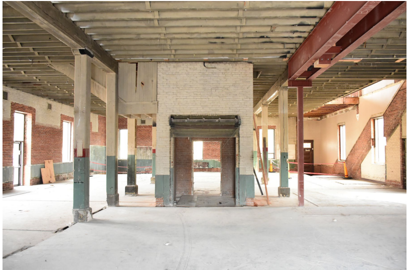
Figure 13: First floor looking north from south wall
