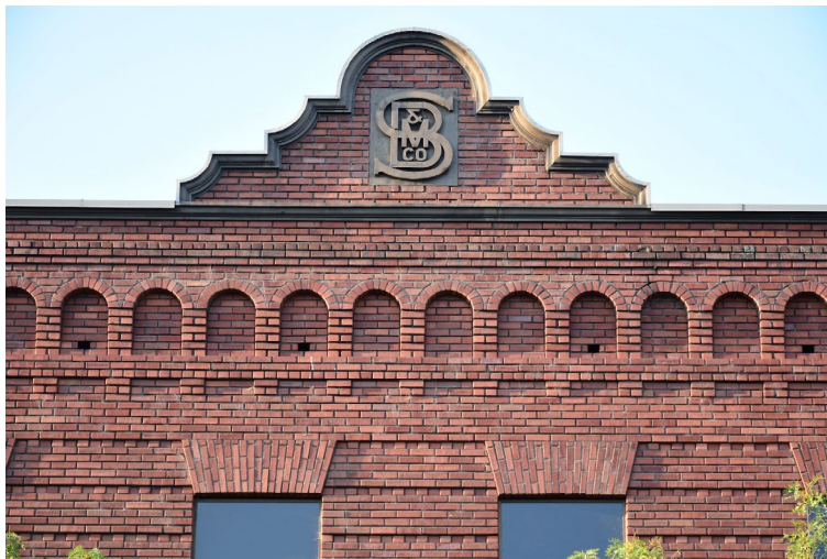
Figure 6: Central pediment detail, north elevation
