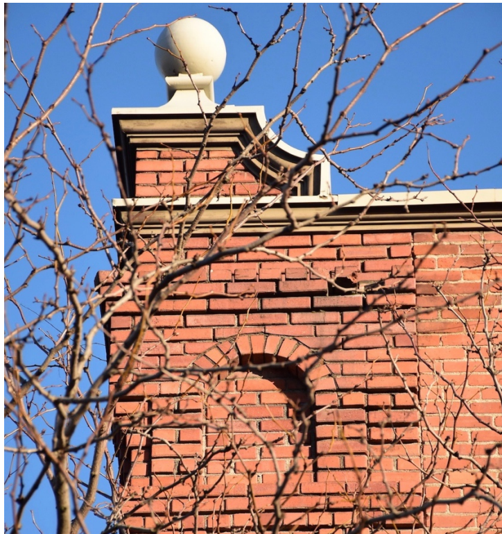
#10. Corner finial atop northwest corner, looking east
