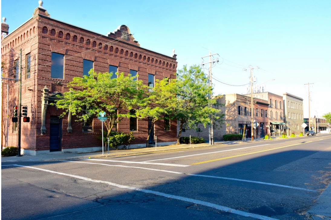
#1. Context along Broadway, looking west from Lincoln Street
