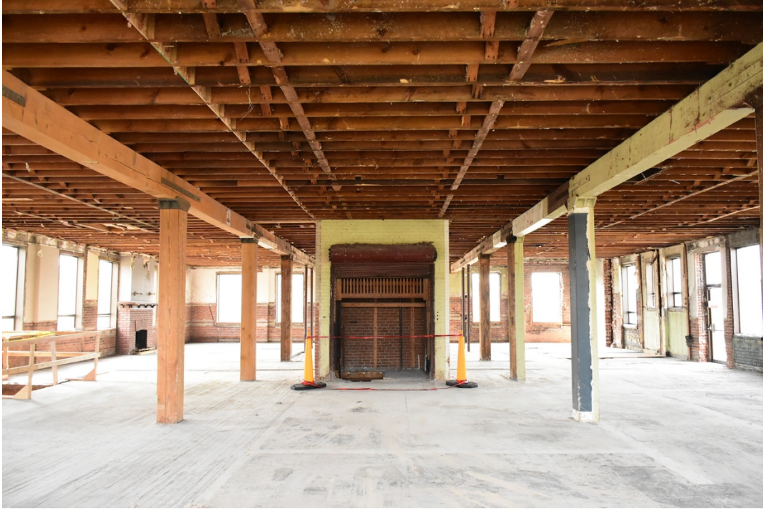
11. Second floor, looking south across room (freight elevator) from north wall
