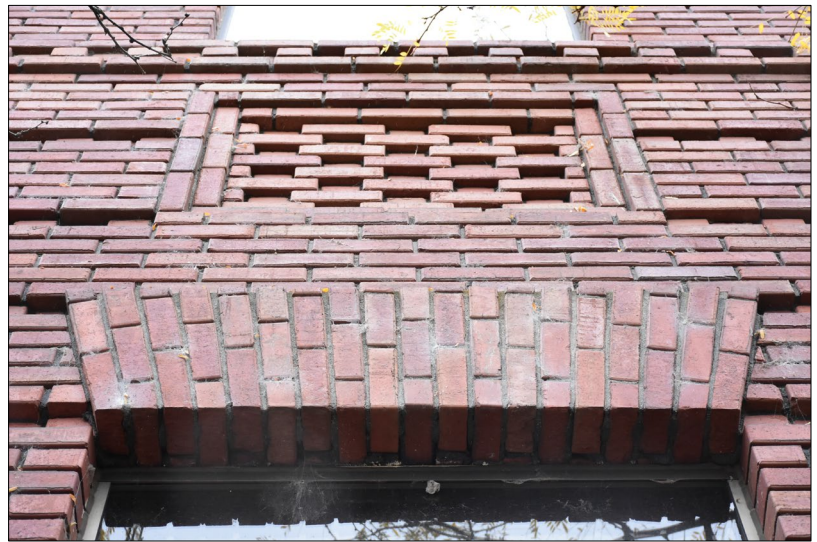
Figure 9: Window, brick detail
