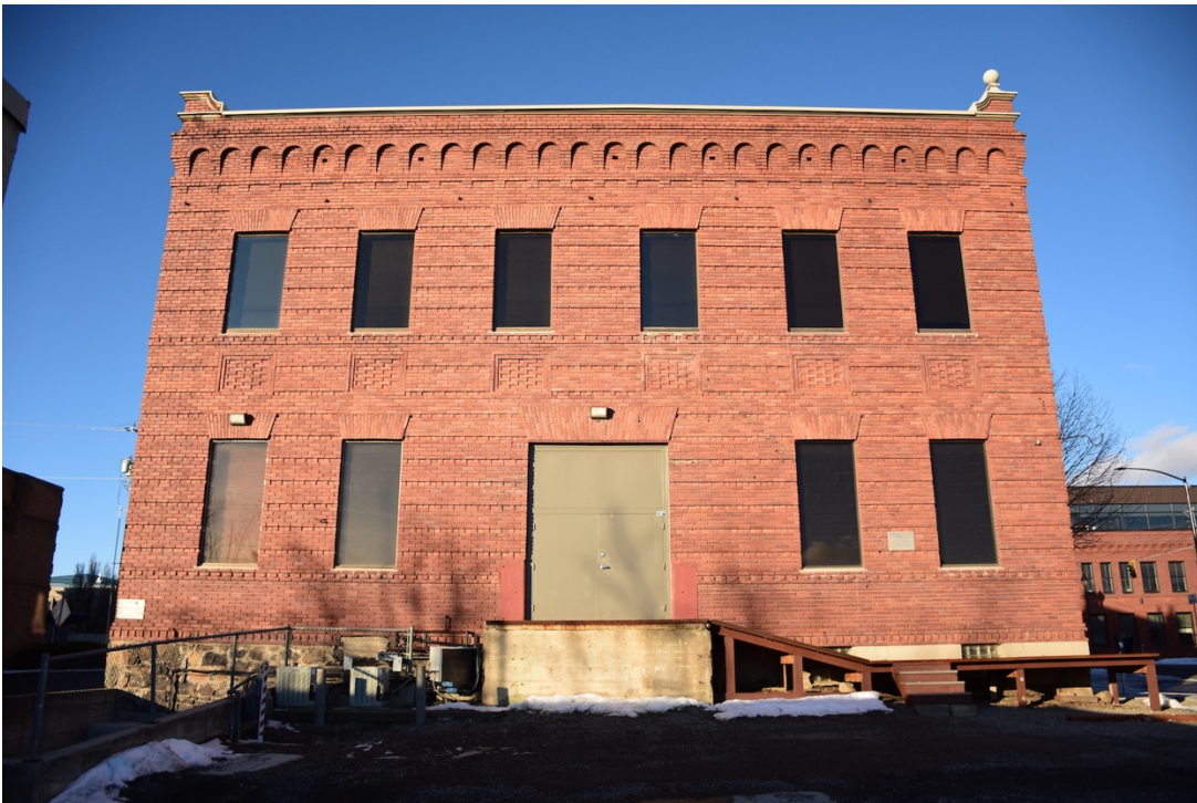
#6. South (rear) facade, looking north
