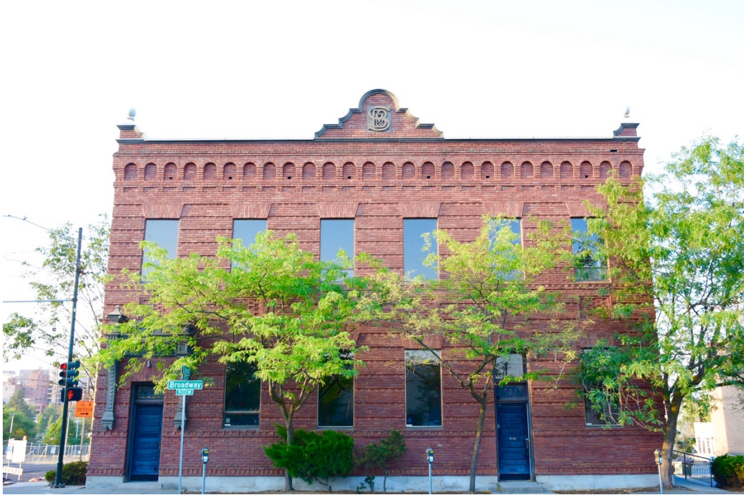
#3. Front (north) facade, looking south
