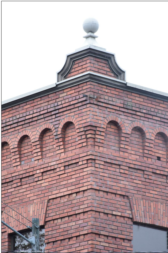
Figure 7: Corner finial detail
