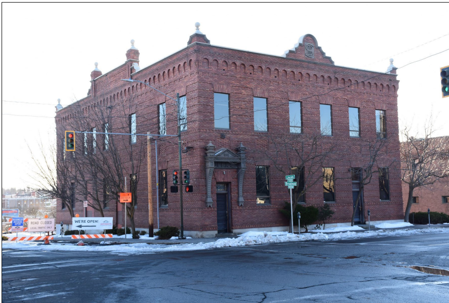
Figure 1: Spokane Brewing & Malting – Southwest corner at Broadway and Lincoln
