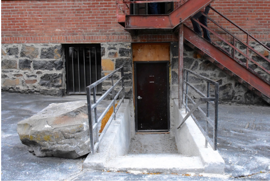
1. Entry to basement from west side.
