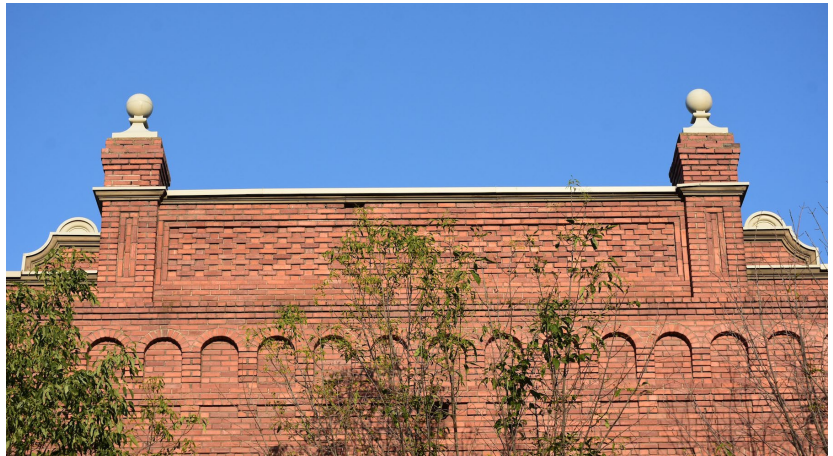
Figure 5: Parapet terminating east elevation
