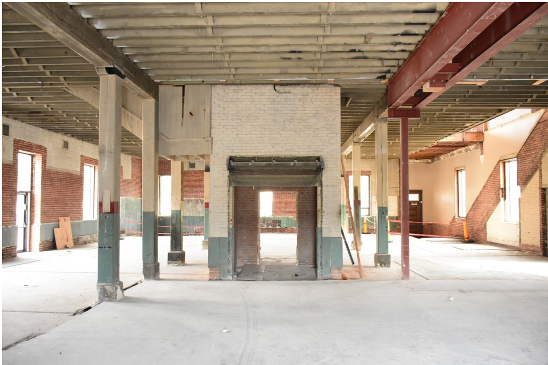
6. First floor, looking north from south wall
