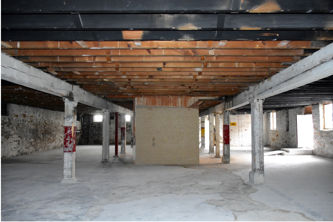
5. Basement, looking south from north wall
