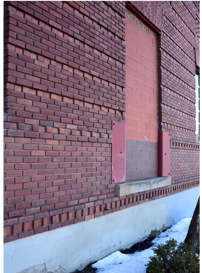
#14. Detail of east facade brickwork, looking southwest
