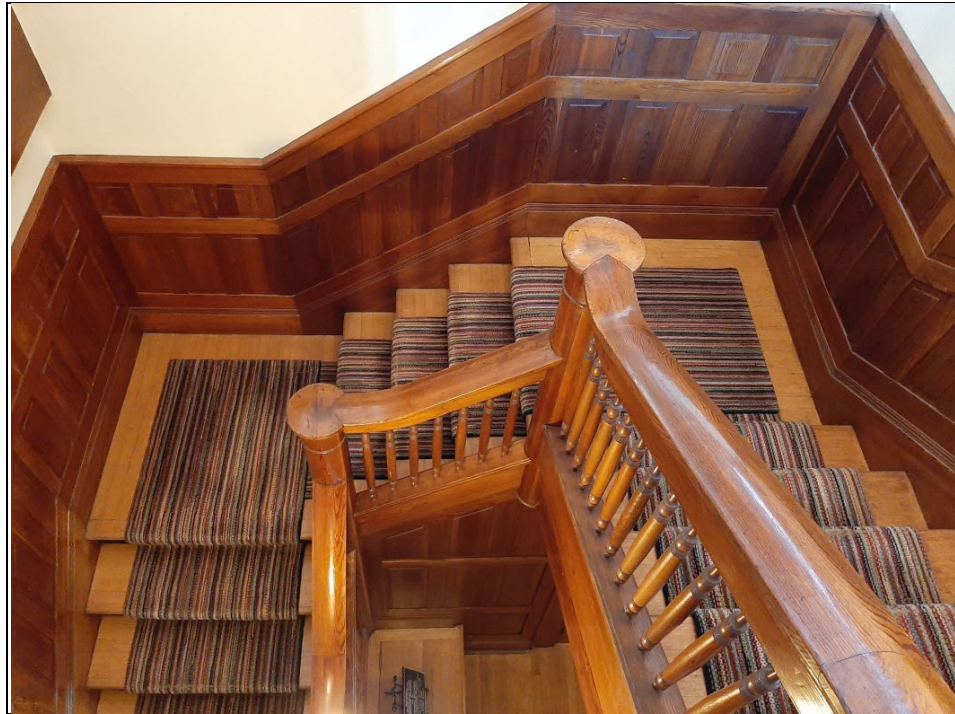
Photo 15 2022 photograph from reception hall staircase at first floor to second floor
