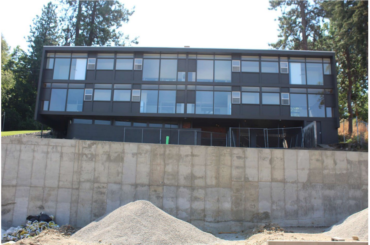
Photo 10: North façade, looking south (garage under construction in foreground)
