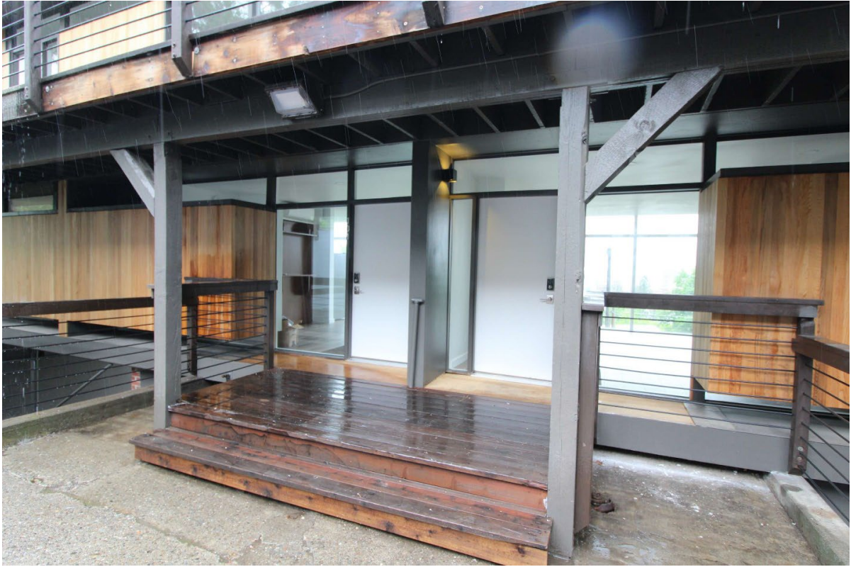
Photo 6: Front (south) façade, Units 101 and 102 entries
