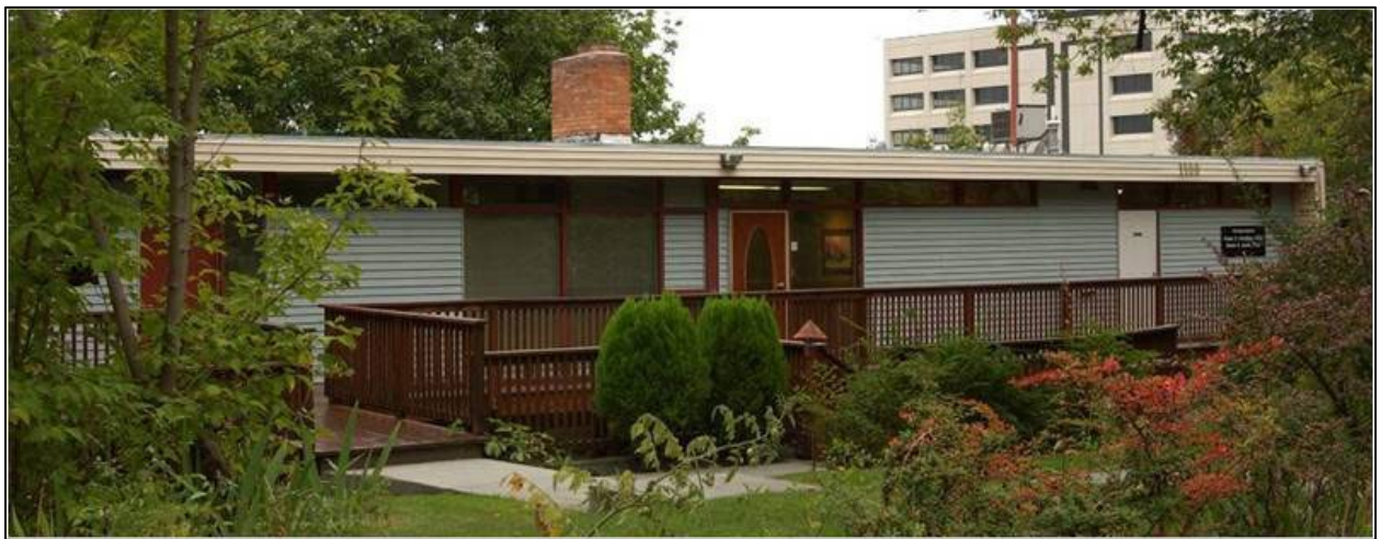
Figure 31: South façade, ca 2019
