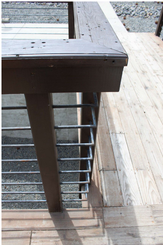
Photo 11: Balustrade detail, typical
