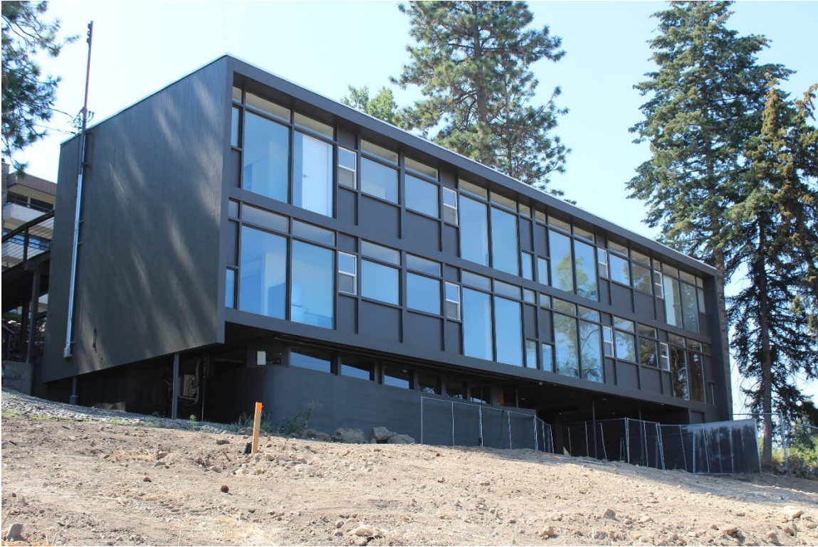
Figure 1: Studio Apartments north facade
