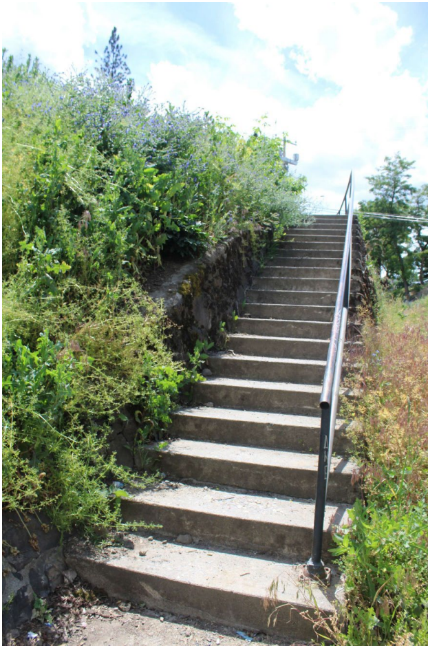
Photo 22: Stairway at 1128 W. 6 th Avenue, west of 1102 W. 6 th Avenue
