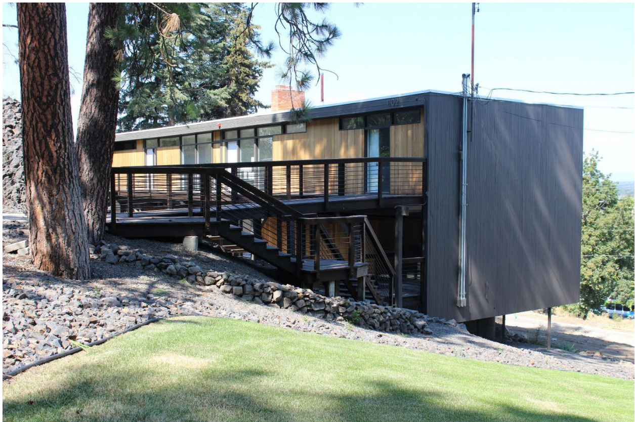
Photo 7: Front (south) façade, looking northwest
