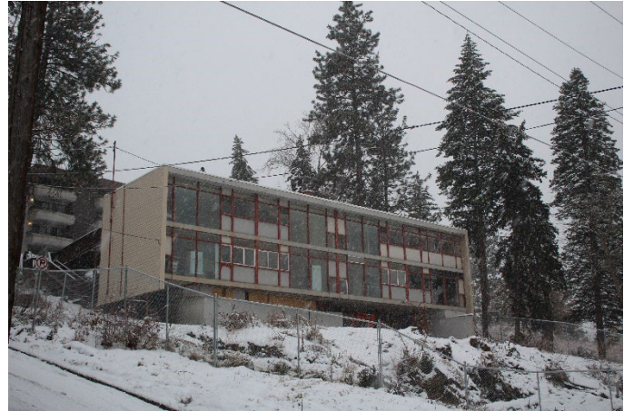
Figure 18: Appearance of the building prior to current rehabilitation
