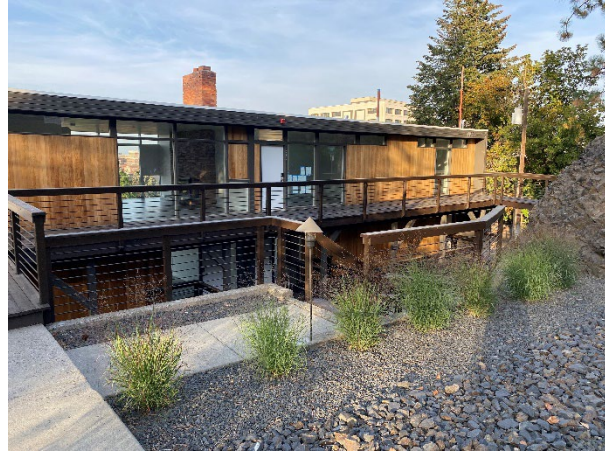
Figure 4: South elevation in 2022
