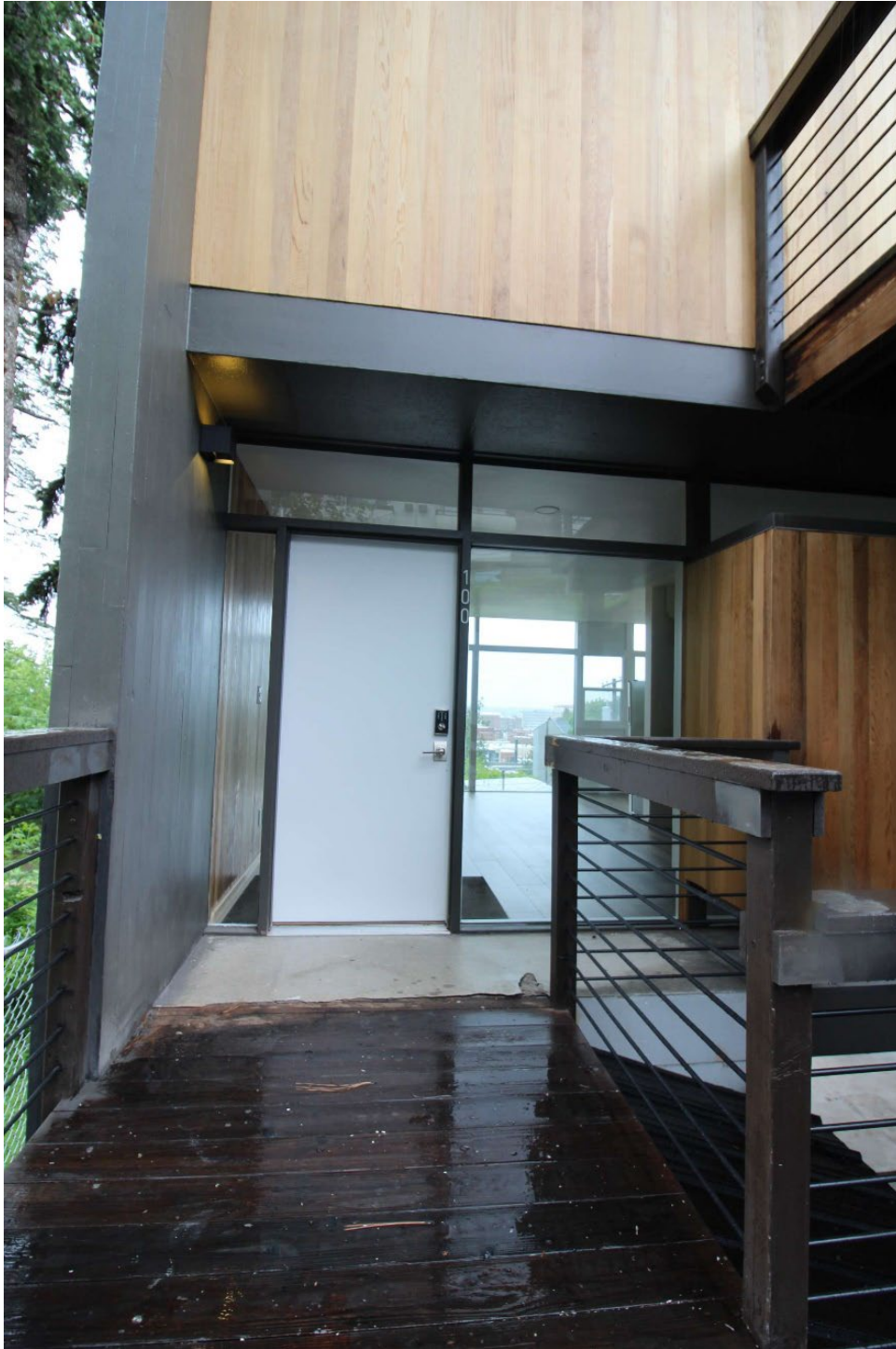
Photo 5: Front (south) façade, Unit 200 entry
