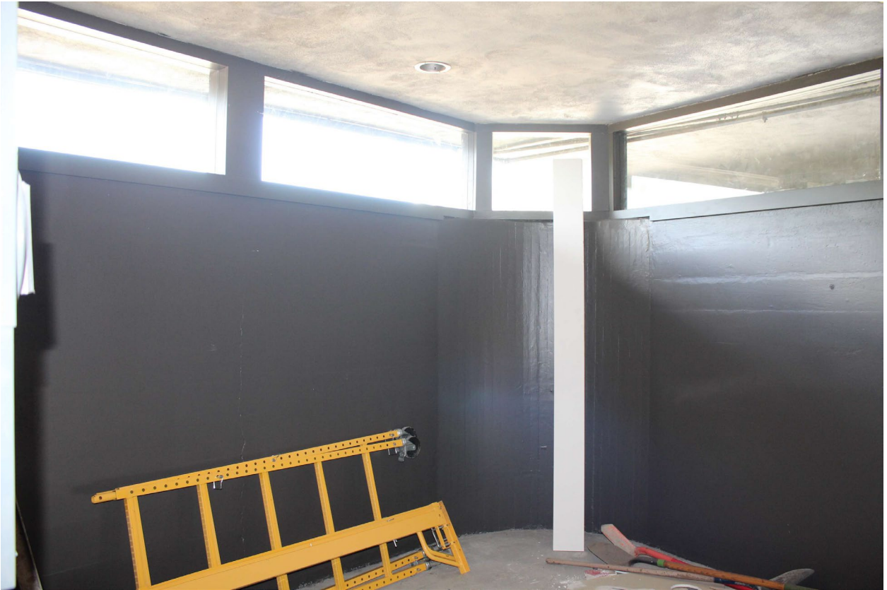
Photo 18: Basement level, northeast corner
