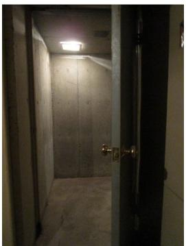
Fig. 8. Entrance to the shelter protected with a right-angle turn.
