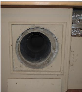
Fig. 11. Air blower in situ on the shelter wall with plumbing for toilet below it
