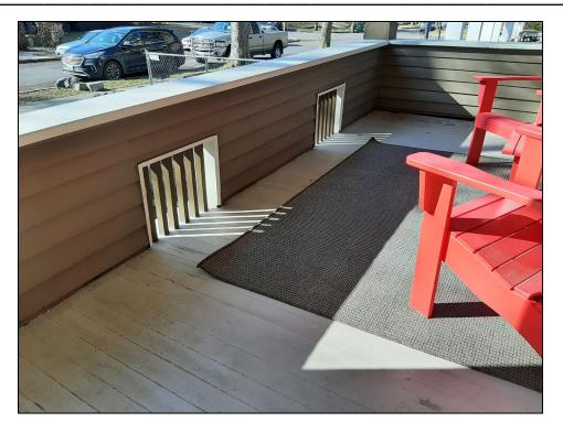
*Photo 3* 2022 photo of scupper detail on front porch
