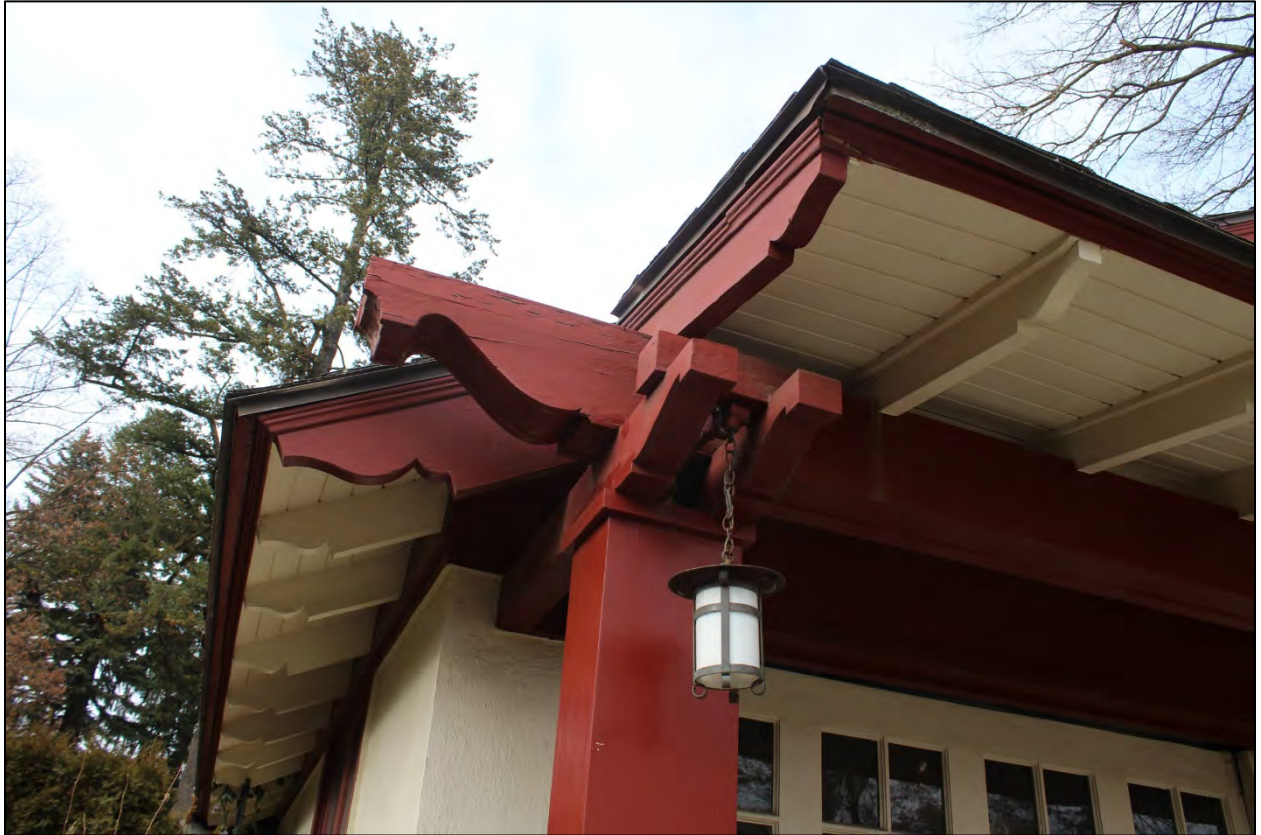
Photo 10 of 21: Garage detail
