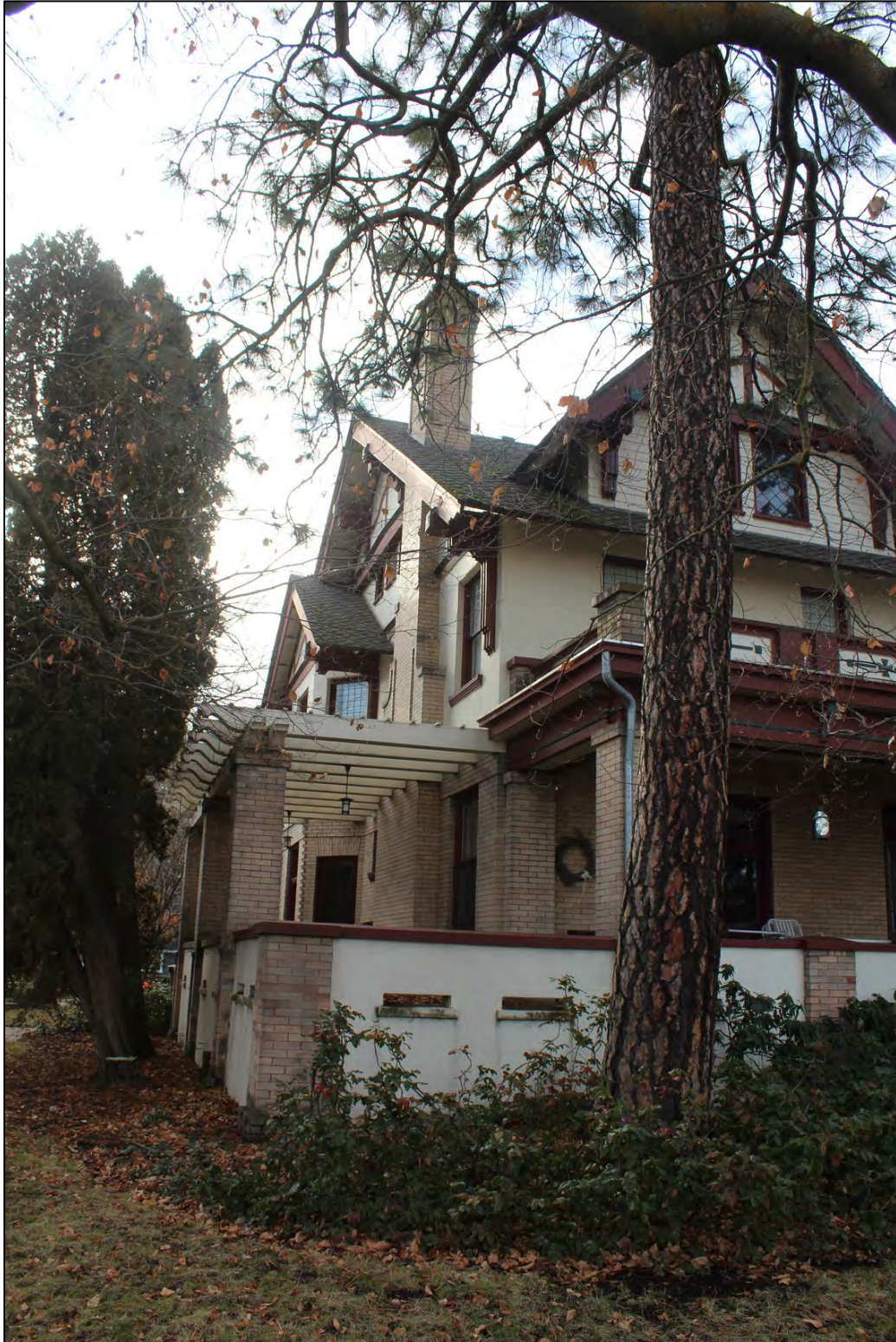
Photo 8 of 21: East side façade, looking south
