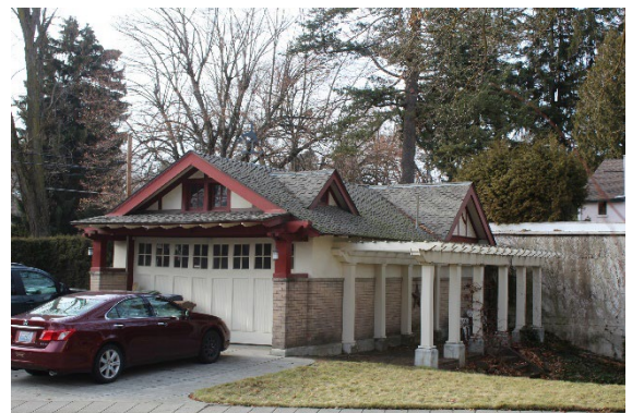
13 Garage - nearest to Sumner Avenue
