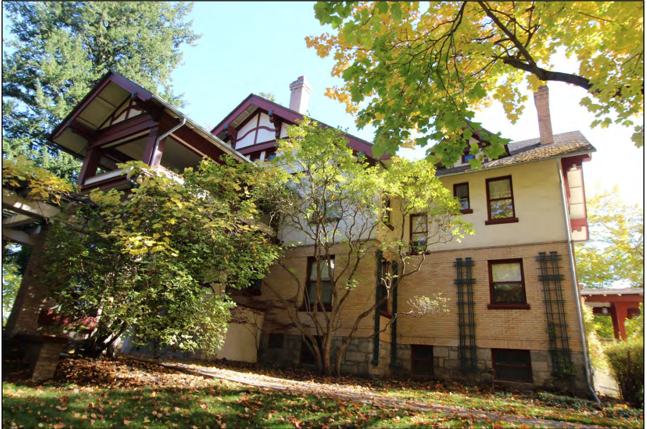
Photo 3 of 21: West side façade, looking east
