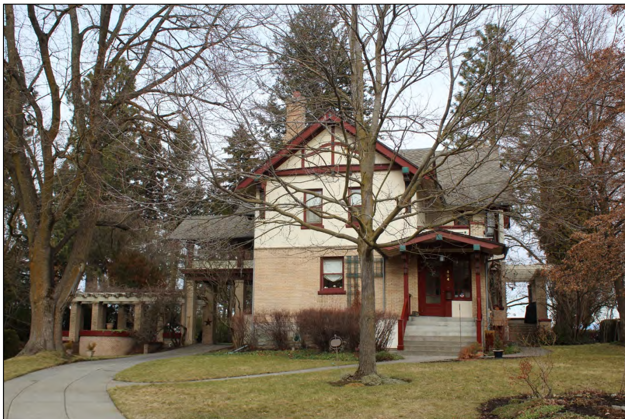
Photo 6 of 21: Rear (south) façade, looking north
