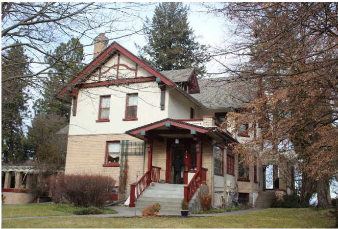
5 Southeast elevation from Sumner
