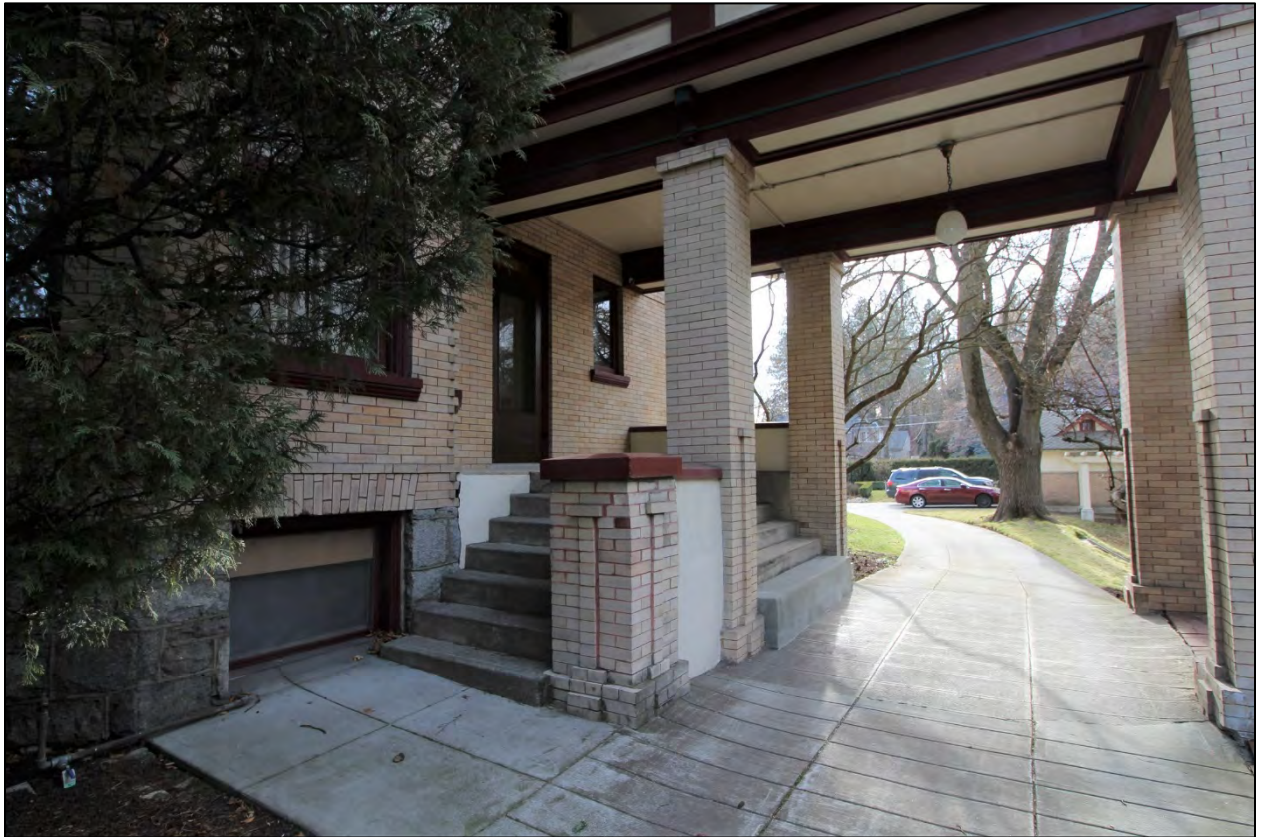
Photo 4 of 21: West side façade, porte cochere, looking south
