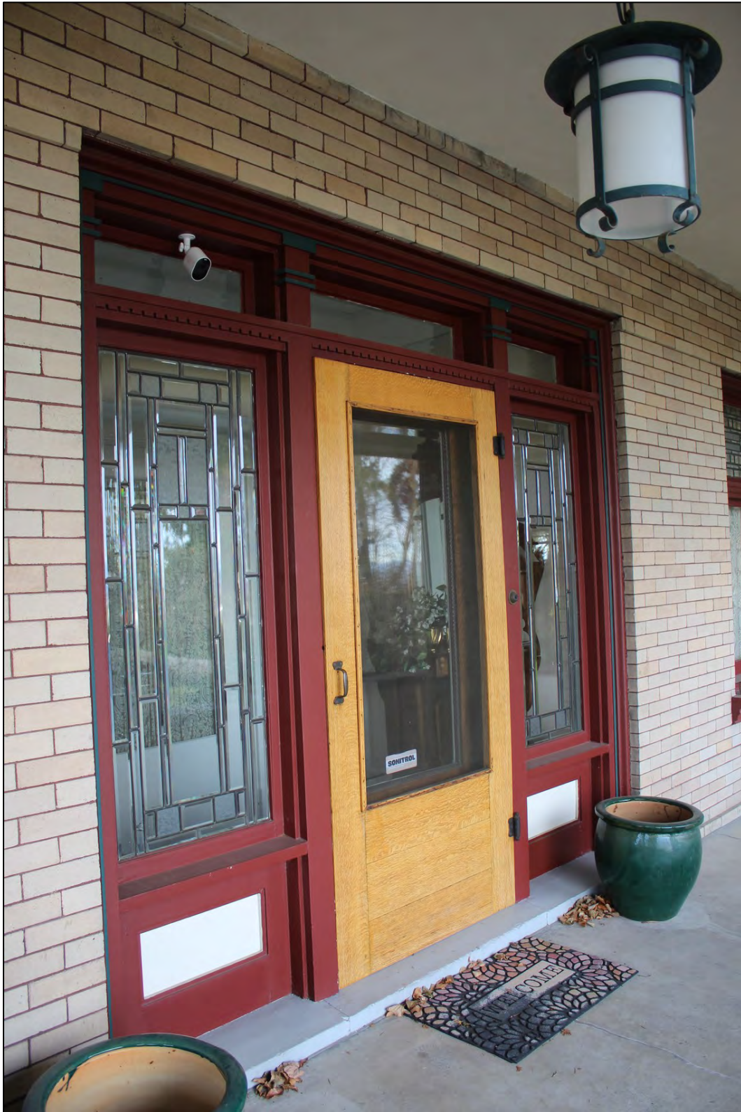
Photo 2 of 21: Front entry detail
