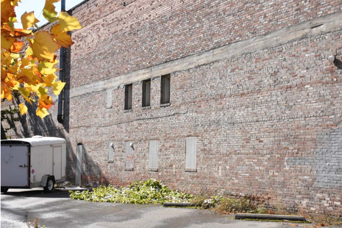
11. East facade - midsection, looking southwest
