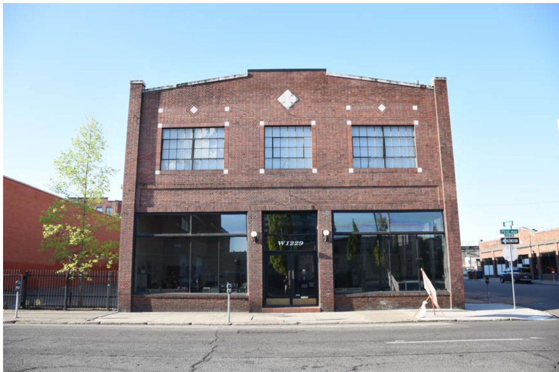
4. Front Façade – 1229 First Avenue – looking south
