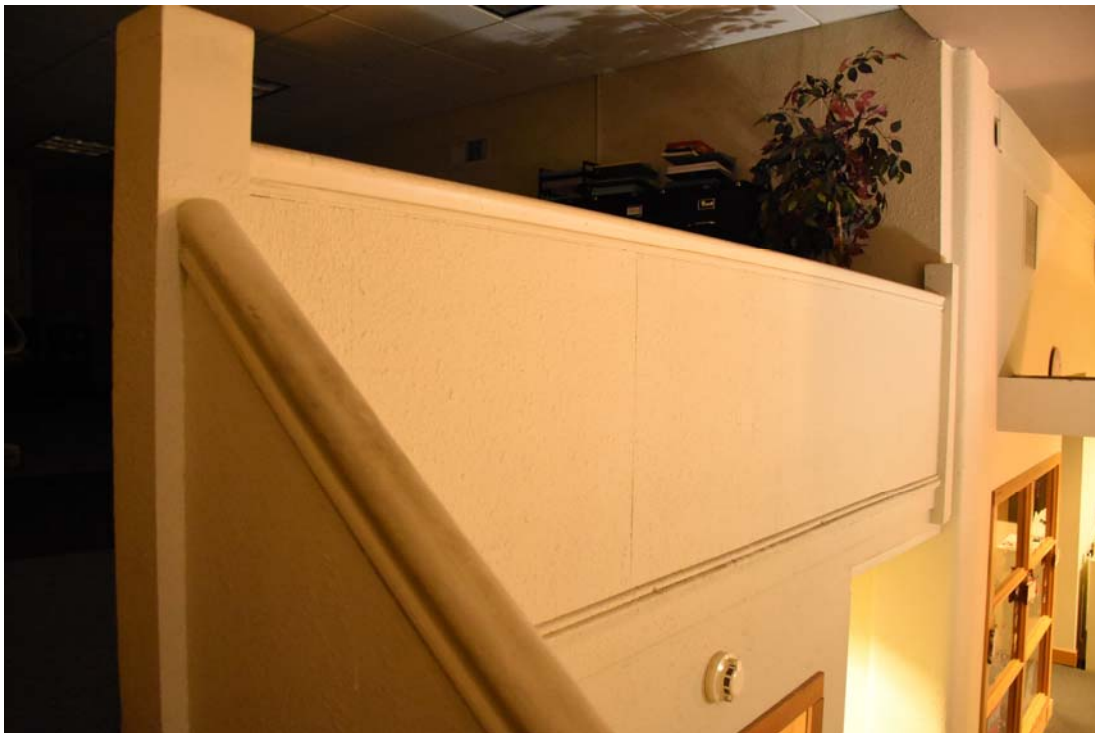
8. Mezzanine, looking west from stairway
