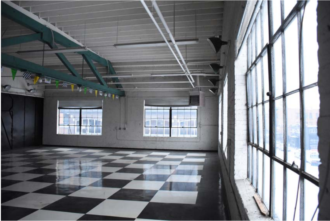
17. Second Floor, looking west along north wall
