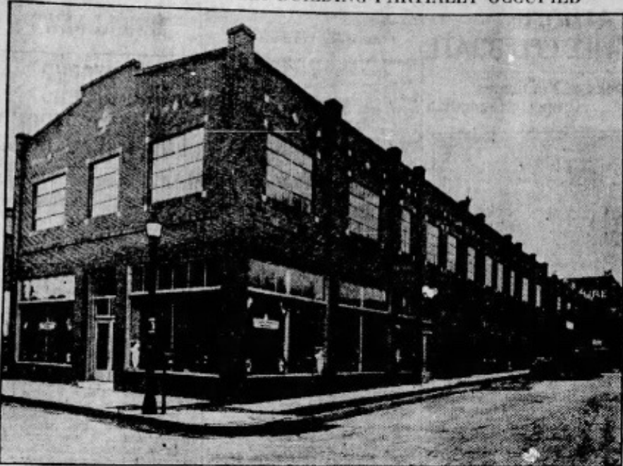
The partially completed Wells-Chevrolet building, First and Adams, is already being used for display and sales of new and used cars.
