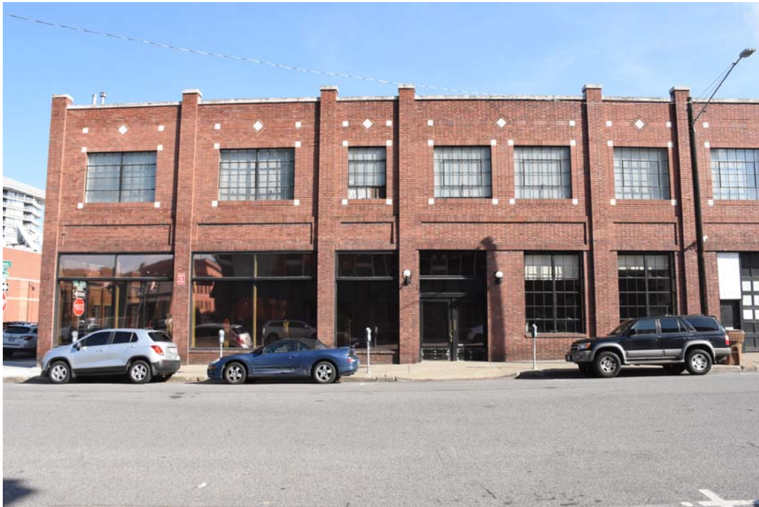
6. North end of west facade, looking east
