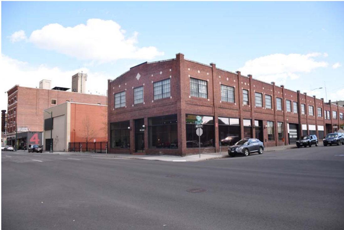
1. First Avenue/Adams Street - context, looking southeast
