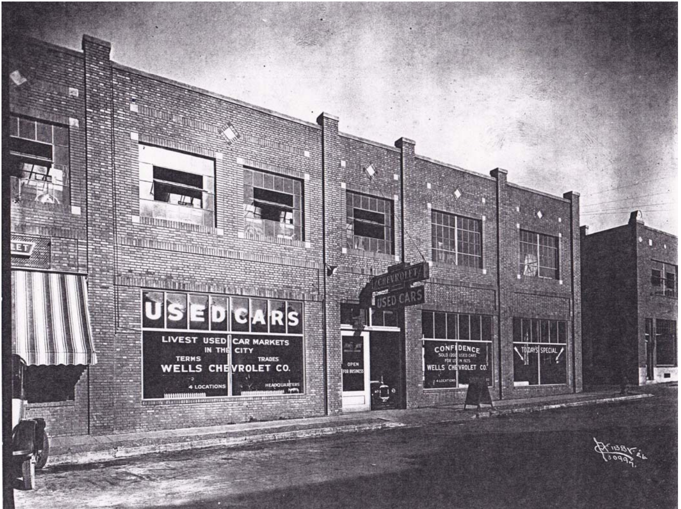
L87-1.30997.26 - Wells original west façade, 1926
