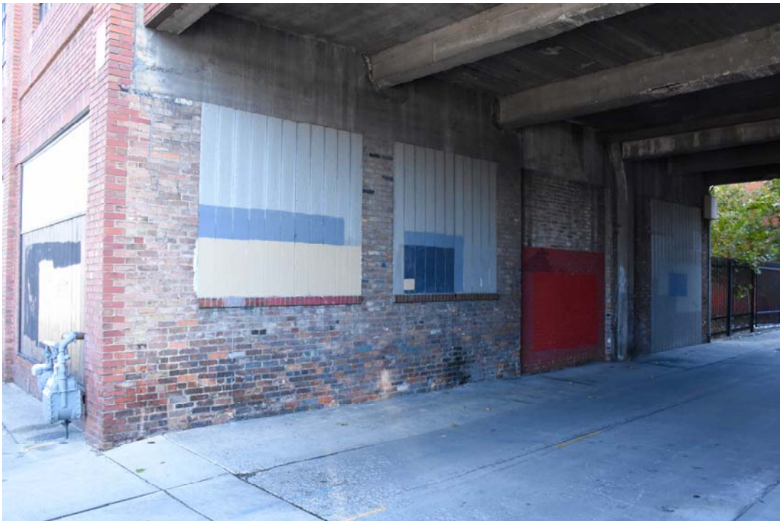
10. South façade along alley, looking northeast (beneath skybridge)
