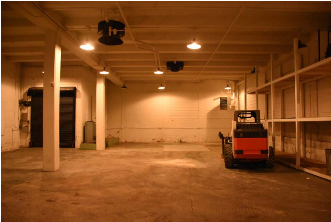
9. Garage Area - south half of building, looking south-freight elevator in southeast corner
