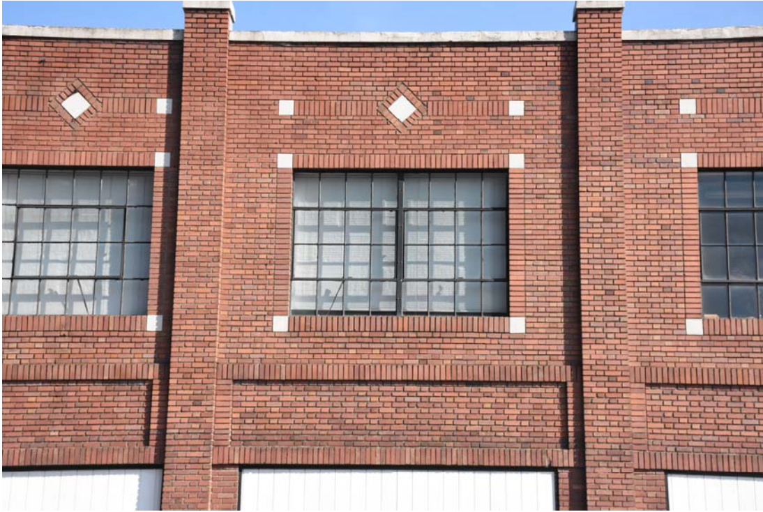
9. West façade second floor window bay detail, looking east
