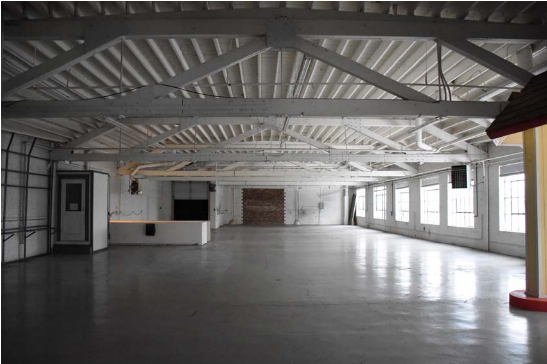
18. Second Floor, Looking South From "Display Room" Partition
