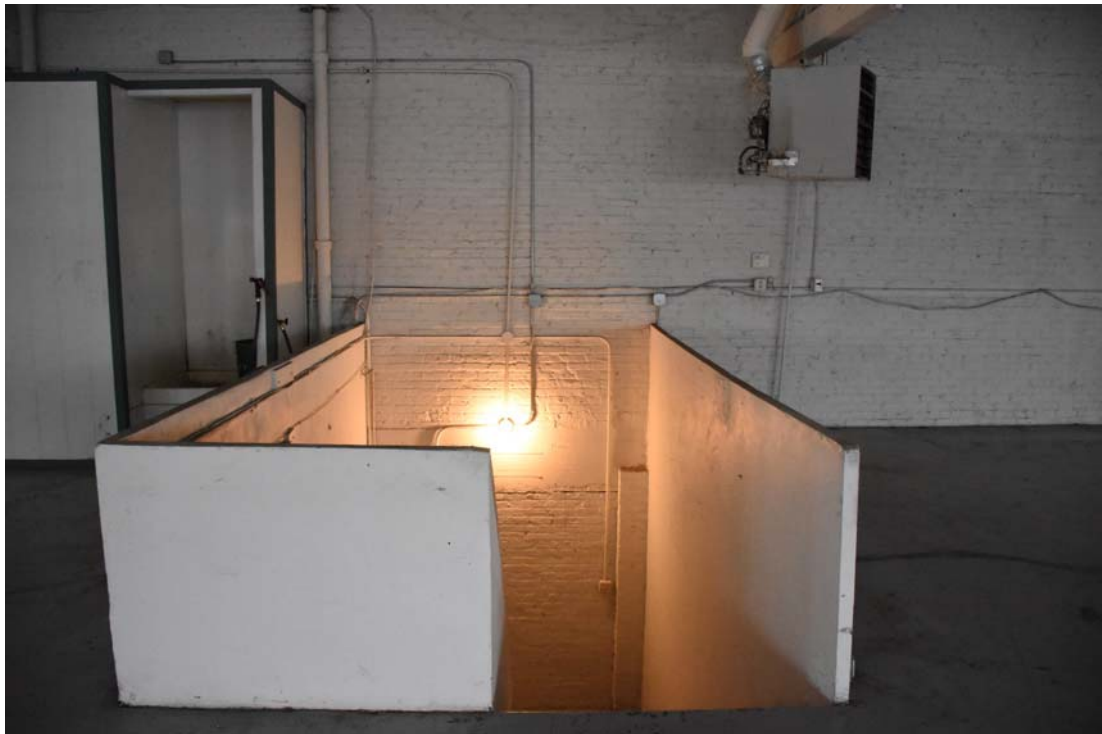
12. Second Floor-stairwell to first floor, looking east
