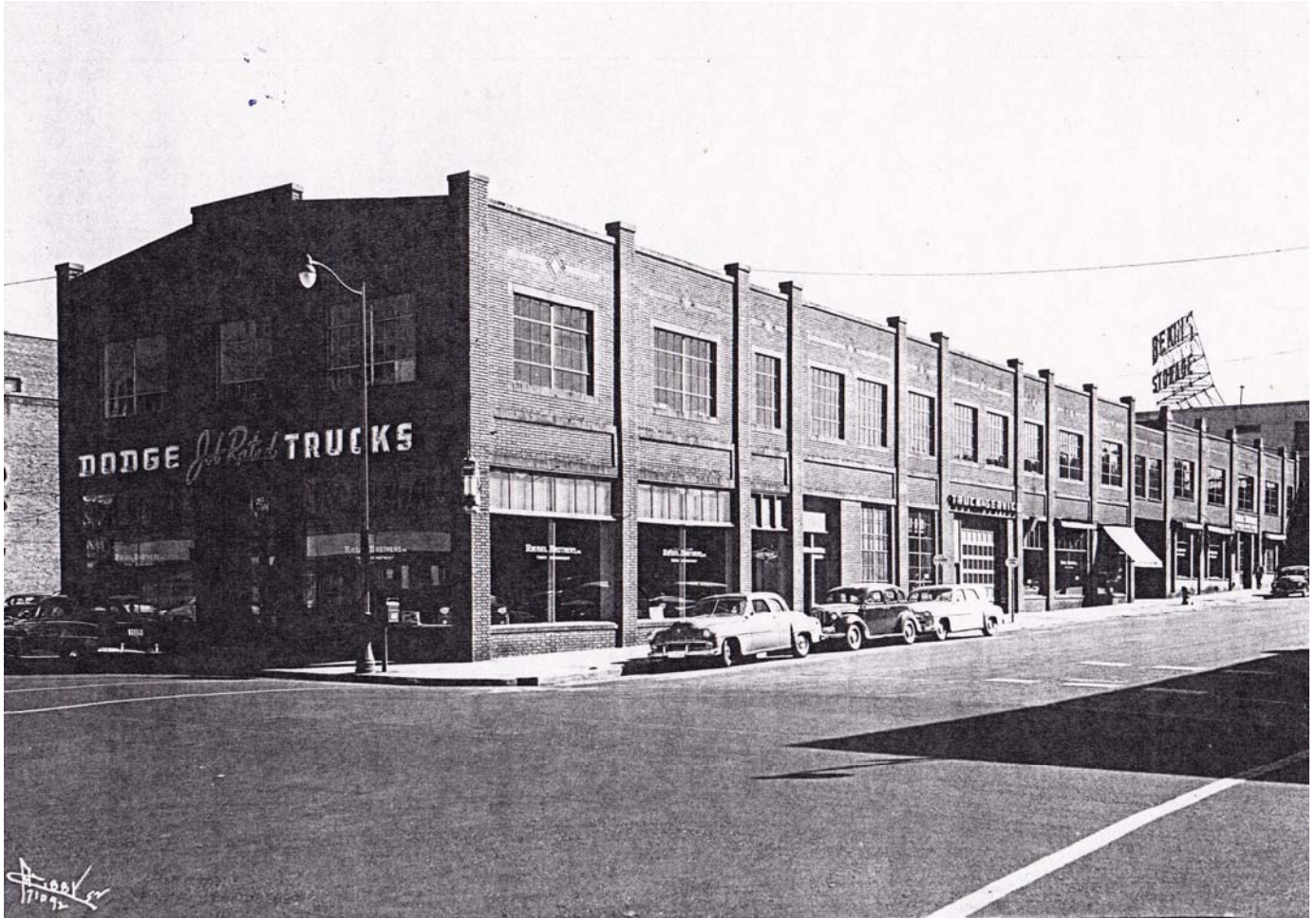
L87-1.71092-52. Riegel Brothers Trucks 1952 (Shows reconfigured Service Entrance in West Façade)
