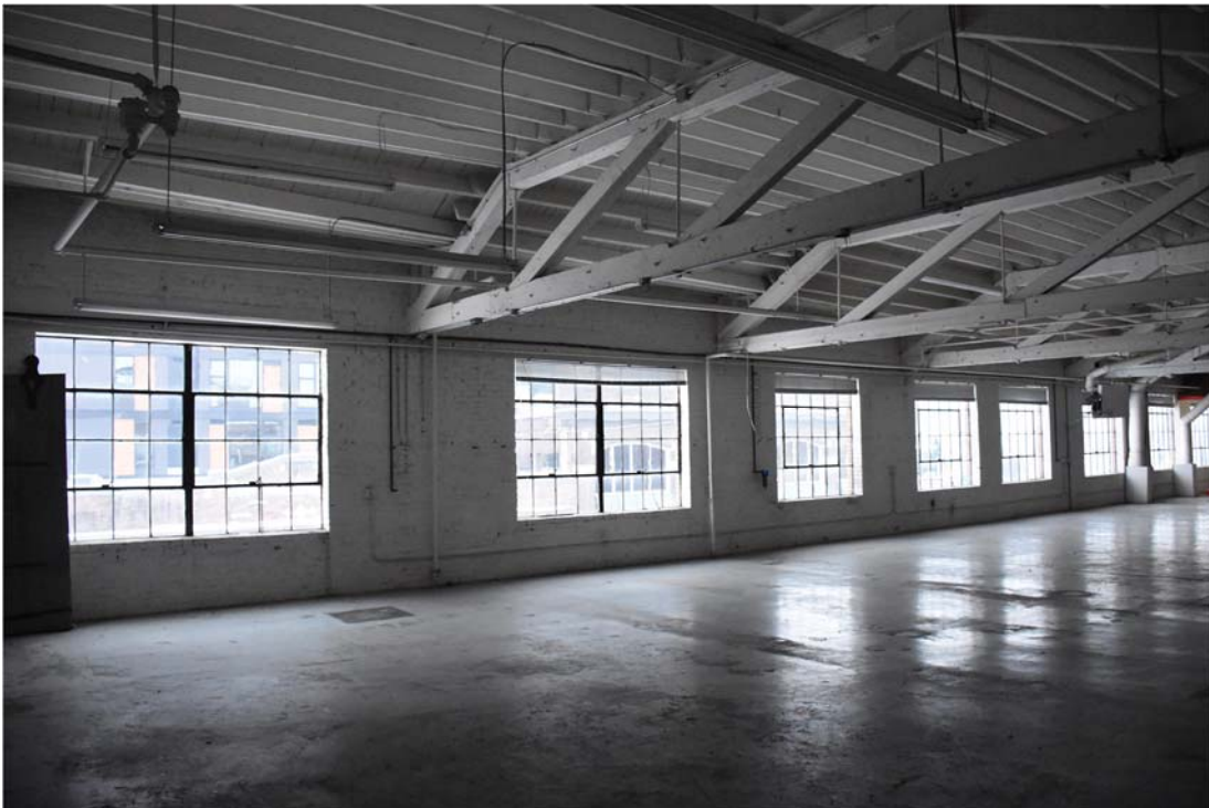
14. Second Floor, looking northwest across shop floor
