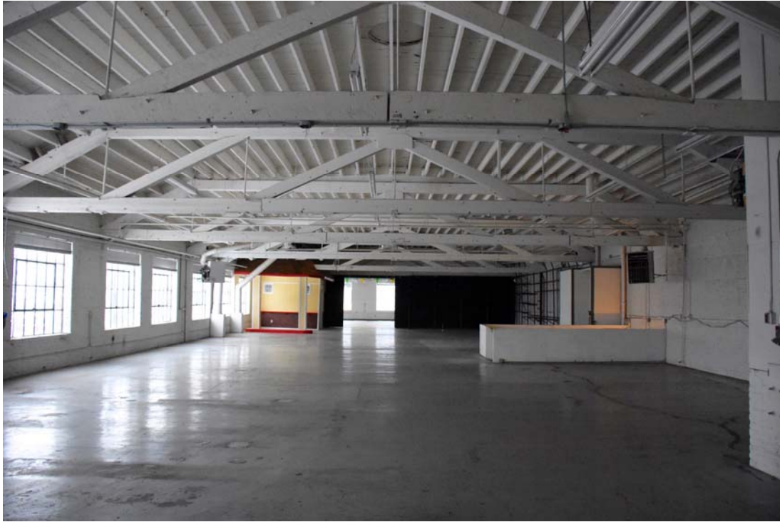
13. Second Floor, looking north from south wall
