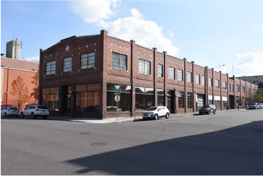
5. Northwest corner – north and west facades, looking southeast
