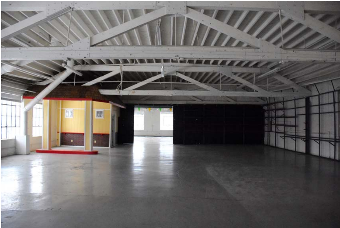
15. Second Floor, looking north toward "display room" partition
