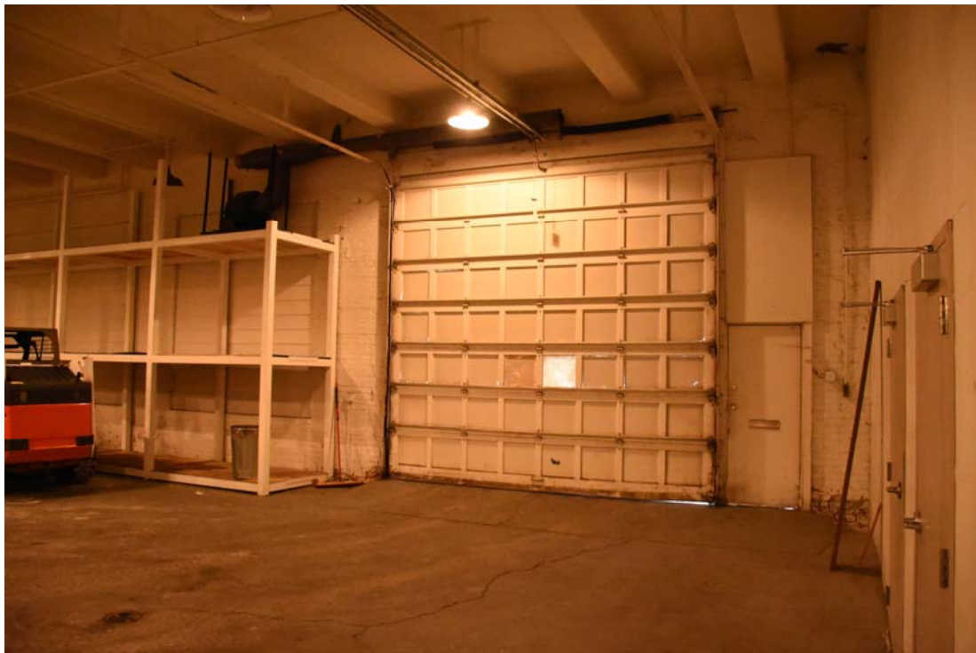
10. Garage Area - looking west toward main entry
