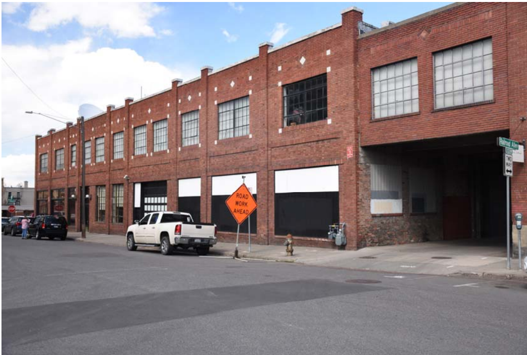
8. Southwest corner – west and alley façades, looking northeast (attached to skybridge of former Wells Chevrolet Service Building)
