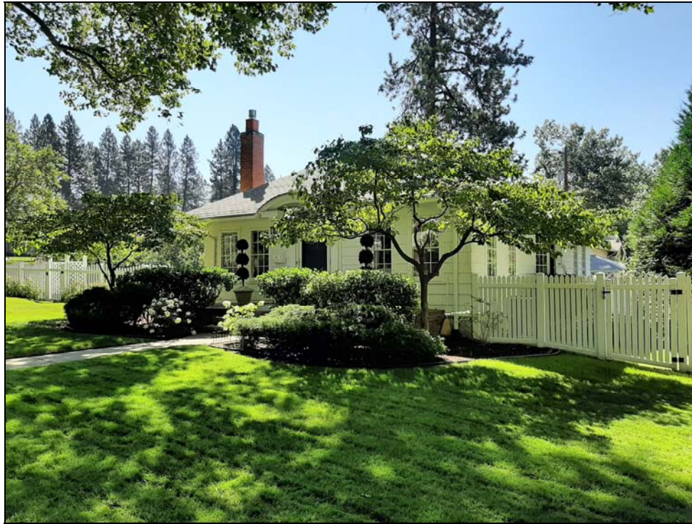
Photo 3—north façade and west side of house in 2020.
