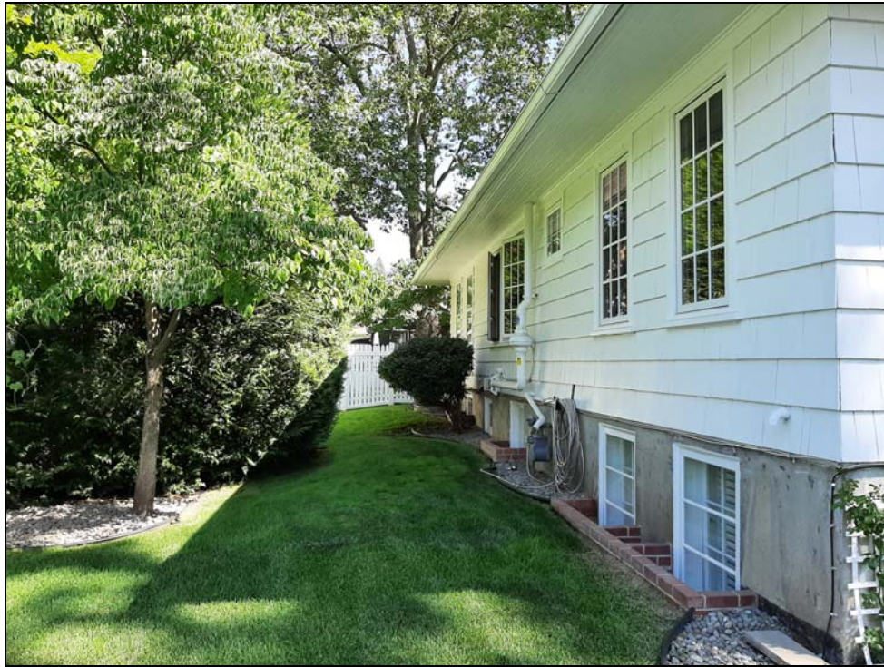
Photo 11—west side of house in 2020, looking north.
