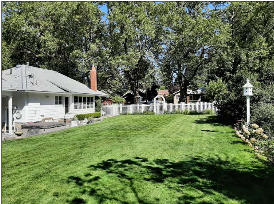
Looking northwest at the east elevation of the Brooke House in 2020.
