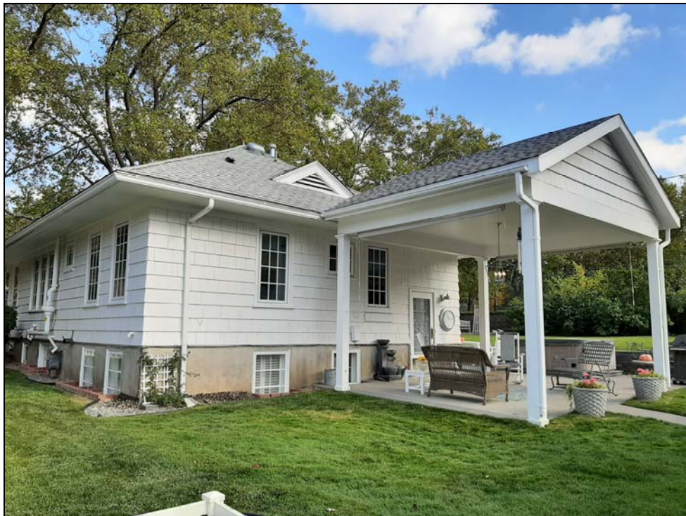
Photo 10—south rear face and covered patio in 2020, looking northeast.
