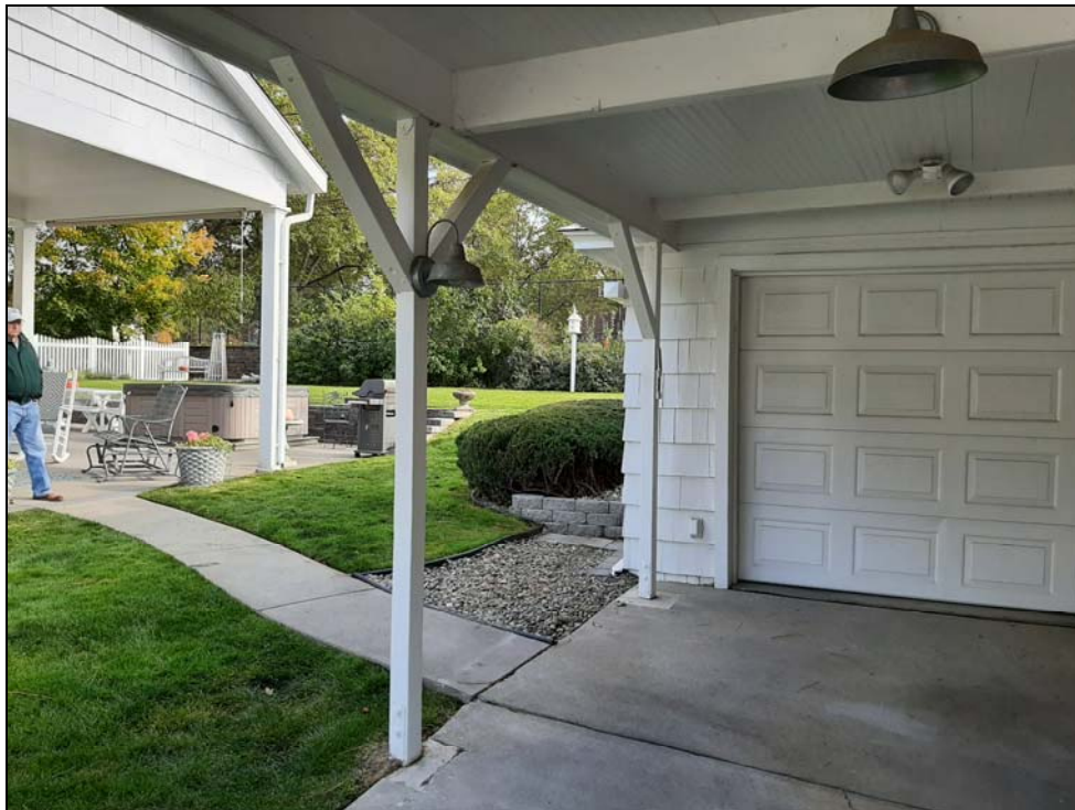
Photo 14—west face of garage door in 2020, looking east.
