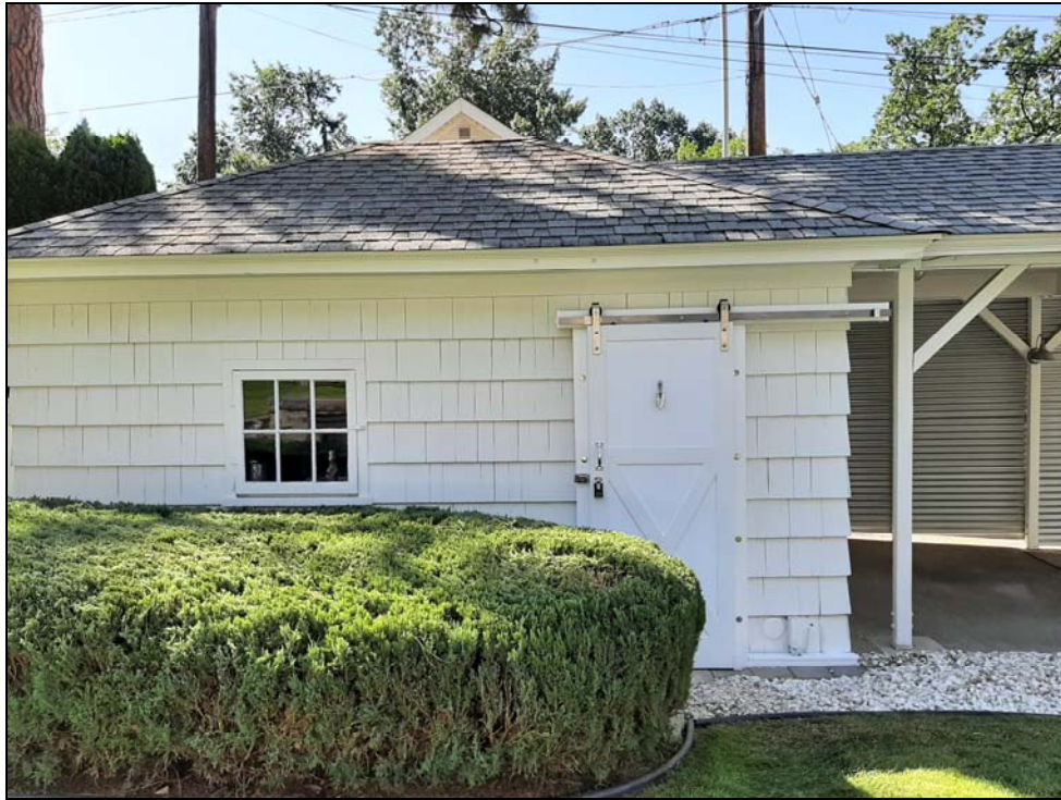
Photo 13—north side of garage in 2020, looking south.
