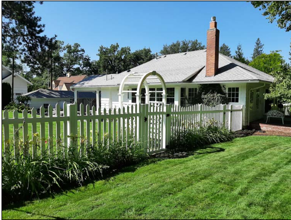
Photo 5—east side of house in 2020, looking west.
