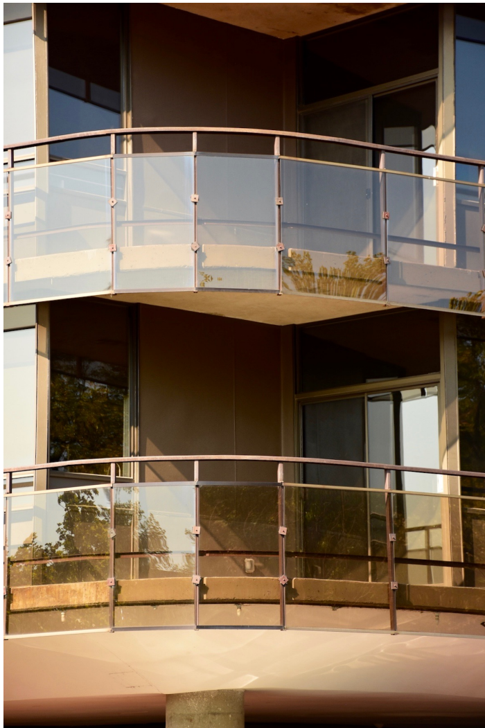
15. Southeast corner balconies, typical
