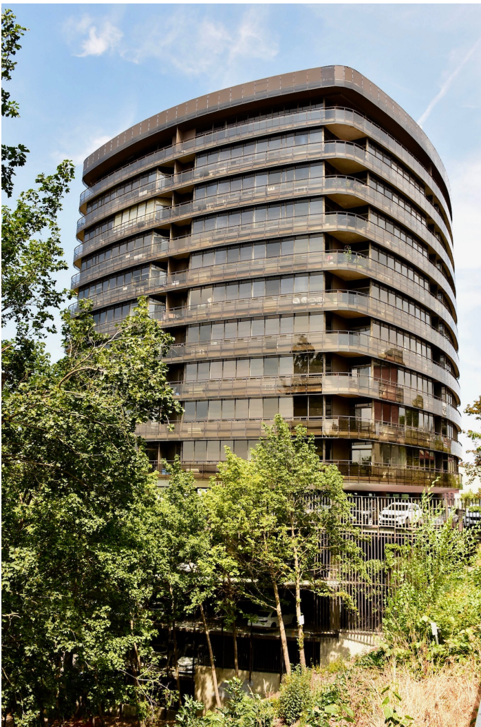
7. West facade - southwest corner, looking northeast
