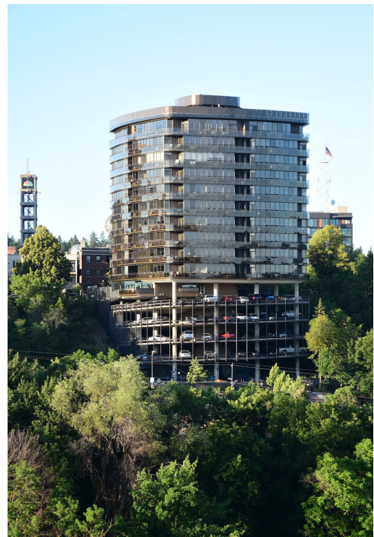
1. Riverfalls Tower as seen from the north looking south
