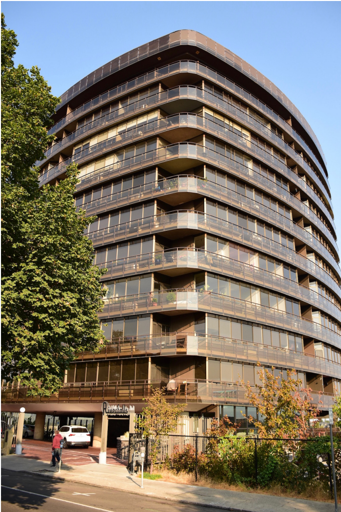
11. Southeast corner - front and east facades, looking northwest
