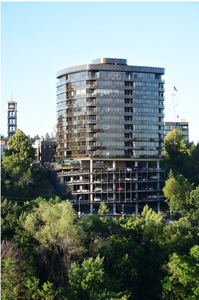
9. Northwest facade, looking southeast
