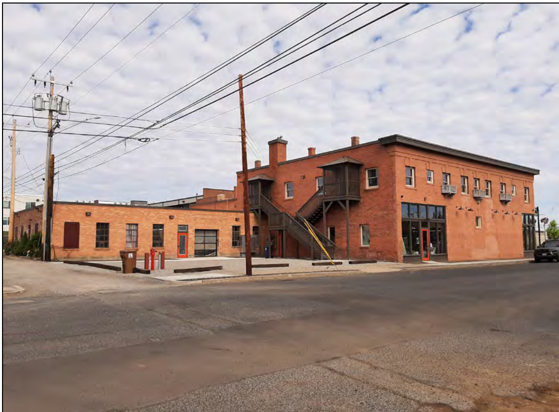
Looking northwest at a 1928 warehouse/shop addition built on the south rear face of the Framingham Building.
