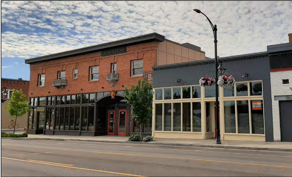
Looking southeast at the north façade of the Framingham Building.
