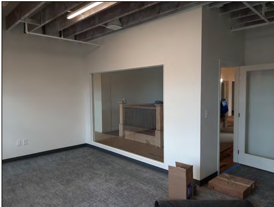
Photo 22 Looking west in 2021 through the above-pictured office on the second floor
