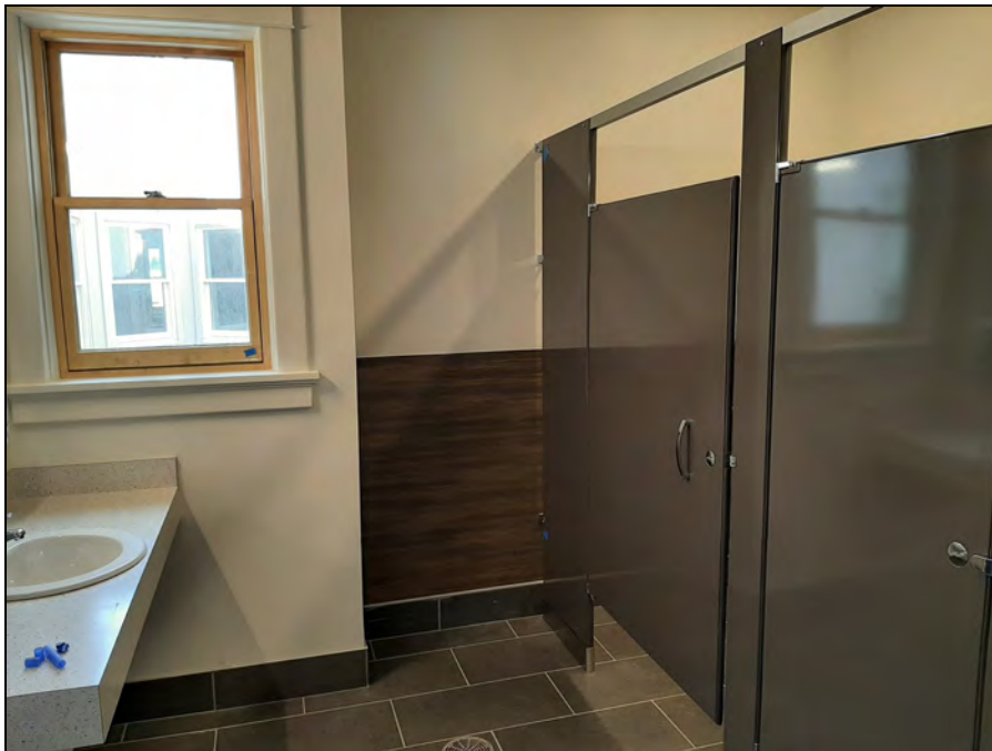
Photo 24 2021 photograph of restroom on second floor, looking west through the lightwell
