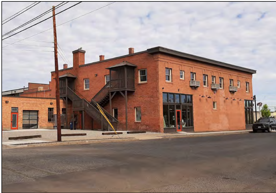
Looking northwest at the south rear face and east face of the Framingham Building.
