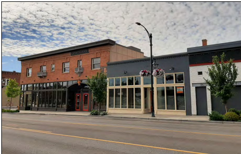
Photo 2 East façade of Framingham Building in 2021—the Framingham Building was built in 1910 as the two-story red brick building with the adjoining west single-story wing
