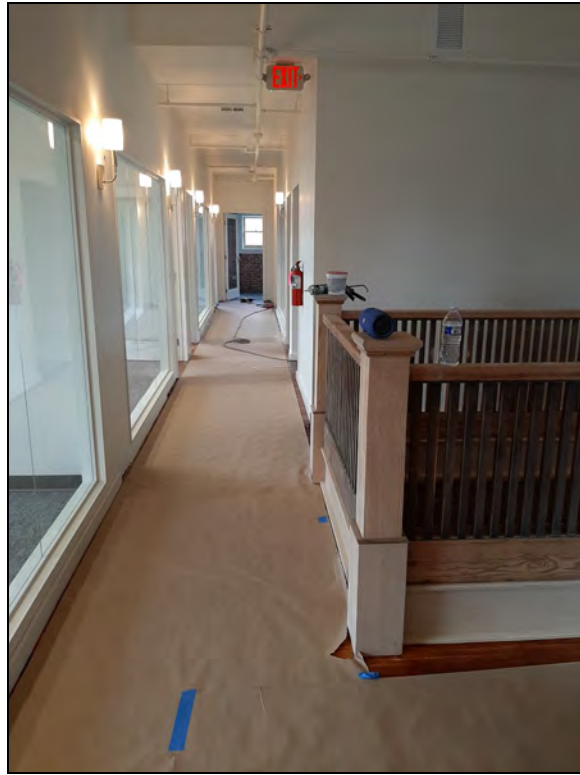
Framingham Building second-floor interior hallway and office “window walls”, looking west.
