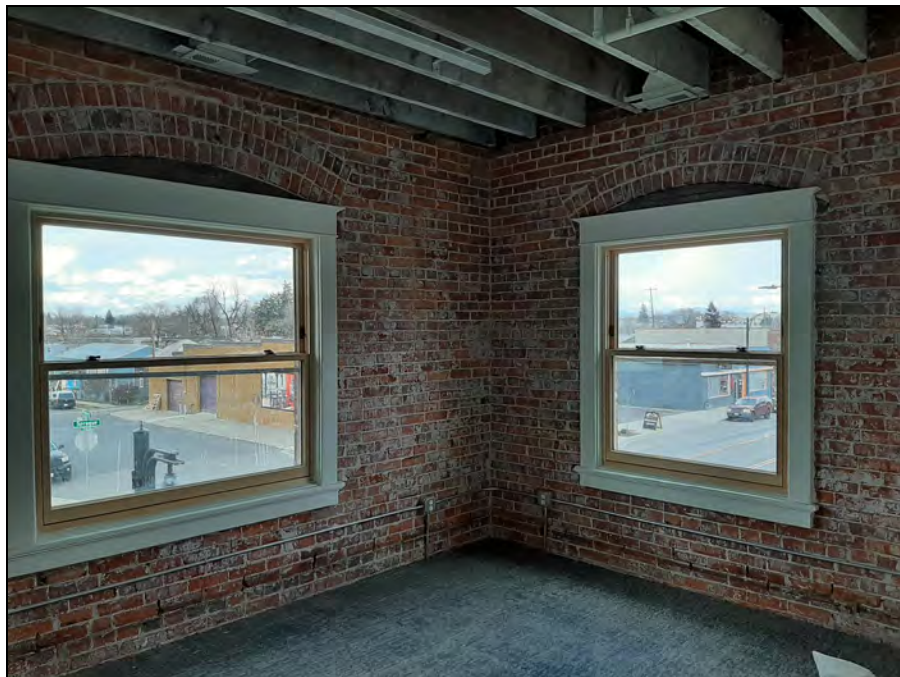
Framingham Building northeast corner room on second floor, looking northeast.
