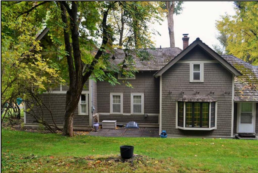
**Figure 11.** Residence, south/rear elevation: ca. 1905 west addition, left, ca. 1885 gable front and wing section, center, ca. 1885-1900 east addition, right. View to the northwest.
