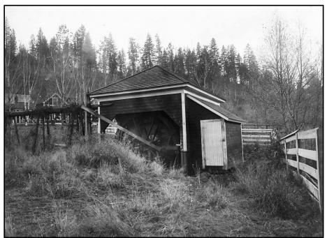
Figure 66. The "Old Mill" that "furnished power before electric service was installed," ca. 1910 (Olmsted Archives 3879-9; Waikiki Farm ca. 1909). Note the boxed eaves, matching construction of the residence's ca. 1895-1900 east addition, and the remodeled residence in the background.
