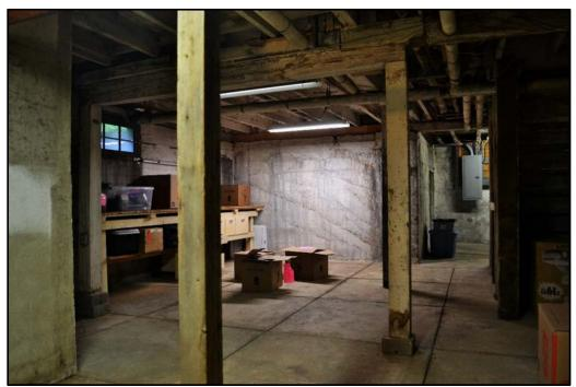
Figure 39. Residence, basement: Cutter & Malmgren Cellar (Rahn Basement); note diagonal banding in the poured concrete wall. View to the southwest.
