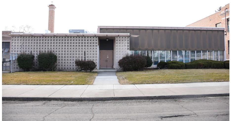
of the glass panel façade wall. The wall is composed of sixteen columns of glass panels divided by steel mullions spaced at 2'-9" on center. Narrower horizontal muntins divide the vertical panels into variable widths from 4 feet to 5 feet. The muntins are staggered and alternate every other vertical division as do the bottom glass panels which are operable. During an energy retrofit in 1986, insulated aluminum panels replaced the upper 10'-6" of the glass panel wall,
