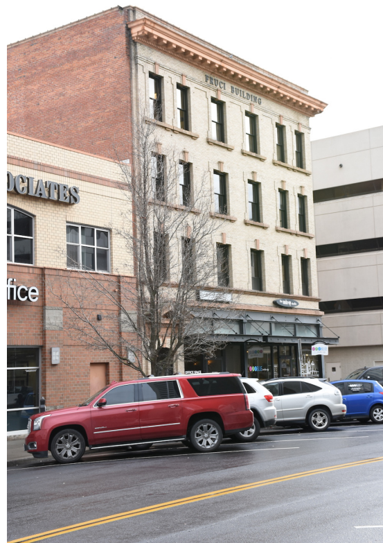
4. Northwest Corner-front and north facades, looking southeast
