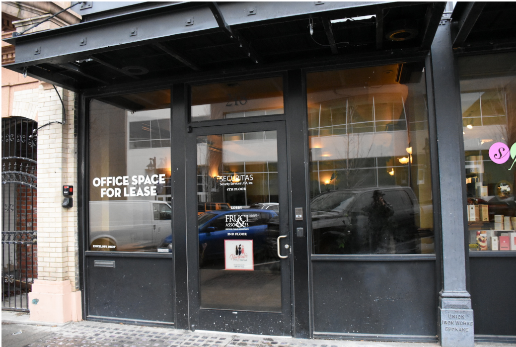
13. Storefront on north side, looking east
