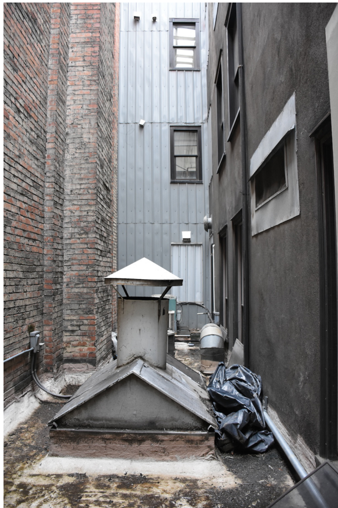
40. 2nd Floor-looking east at lightwell
