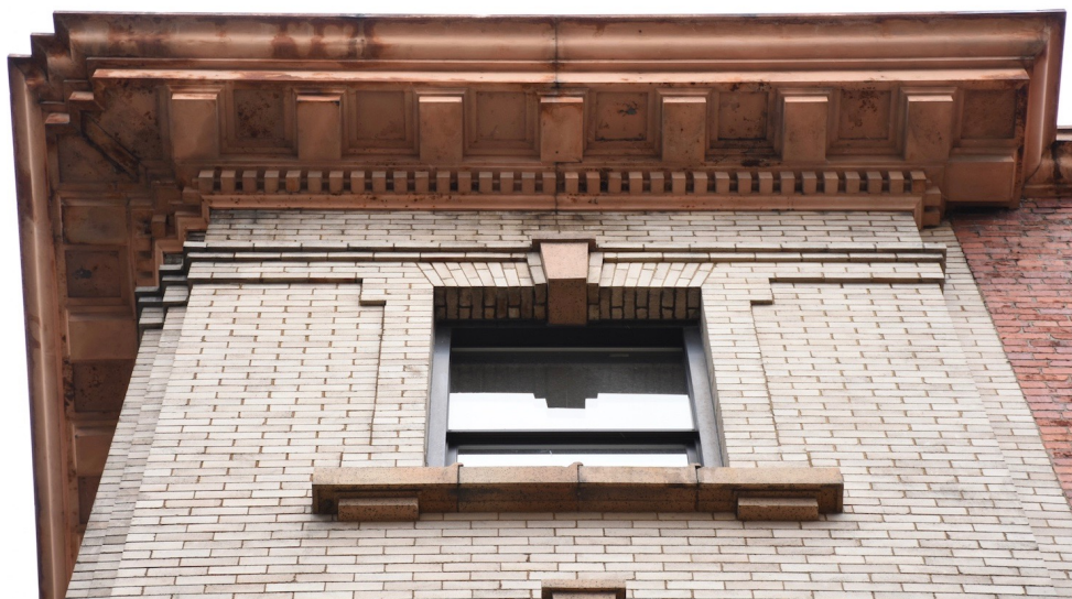
16. Southwest corner, south side window, cornice, looking north, looking northeast
