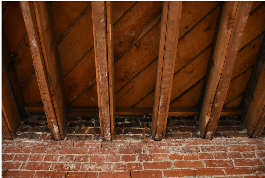
32. 3rd Floor- looking north at floor joints, typical
