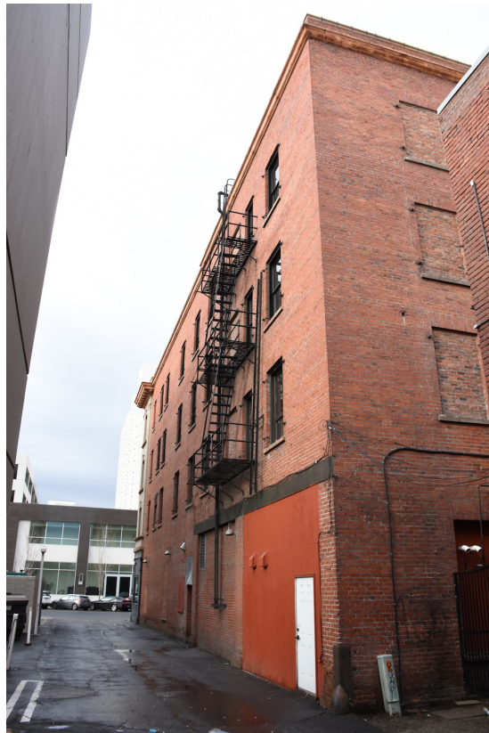
6. Southeast Corner-east façade, looking west along alley
