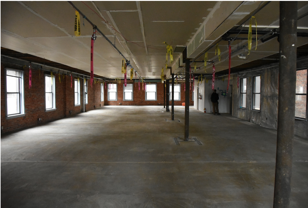
29. 3rd Floor-looking west toward lightwell and stairwell
