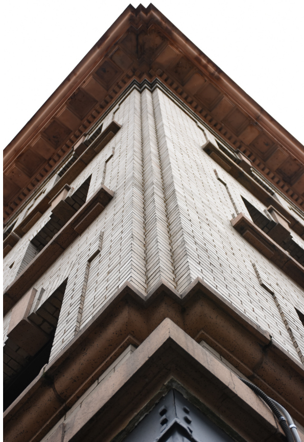
15. Southwest corner details, looking up northeast
