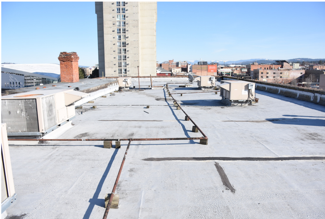
18. Roof, looking east from west end
