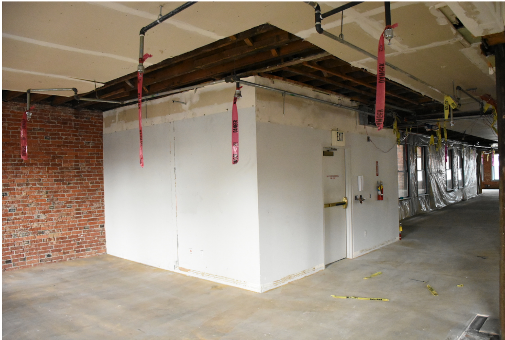
31. 3rd Floor-looking northeast and stairwell
