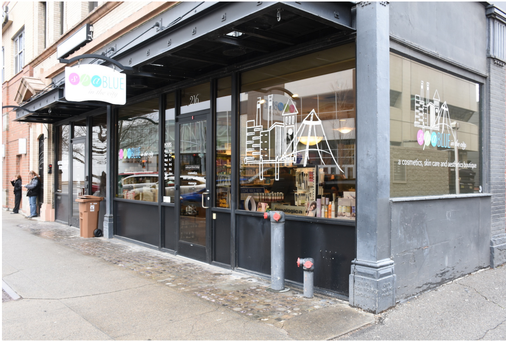
11. Front Facade Storefront and sidewalk vault lights, looking northeast
