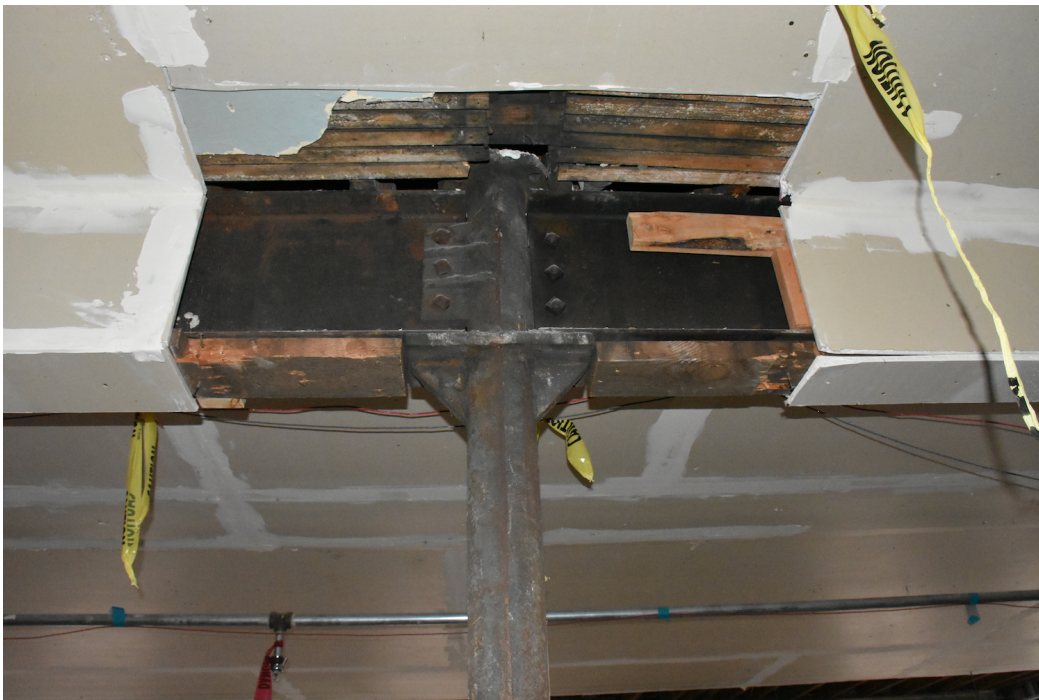
26. 2nd Floor-Steel post and beam along center axis, looking north
