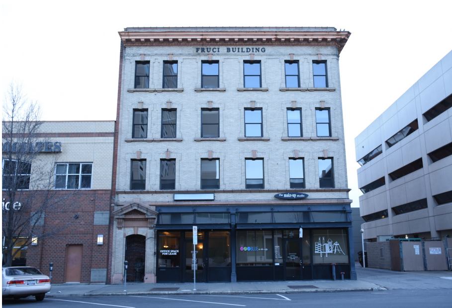
3. Front Facade, looking east
