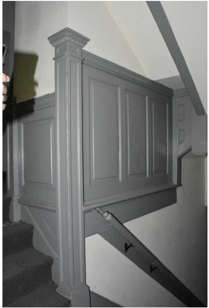
36. Historic stairs- 2nd floor landing, looking southwest
