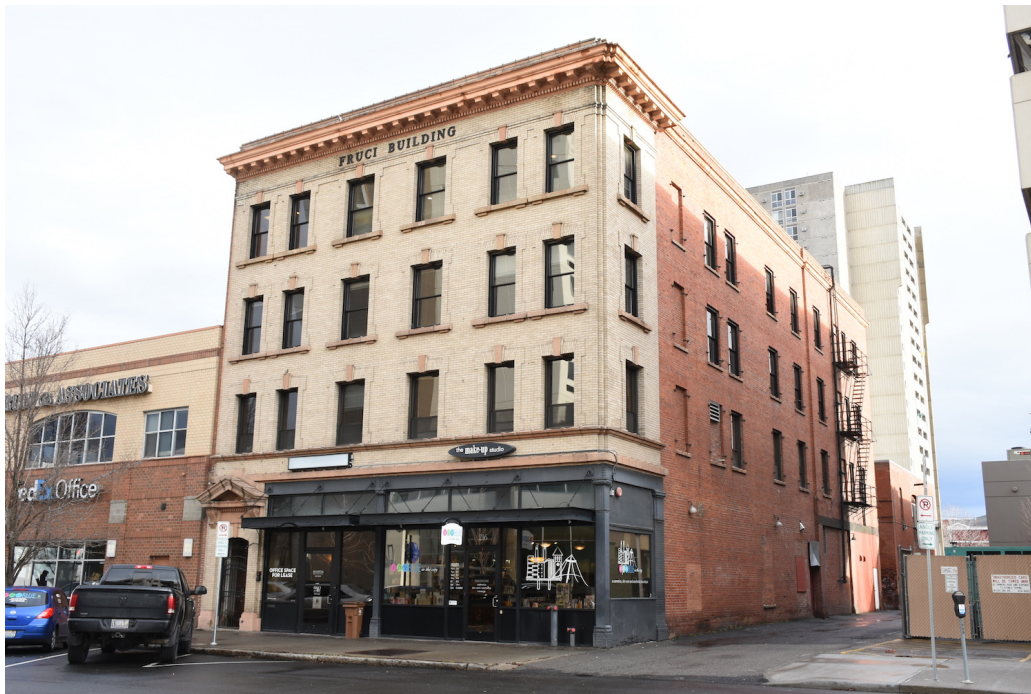
2. Southwest corner of Building-west and south facades, looking northeast
