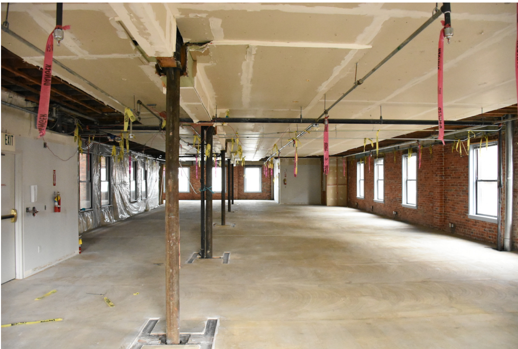
30. 3rd Floor-looking east toward stairwell from west end
