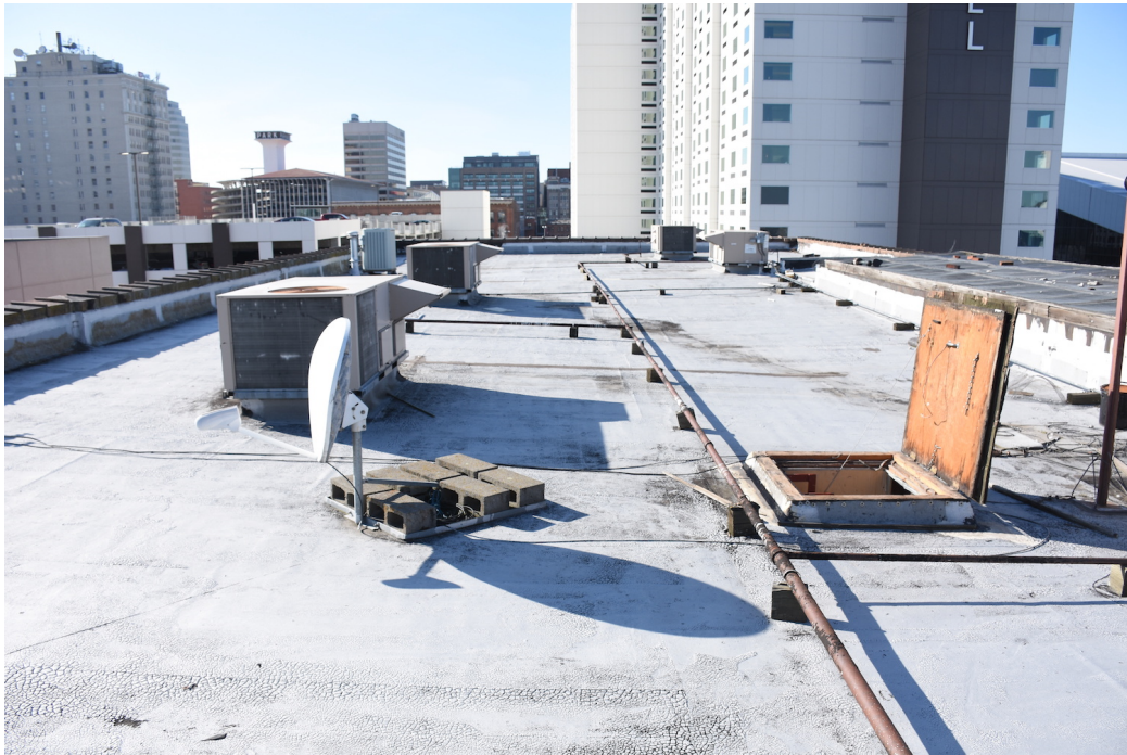
17. Roof, looking west from east end
