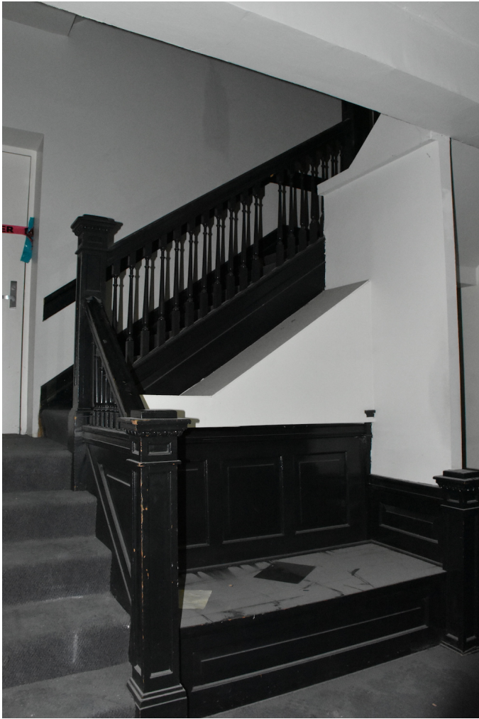
35. Historic stairs and bench on 2nd floor landing.
