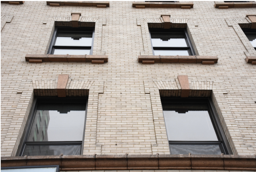
14. Front Facade, window details, looking east
