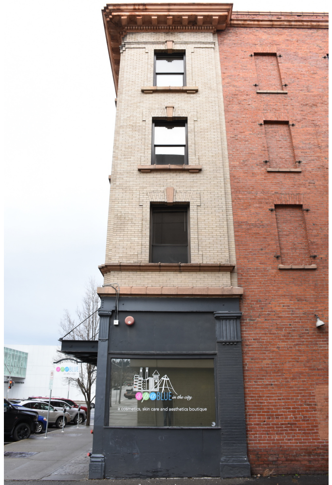
8. South Facade-Southwest corner detail showing cornice
