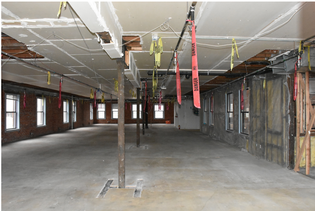
28. 2nd Floor-looking west from rear to front-lightwell to north
