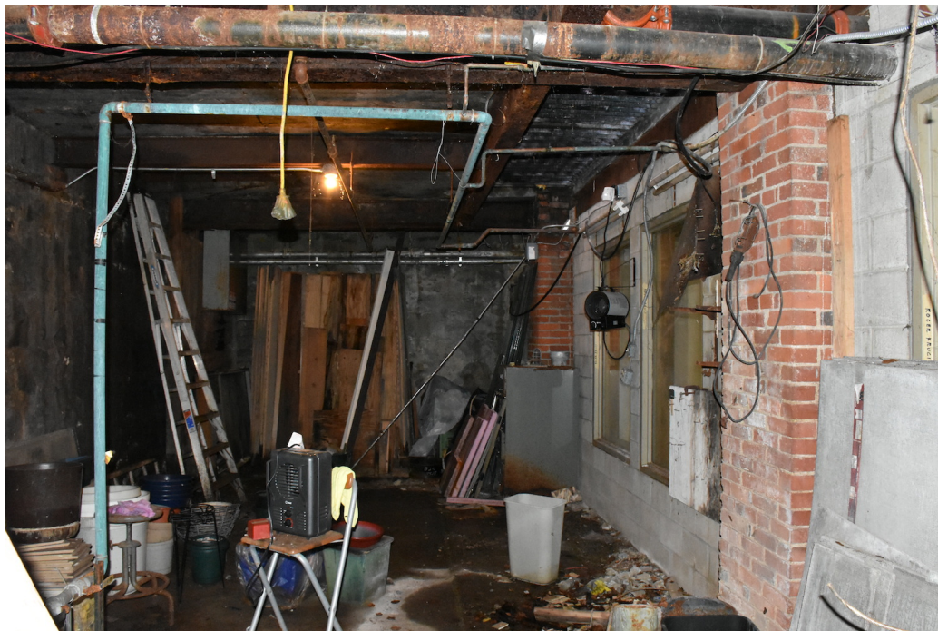
24. Basement-sidewalk vault, looking south
