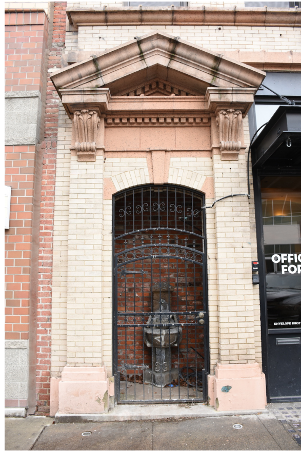
9. Front Facade- former SRO hotel entrance, looking east
