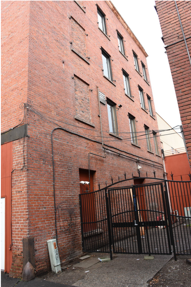
7. Rear (east) facade, looking north return and windows, looking north
