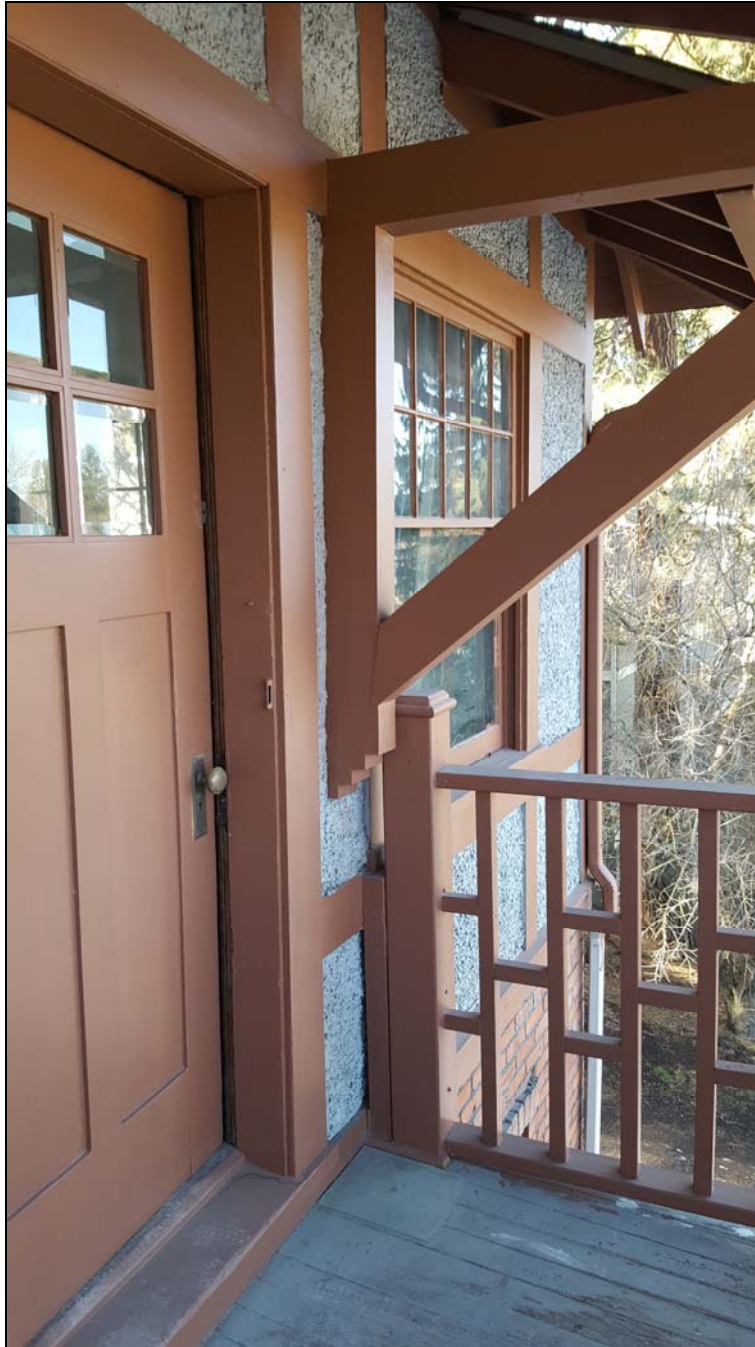
Photo 5—second floor, northwest corner of north façade in 2020
