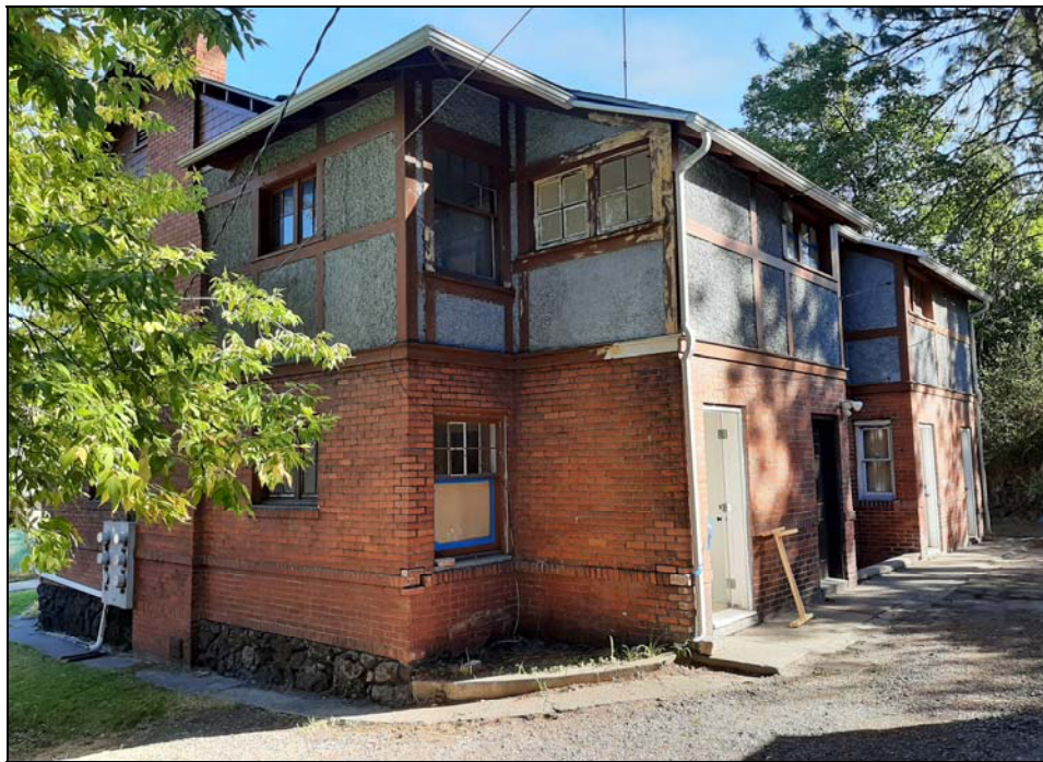
Photo 4—rear face and west end elevation in 2020
