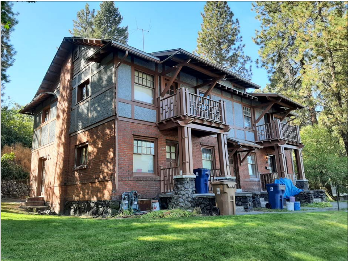
North façade and east end of the Mary Frances Apartments in 2020
