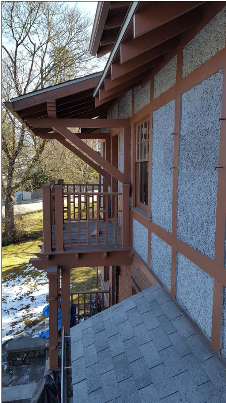
Photo 7—north façade, looking down from second floor in 2020
