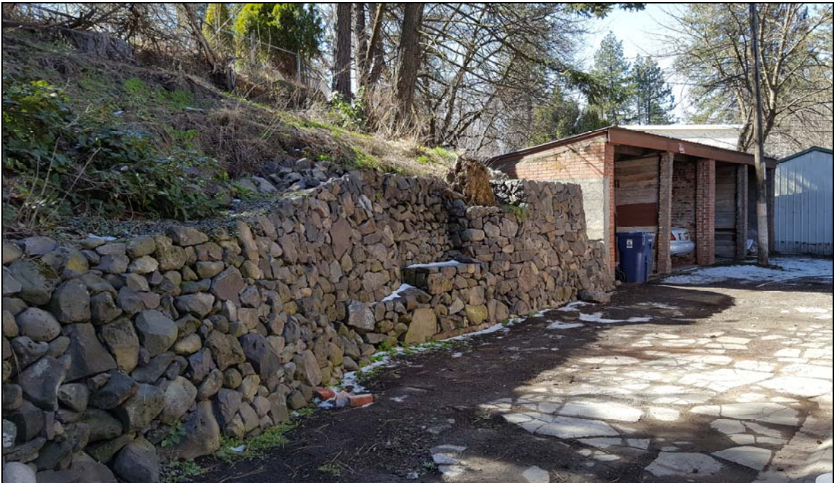
Rear property retaining wall and garages
