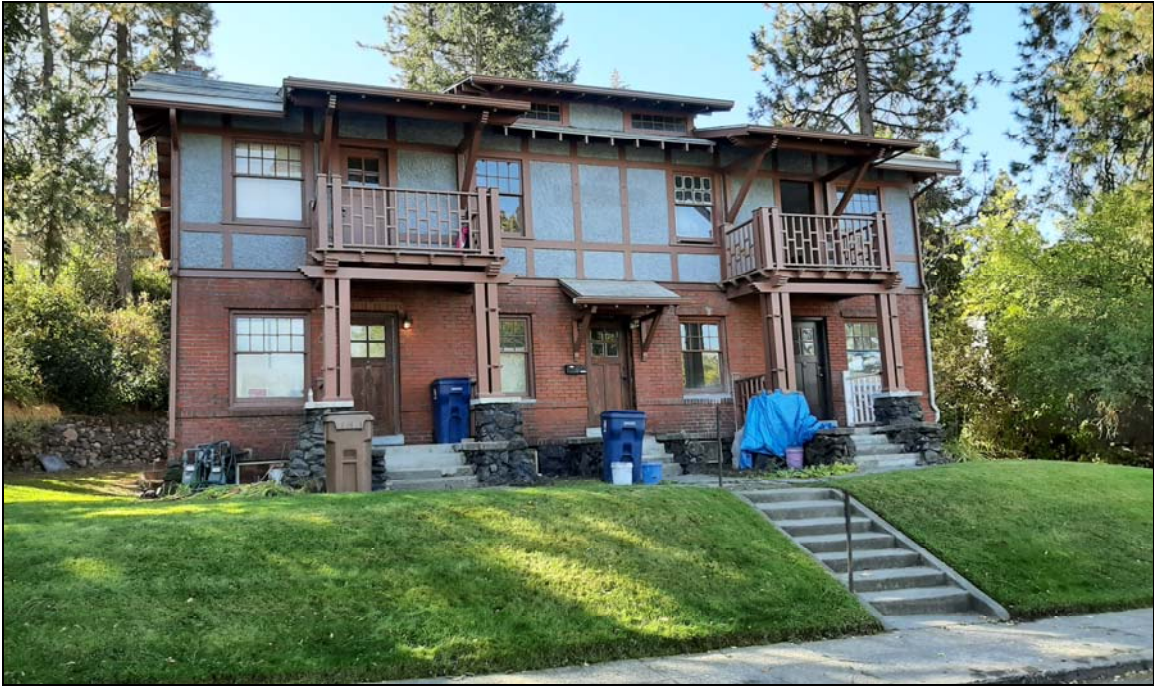
Photo 1—North façade pictured in 2020
