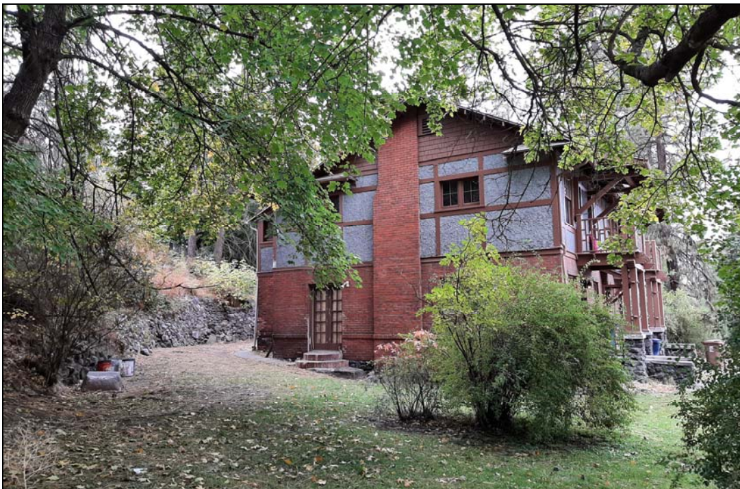
A 2020 photo of the east end of the apartment building and the basalt retaining wall behind the building
