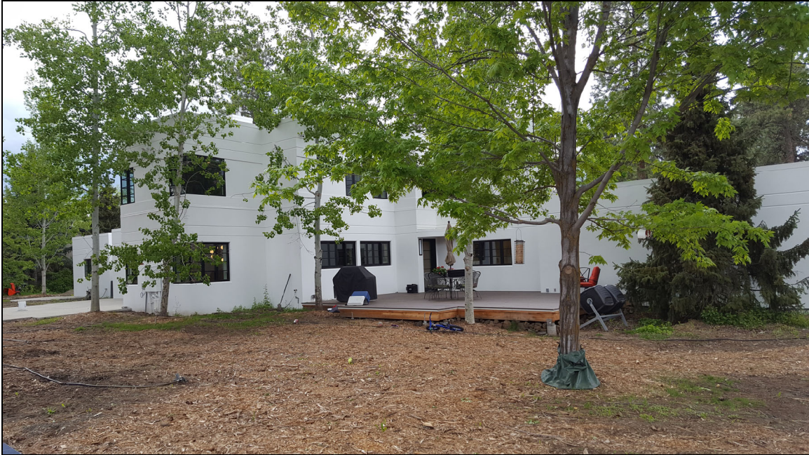
Photo 7: View of rear southeast corner of Thompson House in 2020, looking northwest
