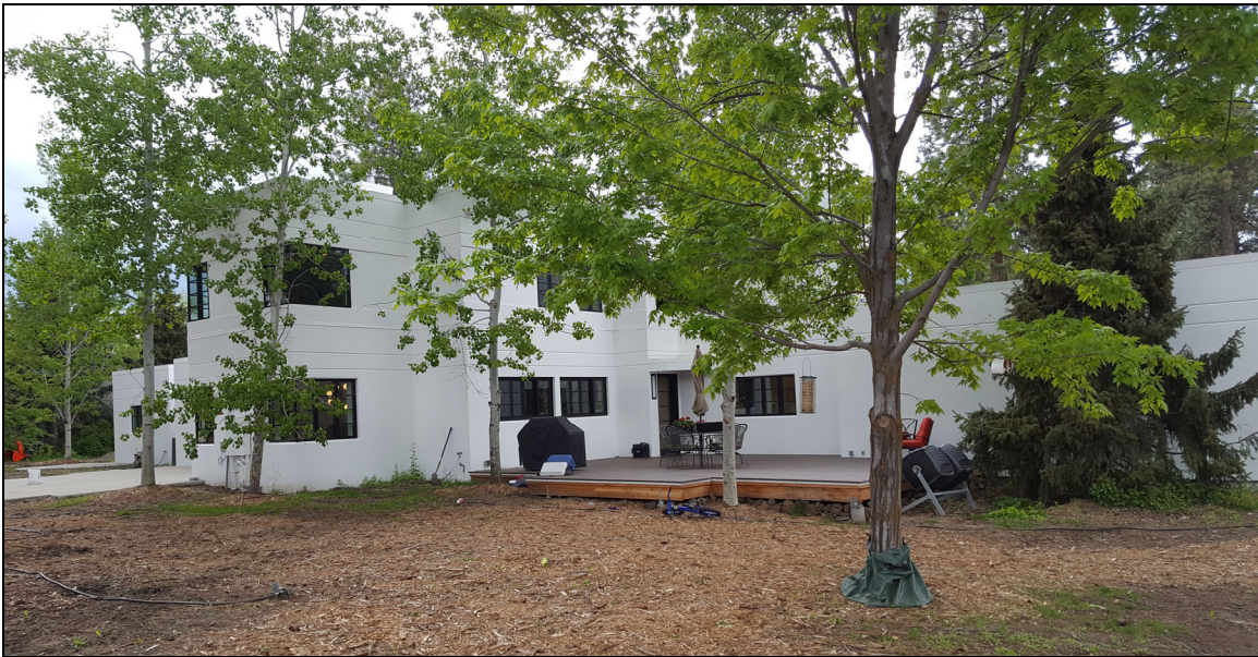
2020 photo of the southeast corner of the Thompson House
