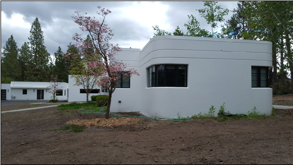
Photo 3: West face of Thompson House in 2020, looking east
