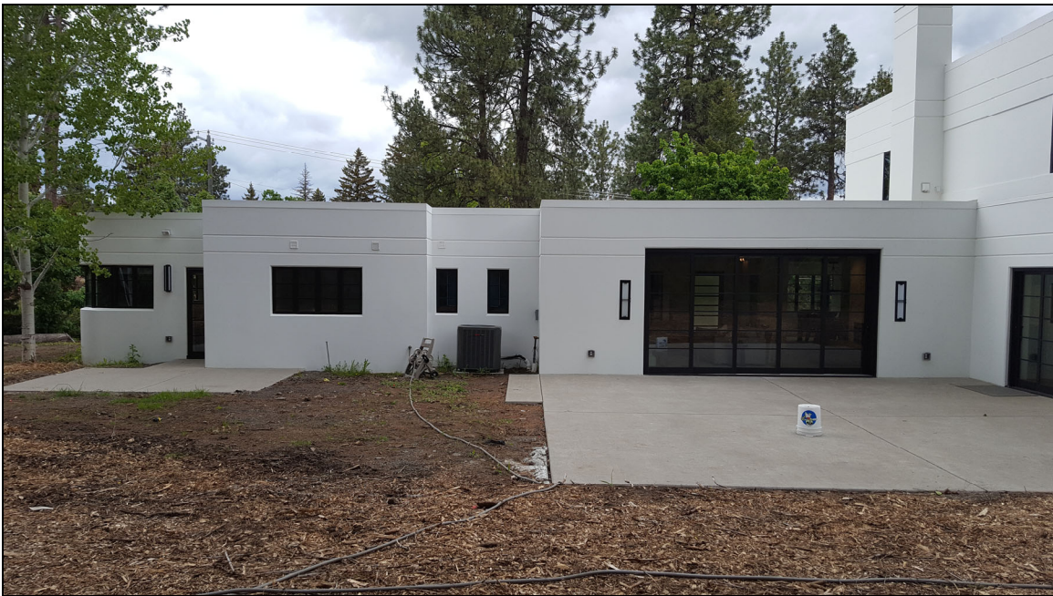
Photos 5 and 6: View of south rear elevation of Thompson House in 2020, looking northeast in Photo 5 and looking north in Photo 6
