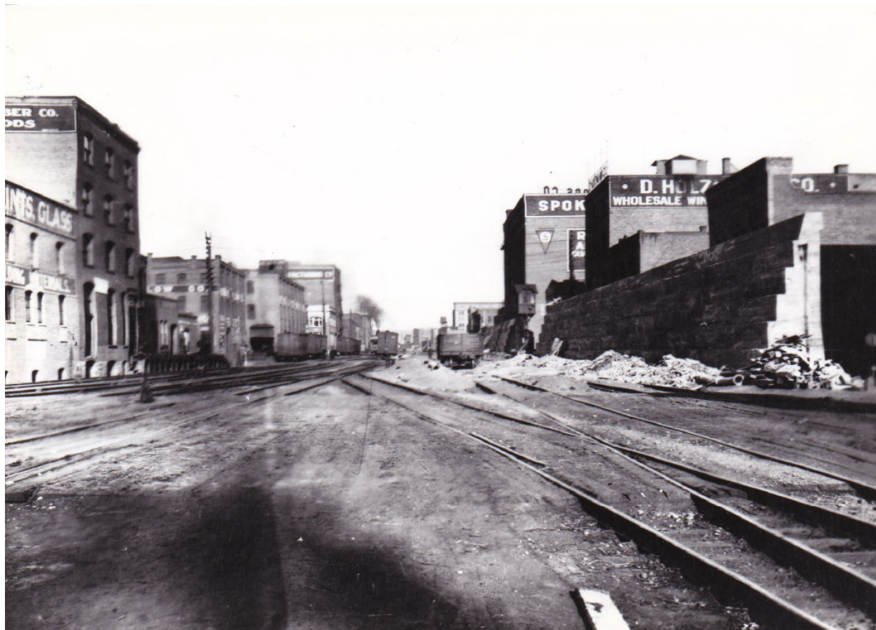
NPRR Tracks, Viaduct Under Construction Looking East from Madison, ca. 1916 North of Tracks: Spokane Paint & Oil, Washington Rubber, Washington Machinery
