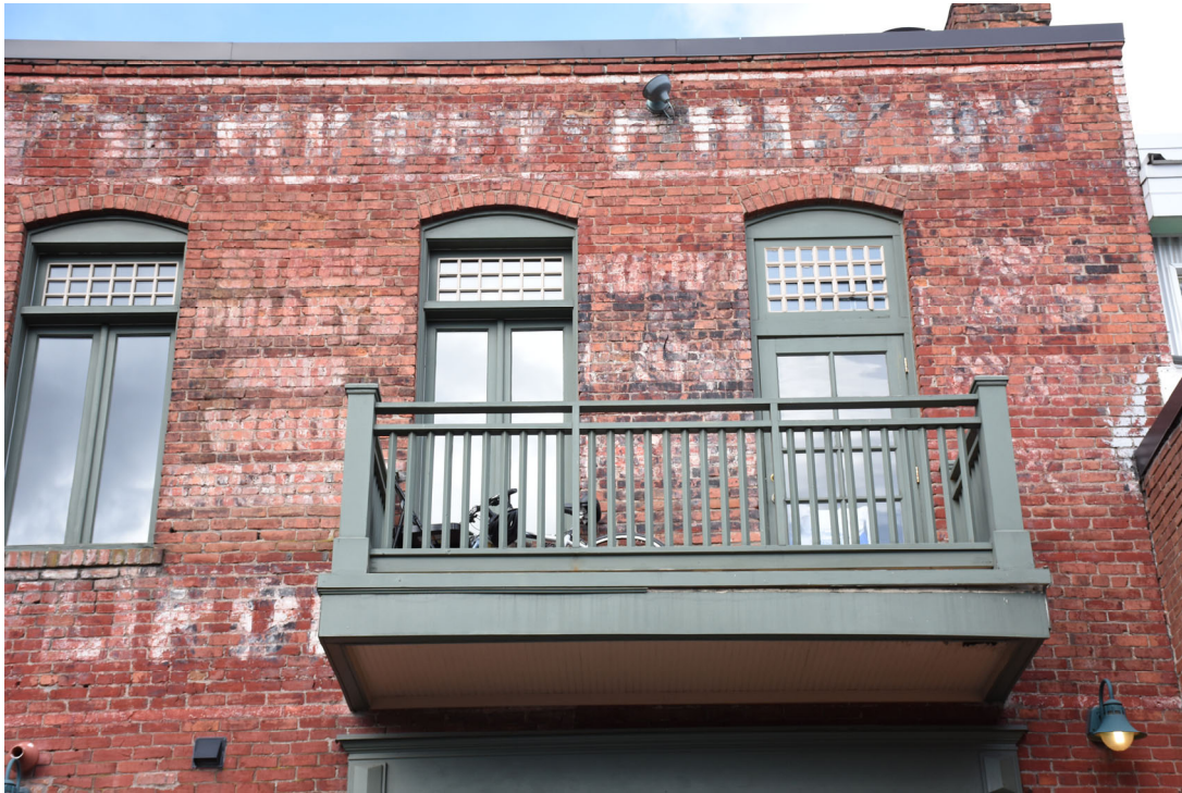
11.South facade-second floor, door, windows, and balcony
