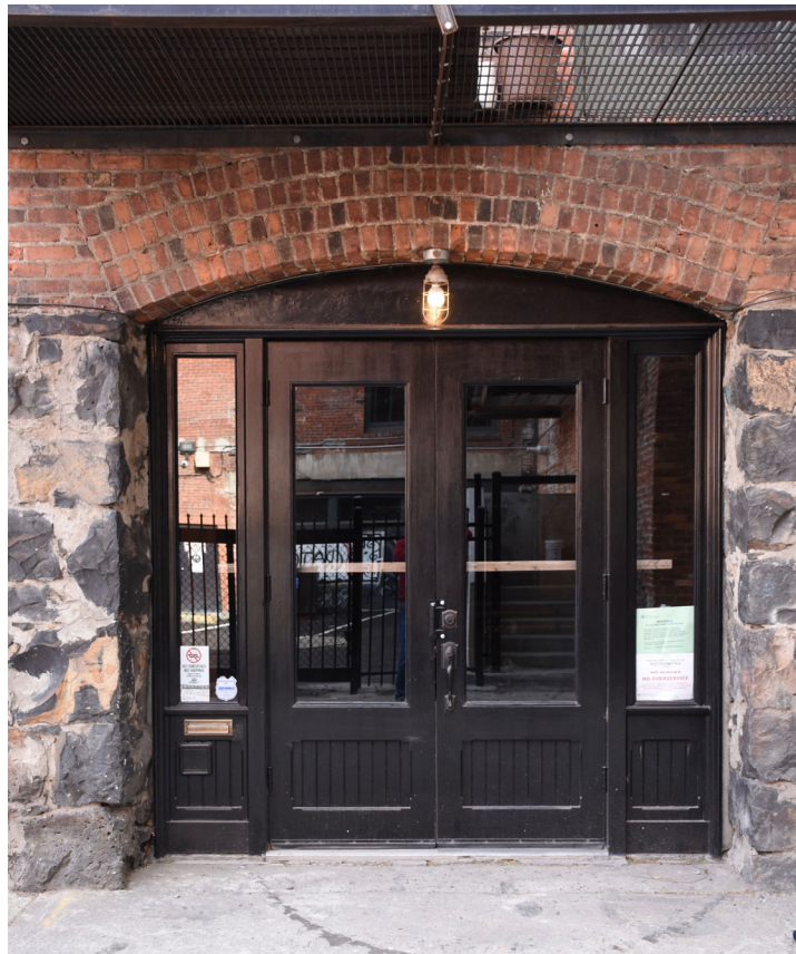
4. North facade-main entry to basement/ground floor
