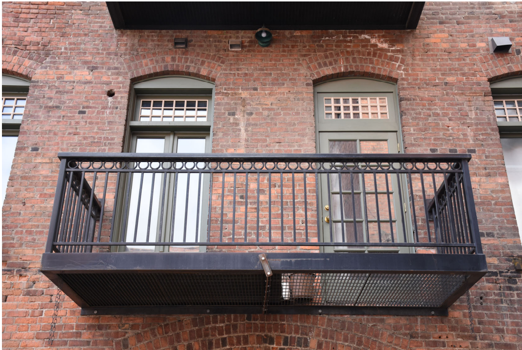
5. North facade-second floor window and door and balcony
