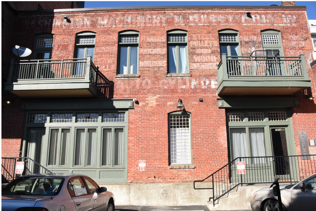
8. South facade, entry to apartments, first and second floor
