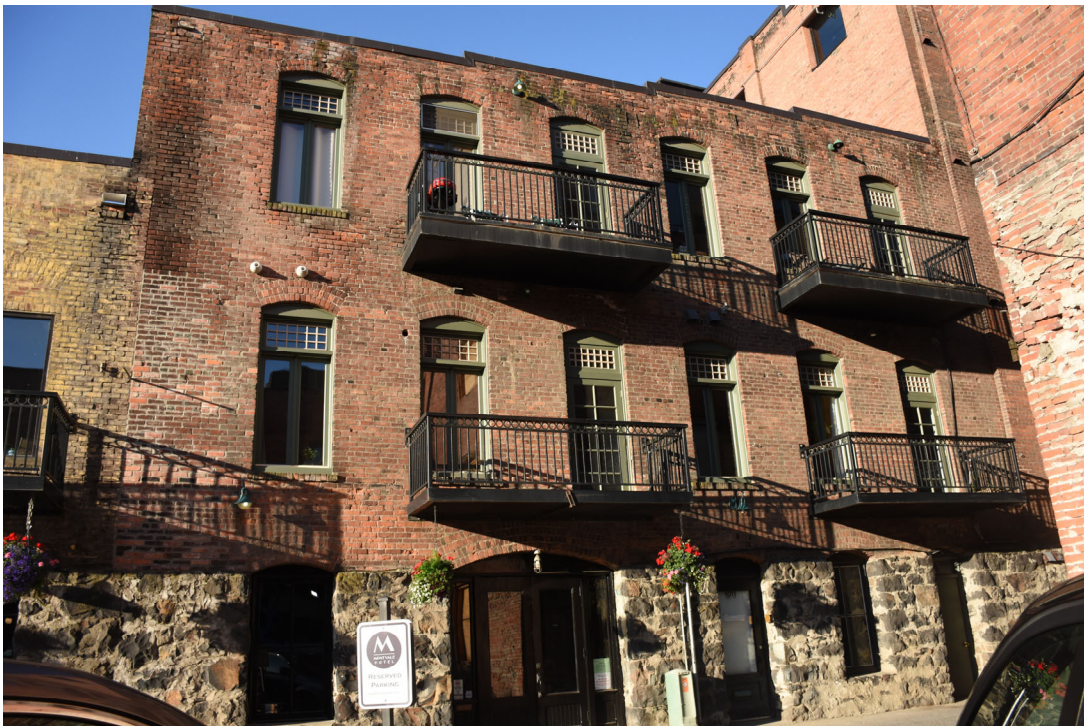
2. North facade-three-story including at grade basement
