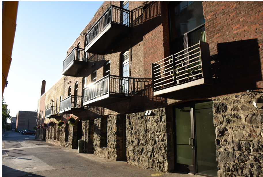
3. North facade-northwest corner adjacent to Washington Rubber Building to west, looking east
