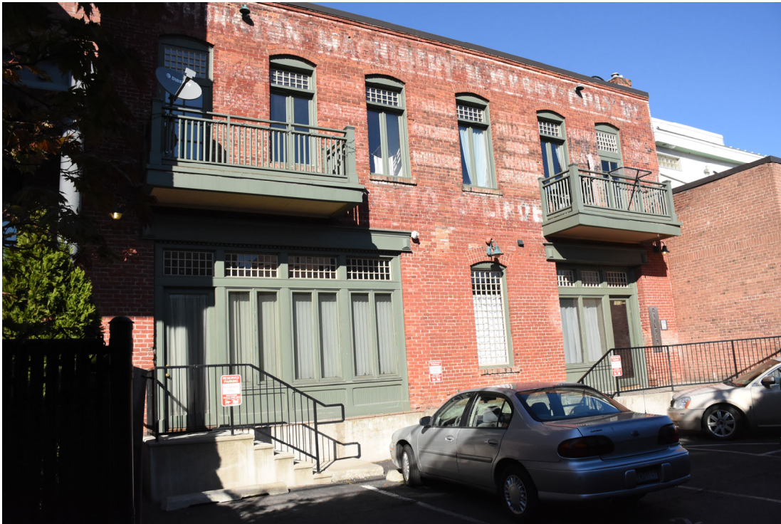
9. South facade-looking northeast
