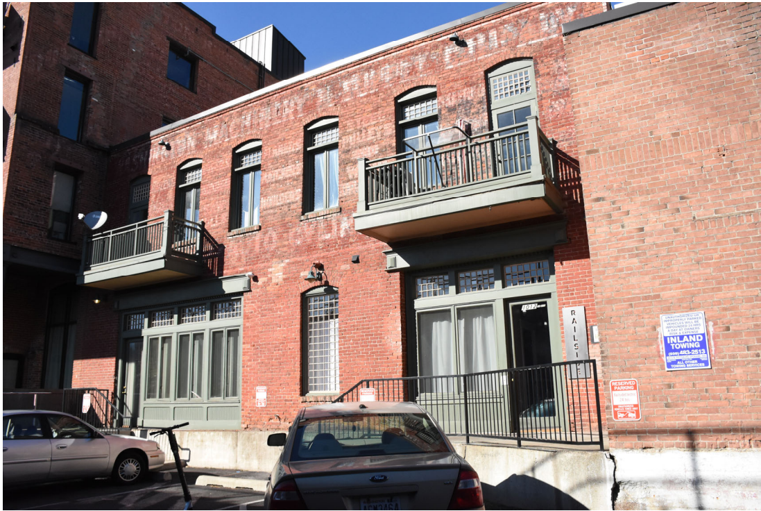
7. South facade-two-story with loading dock, looking northwest
