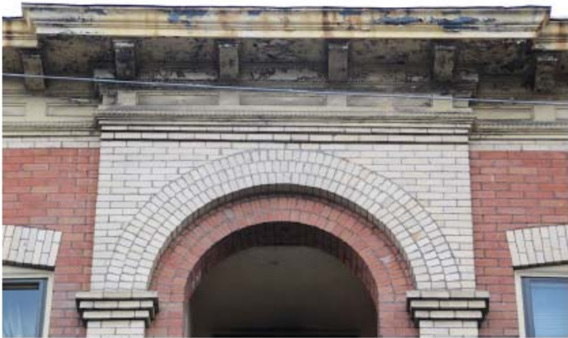
10. Cornice detail, looking south
