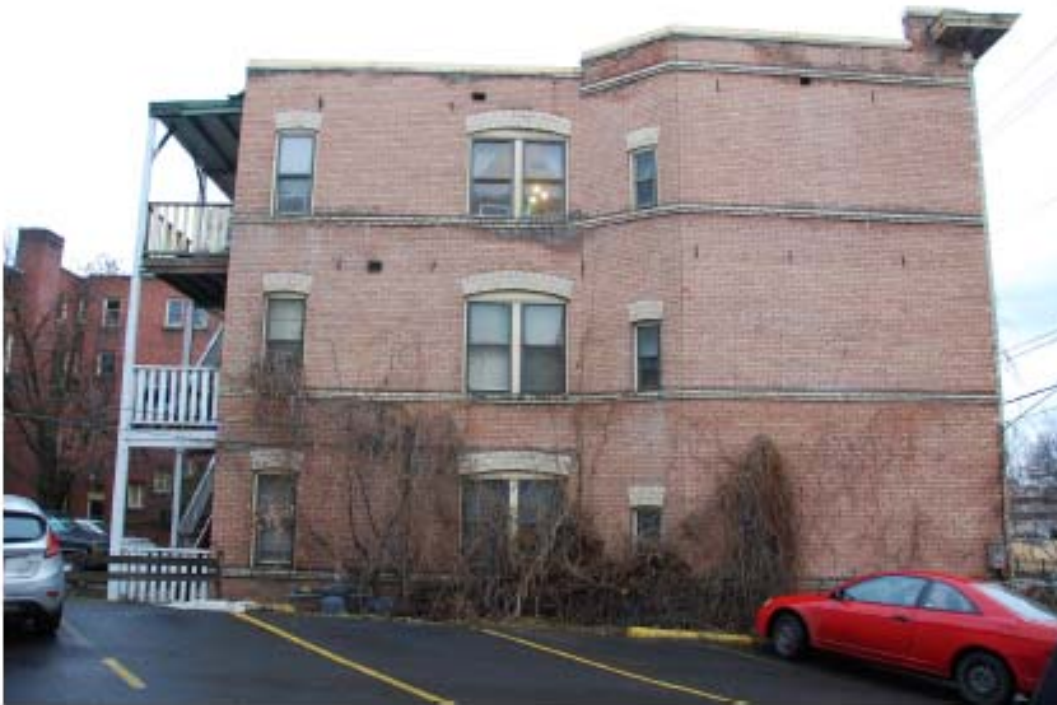
6. East facade, looking west
