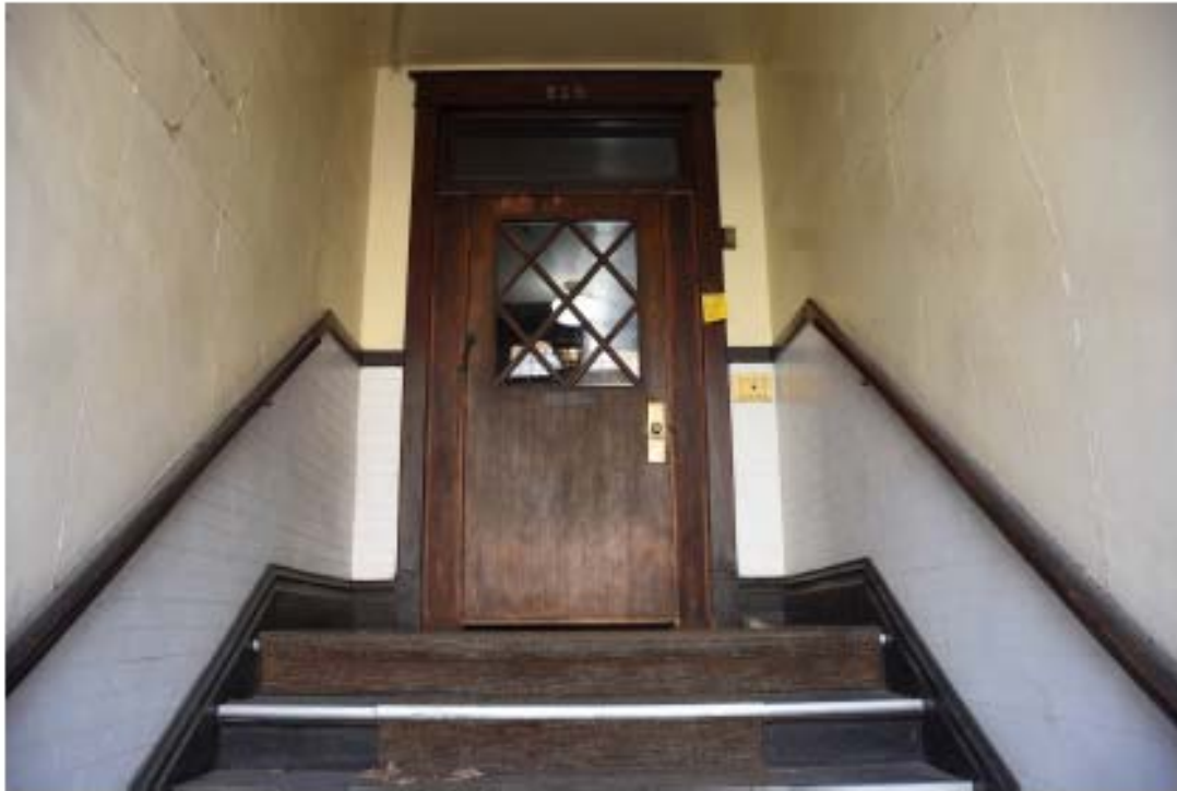
1. Entry alcove - front door to first floor, looking south
