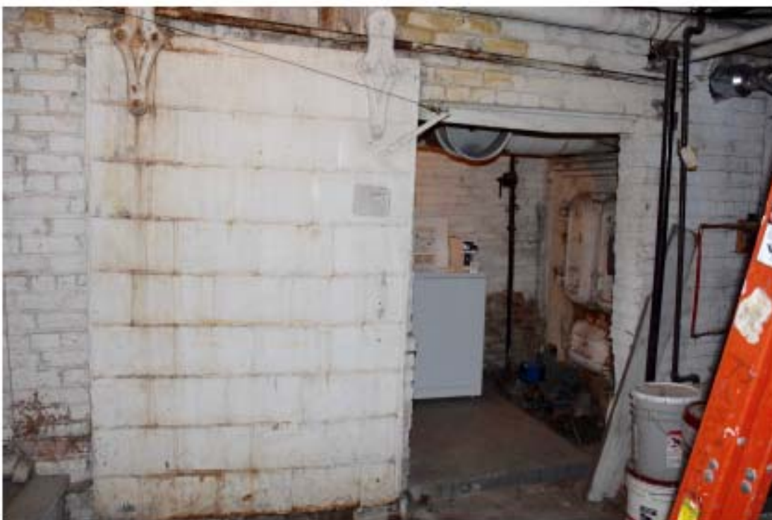
16. Ground level utility room, looking west at furnace room
