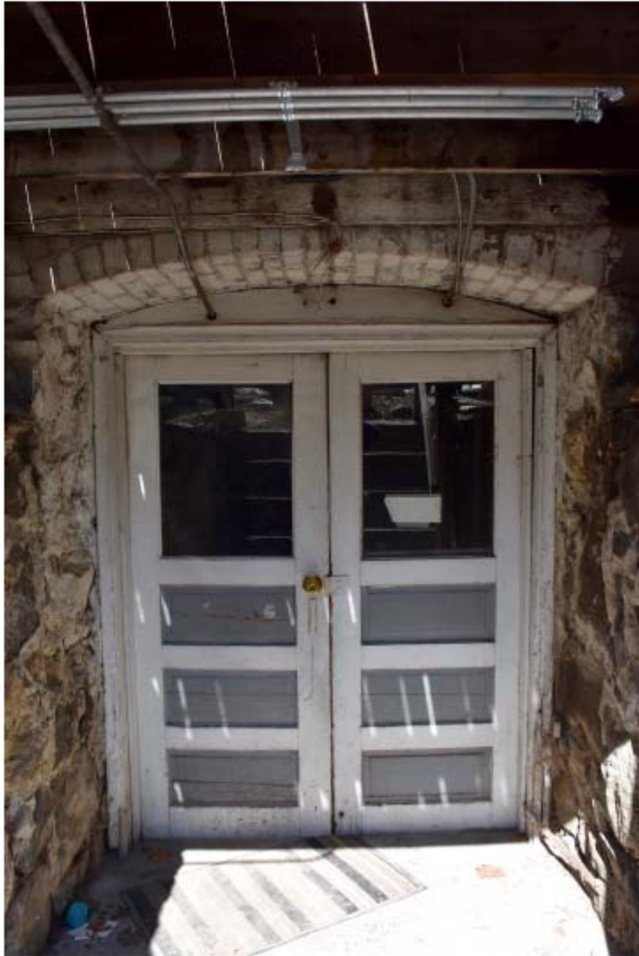
14. Rear entry to ground level utility rooms
