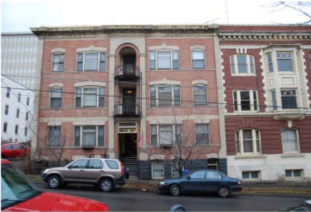
5. Front facade, looking south
