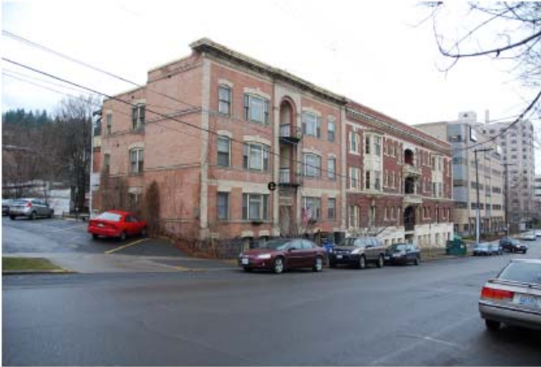
3. Looking southwest at northeast corner - front and east facades
