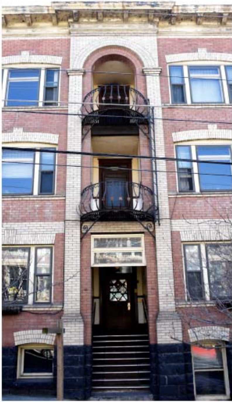
9. Front façade - entry bays, looking south
