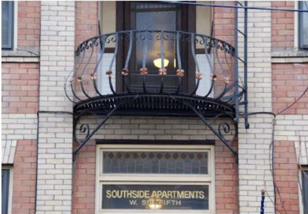
13. Balcony and transom detail
