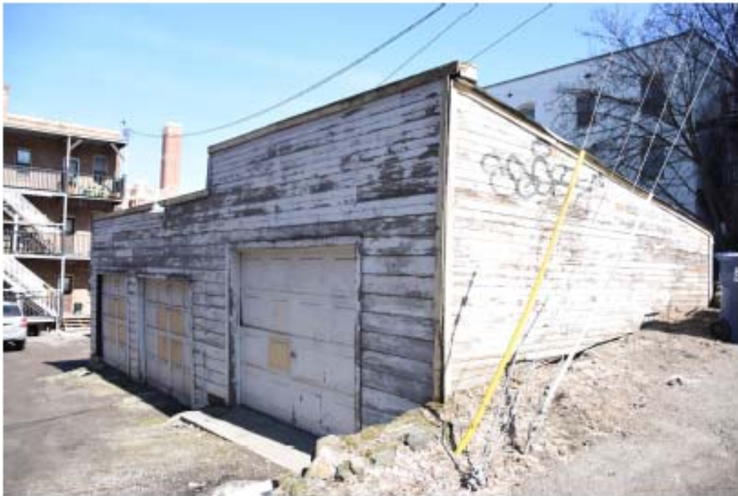
8. The Garage, looking northeast
