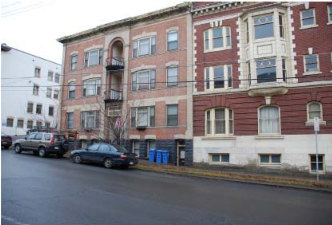
4. Looking southeast at northwest corner - front facade
