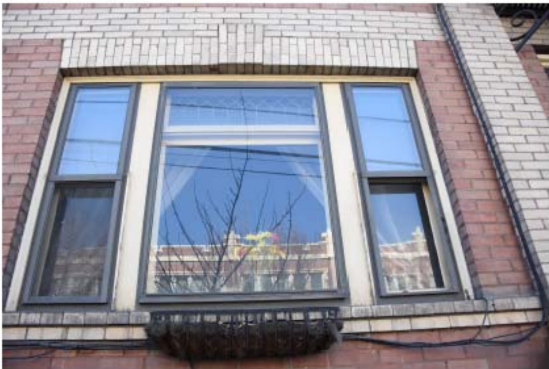
11. First floor window detail (leaded glass)
