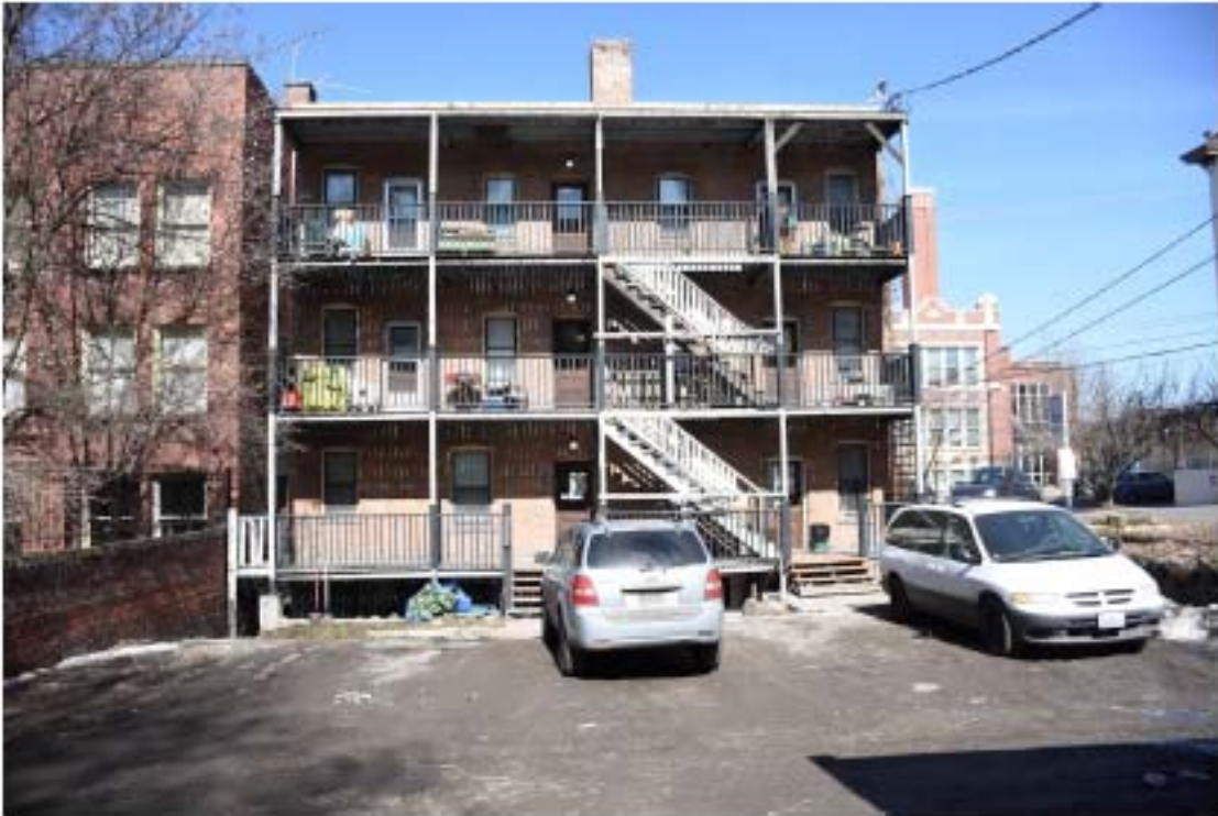
7. Rear facade, looking north
