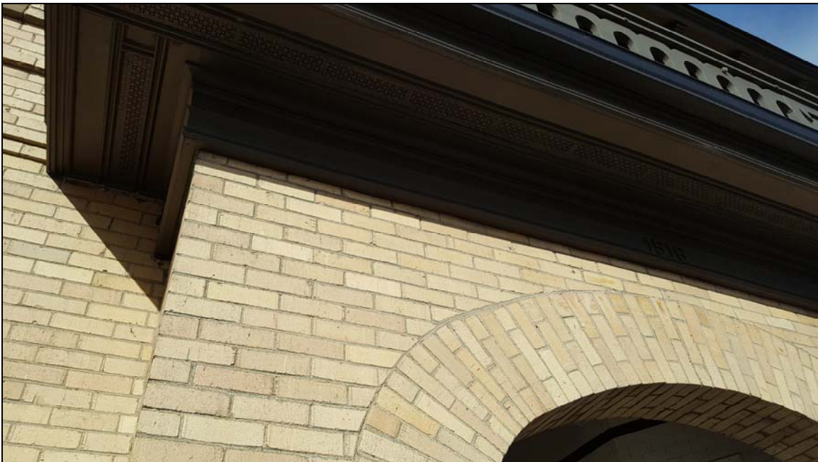
Number 8—south façade front entrance in 2019
