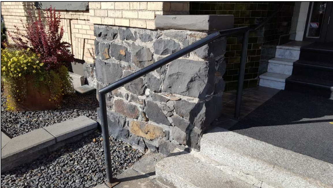
Number 10—south façade front entrance steps in 2019
