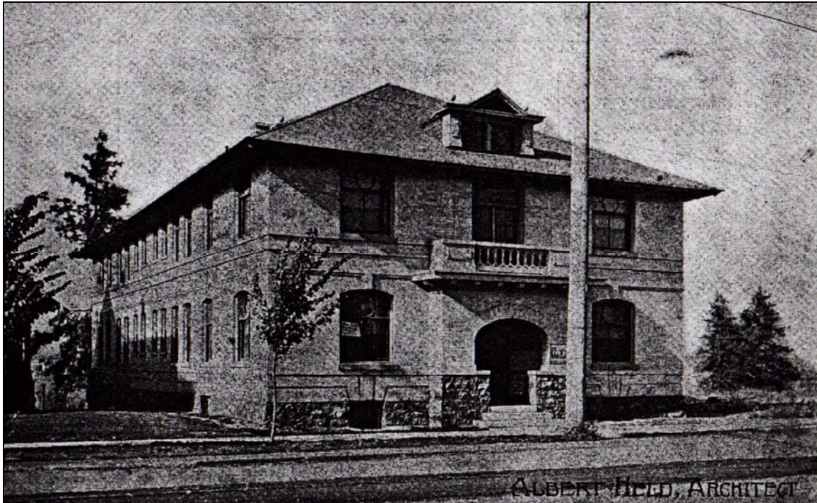
Number 1—1905 photograph of south façade of Ammann Apartments, looking north
