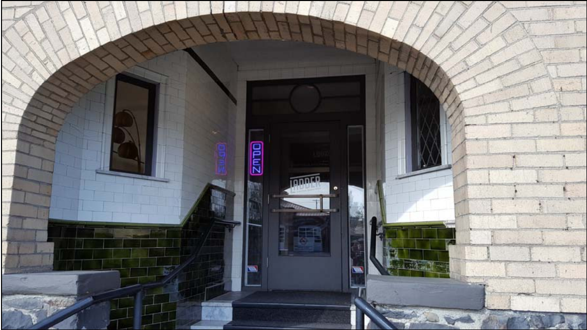
Number 5—Front entrance at south façade, looking north in 2019
