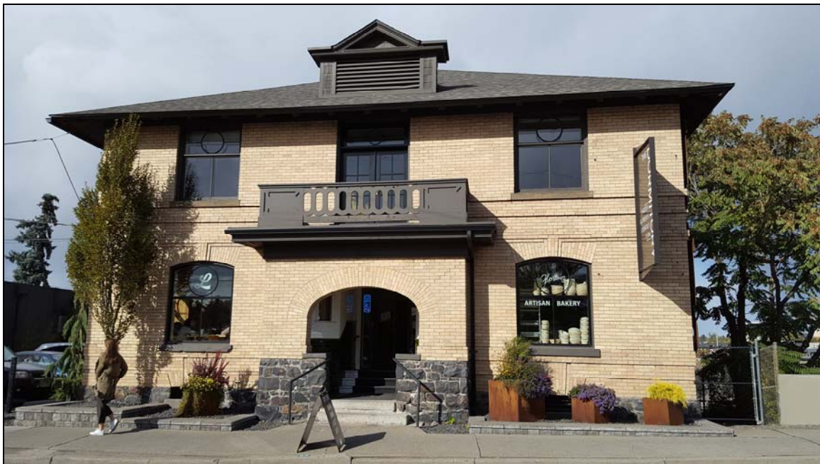
Number 2—2019 photograph of south façade of Ammann Apartments, looking north
