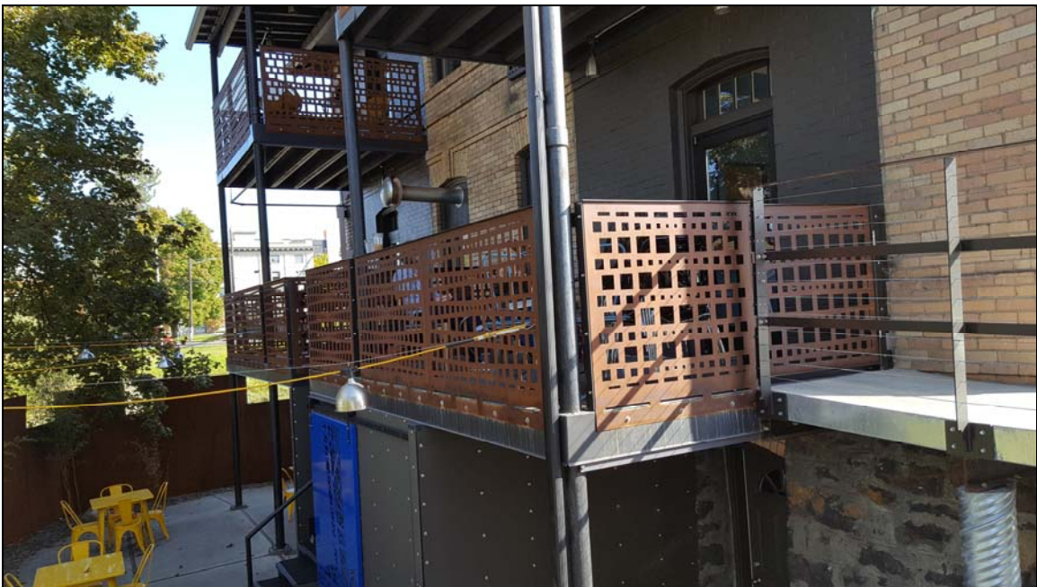
Number 12—north rear face first and second-floor balconies in 2019
