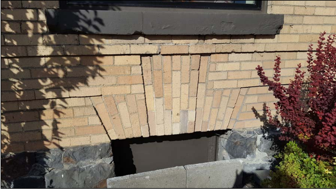
Number 9—south façade brick detail in 2019
