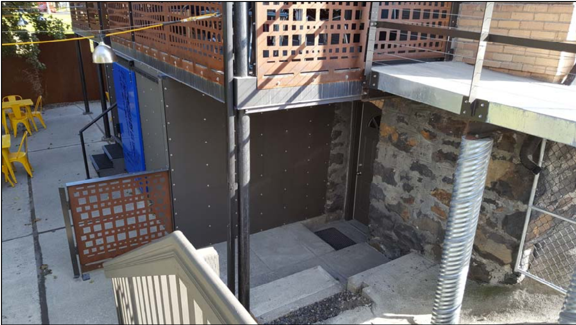
Number 13—north rear face first-floor balcony and basement level in 2019
