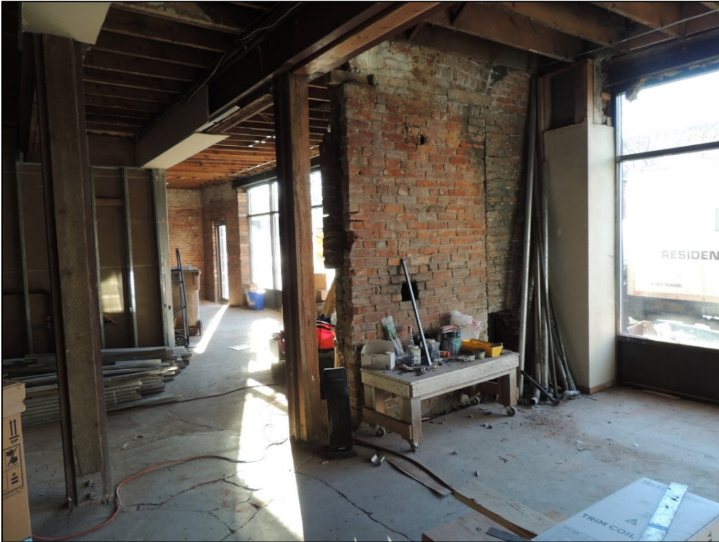
Logan Camporeale, "First floor near middle of building facing southwest, partial brick wall shows division between original building and c.1902 addition," December 6, 2018, Spokane Historic Preservation Office Photographs.
