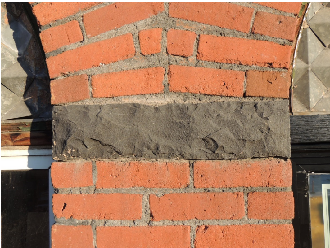
Logan Camporeale, "Third floor windows with granite detailing," December 6, 2018, Spokane Historic Preservation Office Photographs.
