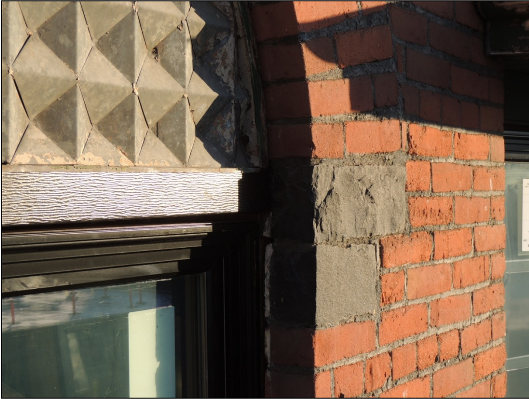
Logan Camporeale, "Third floor windows with granite detailing" December 6, 2018, Spokane Historic Preservation Office Photographs.
