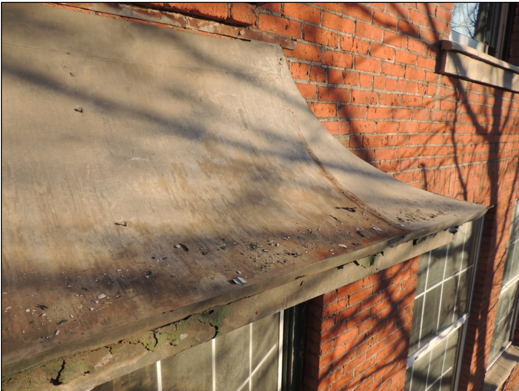
Logan Camporeale, "Metal roof over second floor oriel bay window," December 6, 2018, Spokane Historic Preservation Office Photographs.
