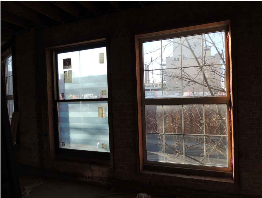
Logan Camporeale, "Replacement vinyl windows on right and new metal clad wood windows on left," December 6, 2018, Spokane Historic Preservation Office Photographs.
