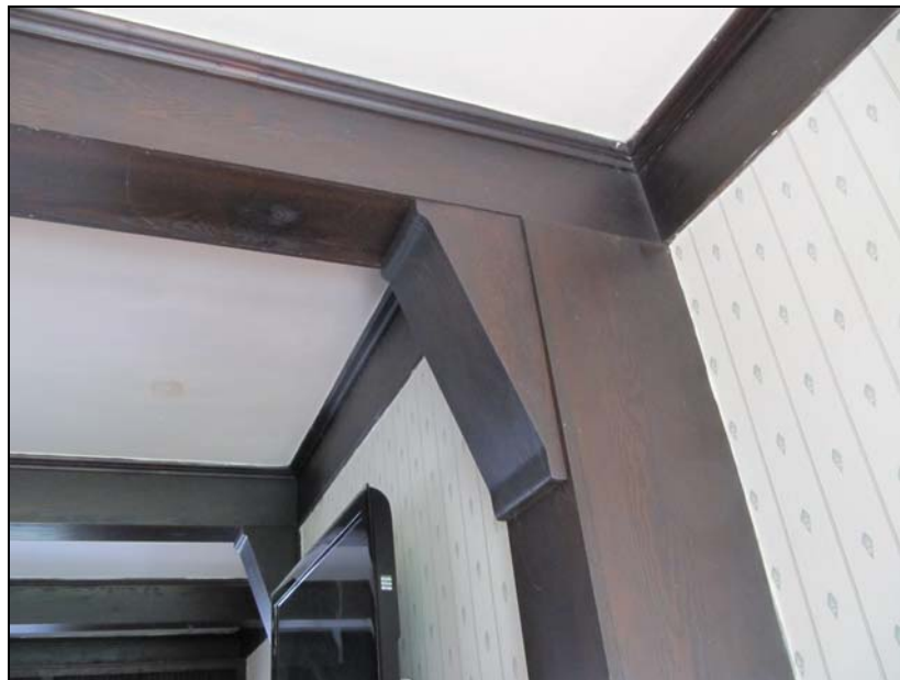
1905 ceiling beam bracket
