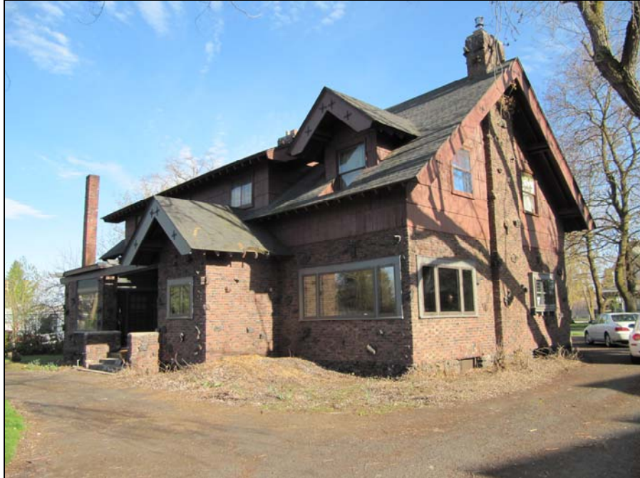
Northwest façade corner in 2017
