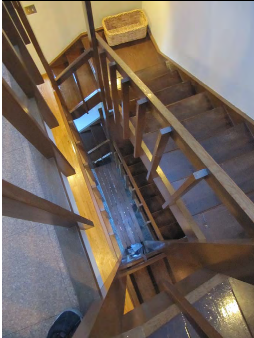
Overhead view, looking down at stairwell in Trogdon House in 2016
