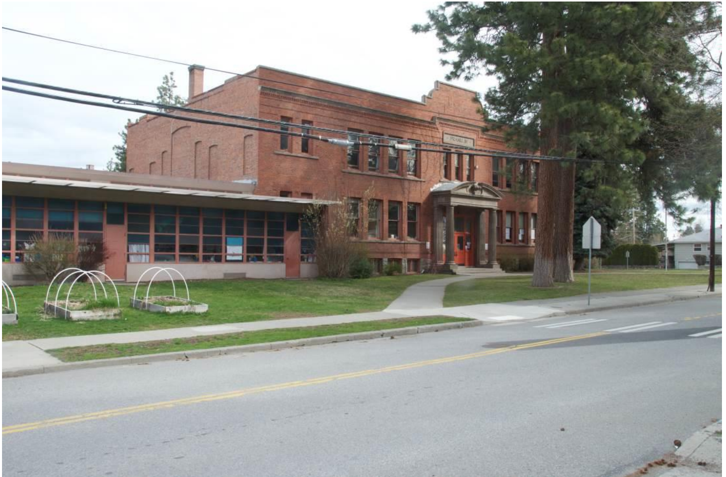
1 of 28 Main façade of school showing original 1909 building and 1953 addition - Looking northeast
