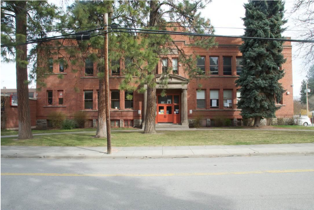
2 of 28 Main Façade - Looking north
