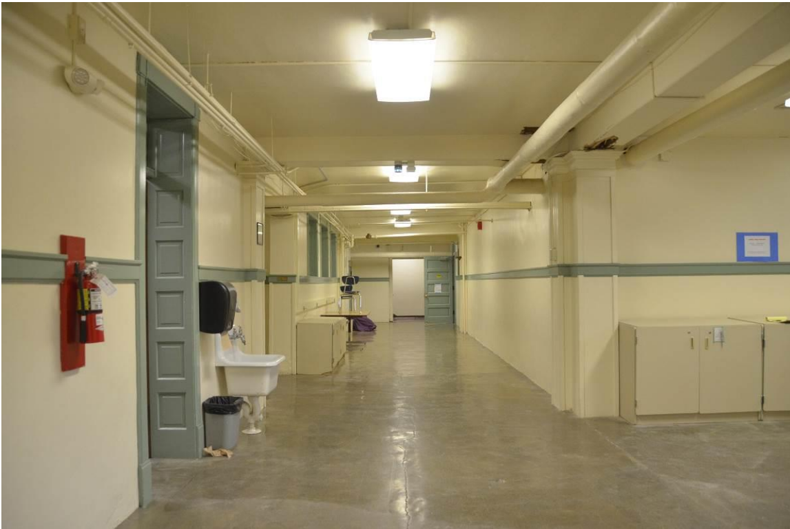
20 of 28 1909 building, Basement Hall looking west
