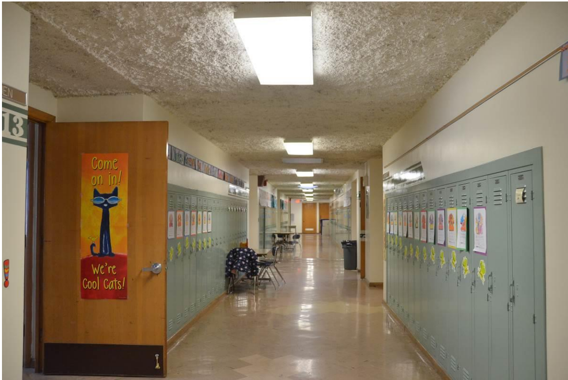
22 of 28 1953 addition, classroom hallway looking west.
