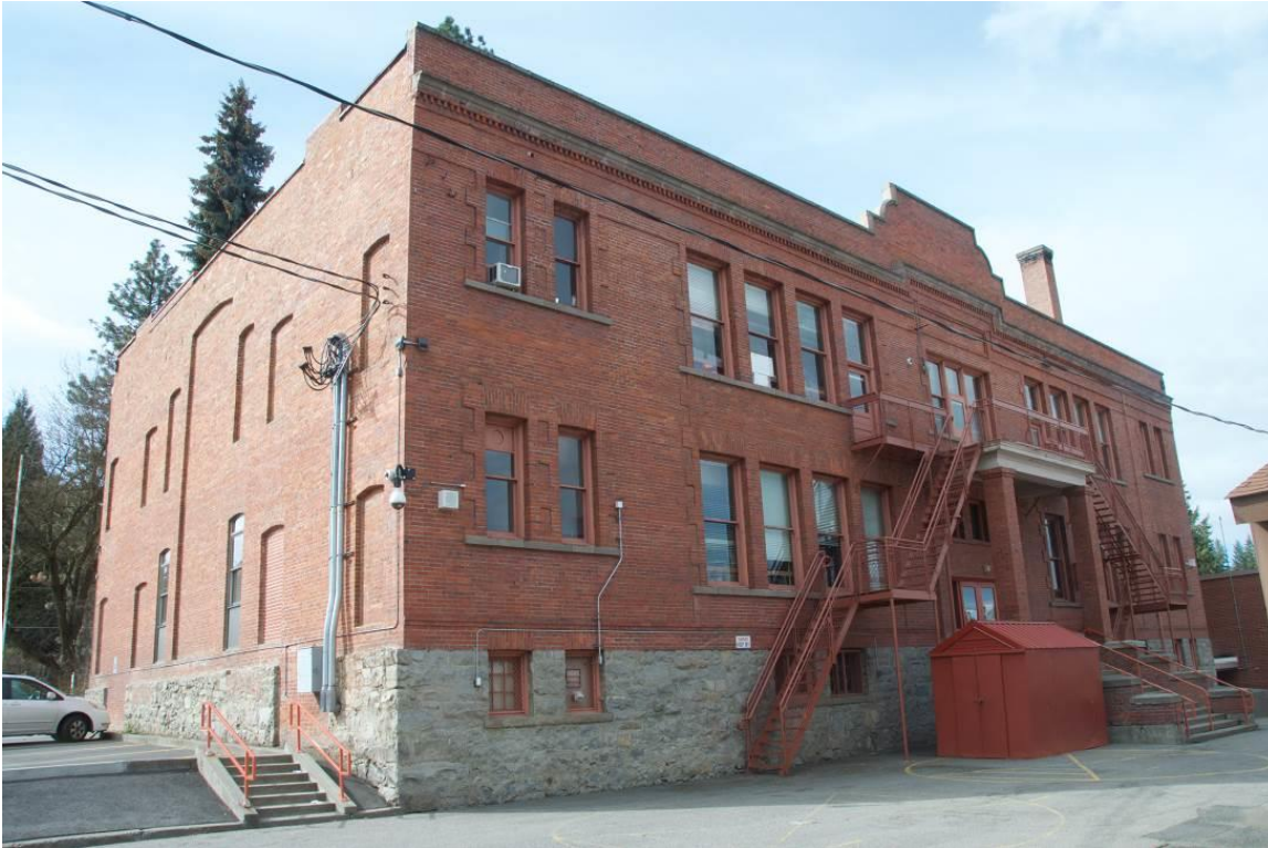
4 of 28 Rear façade, northeast corner - Looking southwest
