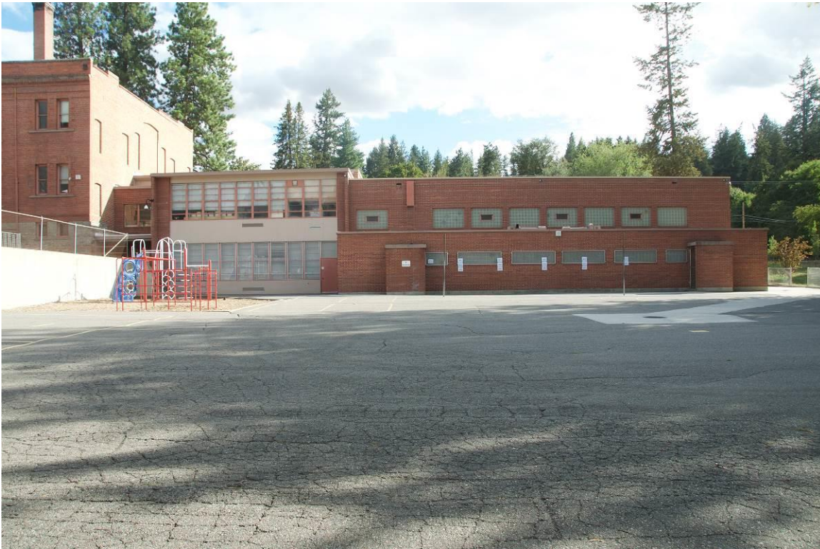
8 of 28 Rear facade of 1953 addition - Looking south
