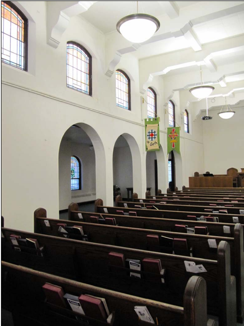
1923 church nave (auditorium), looking northwest towards the sanctuary at the front of church in 2016.
