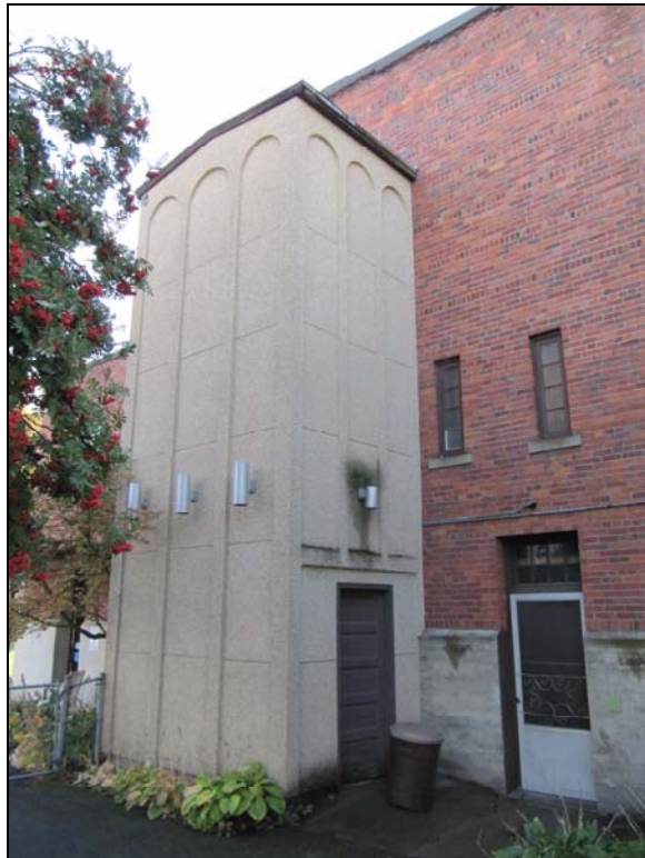
North rear elevation of 1923 church in 2016.
