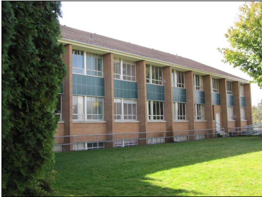
North rear elevation of 1959 addition in 2016.
