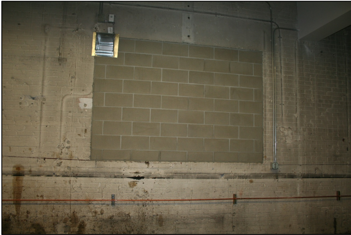
DB-15 First floor, rear parking area, filled in window, view to the east.
