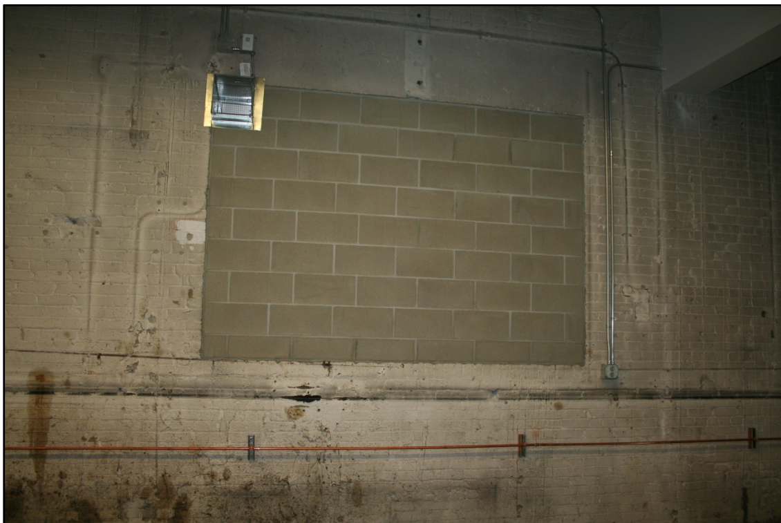
DB-20 Second floor, filled in window space on south wall, view to the south.
