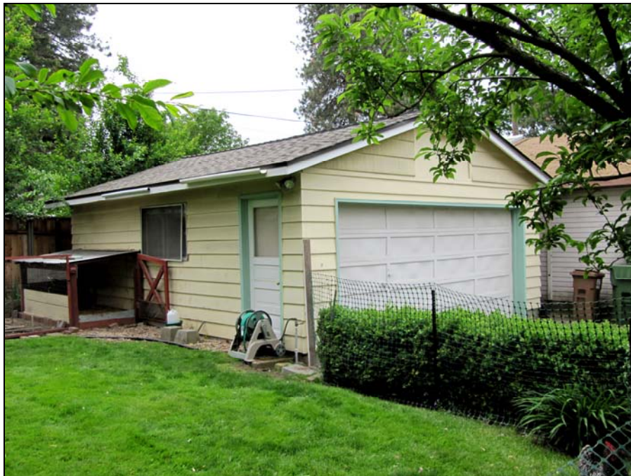
Rock retaining wall in 2016. Double-car garage in 2016.
