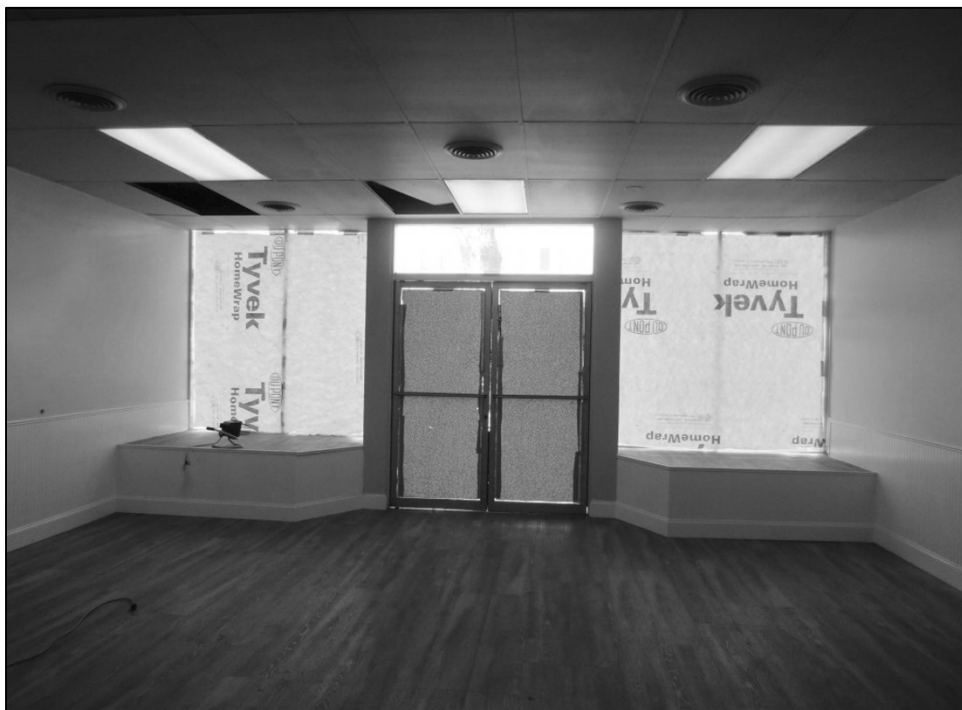
Interior of 821 looking north.
