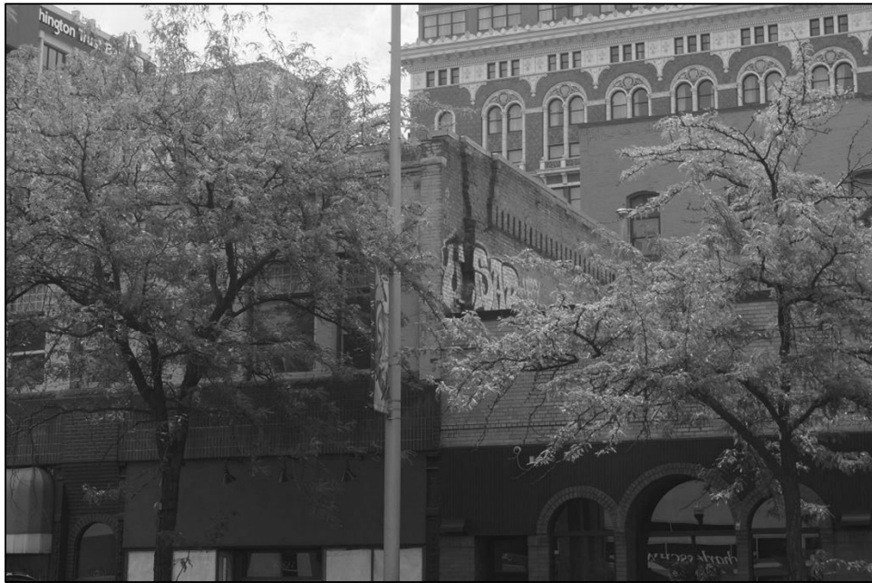
Detail of northwest oblique.
