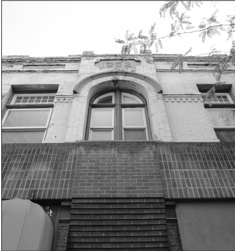
Detail of "1892" on second story of north façade.
