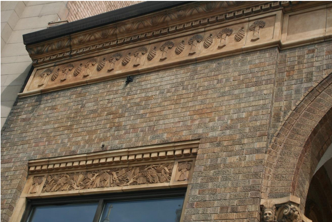
SCB-7 Window lintel and cornice designs, south (front) elevation, view to the northwest.
