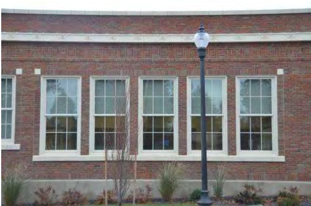
Photo 8 - East Facade Showing Wall and Window Detail - Looking West.
