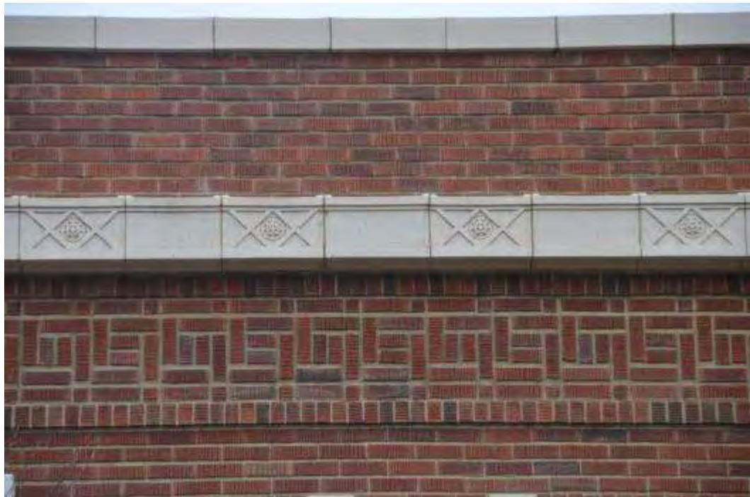
Photo 14 - Parapet, Belt Course & Brick Pattern- Typical
