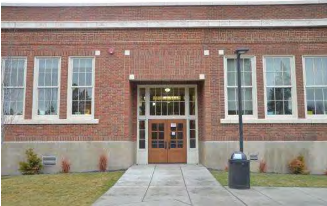
Photo 13 - South Facade - Historic Entry & Juncture of Historic Addition to South Wing
