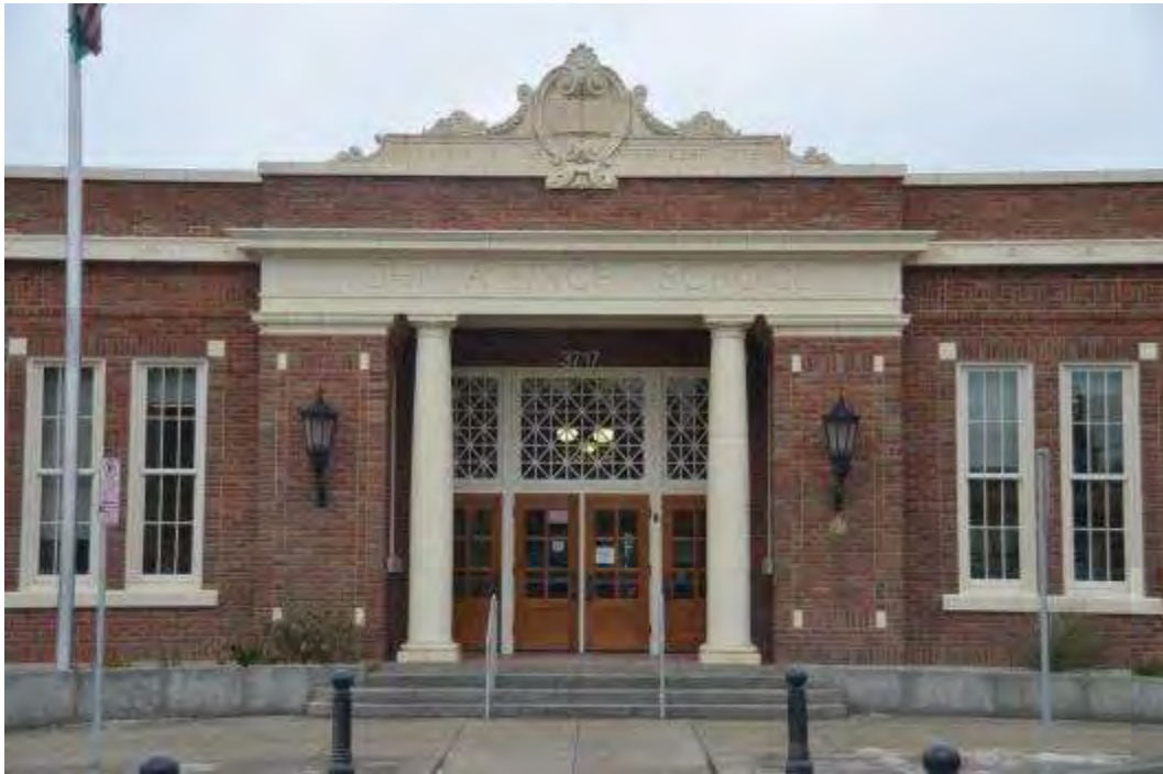
Photo 15 - Main Entry - East Facade
