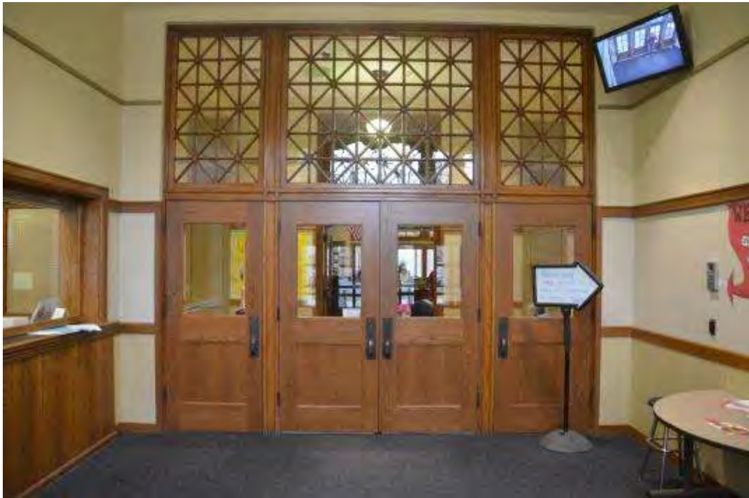
Photo 19 – Front Entry Vestibule - Looking West
