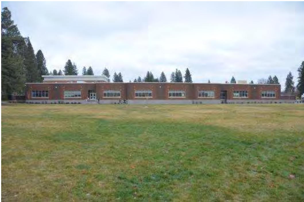
Photo 4 - New West Wing Addition - Looking East
