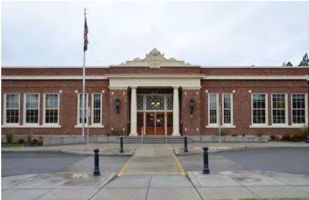
Photo 7 - East (Front) Facade Showing Main Entry - Looking West
