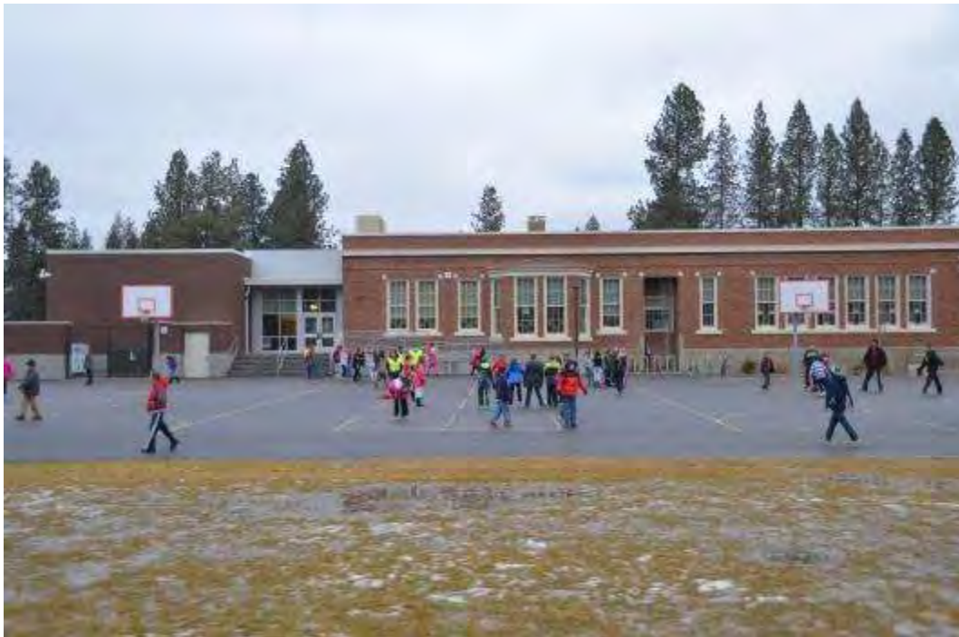
Photo 12 - Juncture of New West Wing and Historic South Facade
