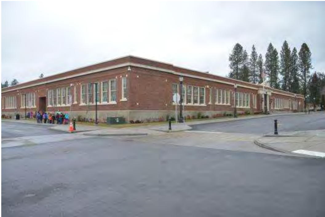
Photo 1 - SE Corner - East & South Facades - Looking NW
