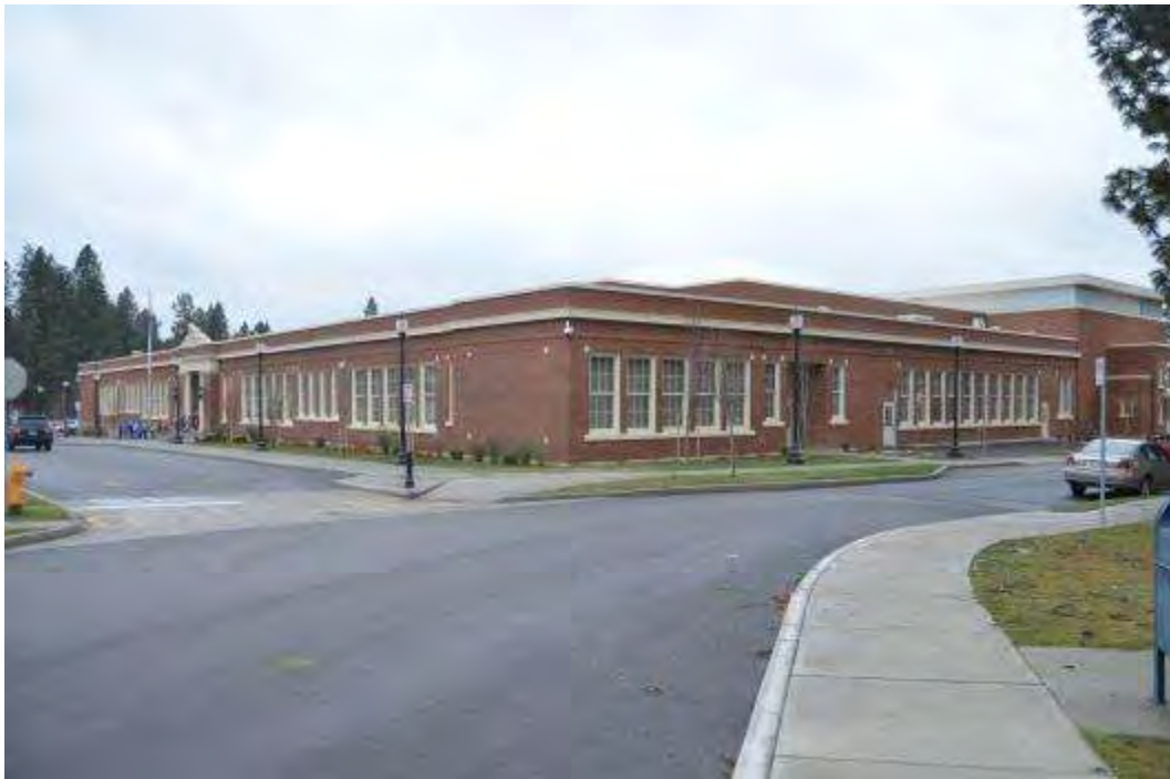
Photo 2 - NE Corner - East & North Facades - Looking SW
