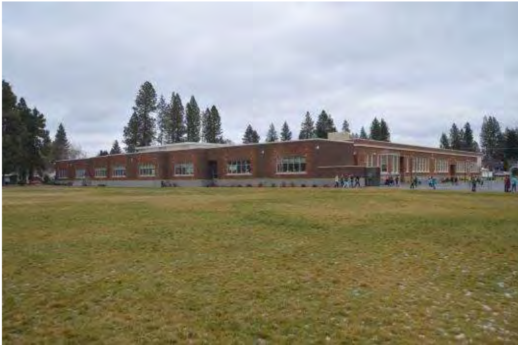
Photo 5 - SW Corner Showing New West Wing & Historic South Facade
