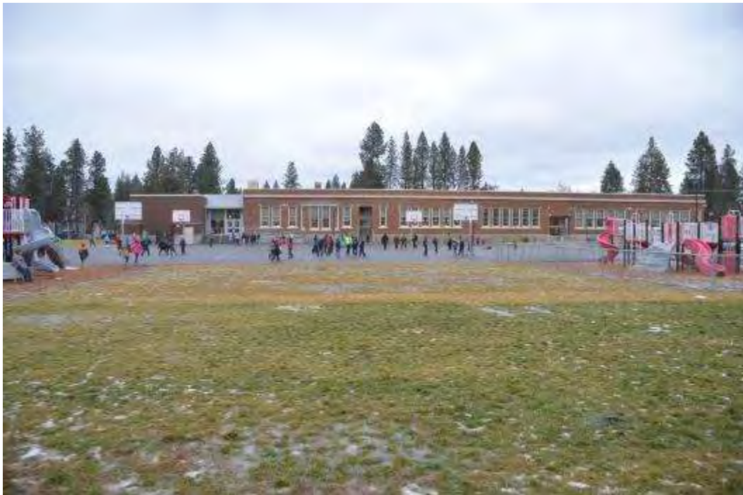
Photo 6 - South Facade - Looking North Juncture of New West Wing and Historic Wing
