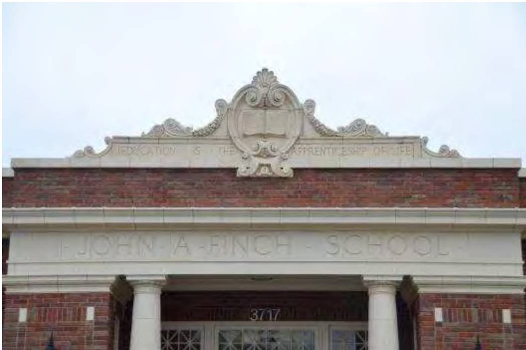
Photo 16 - Main Entry Pediment
