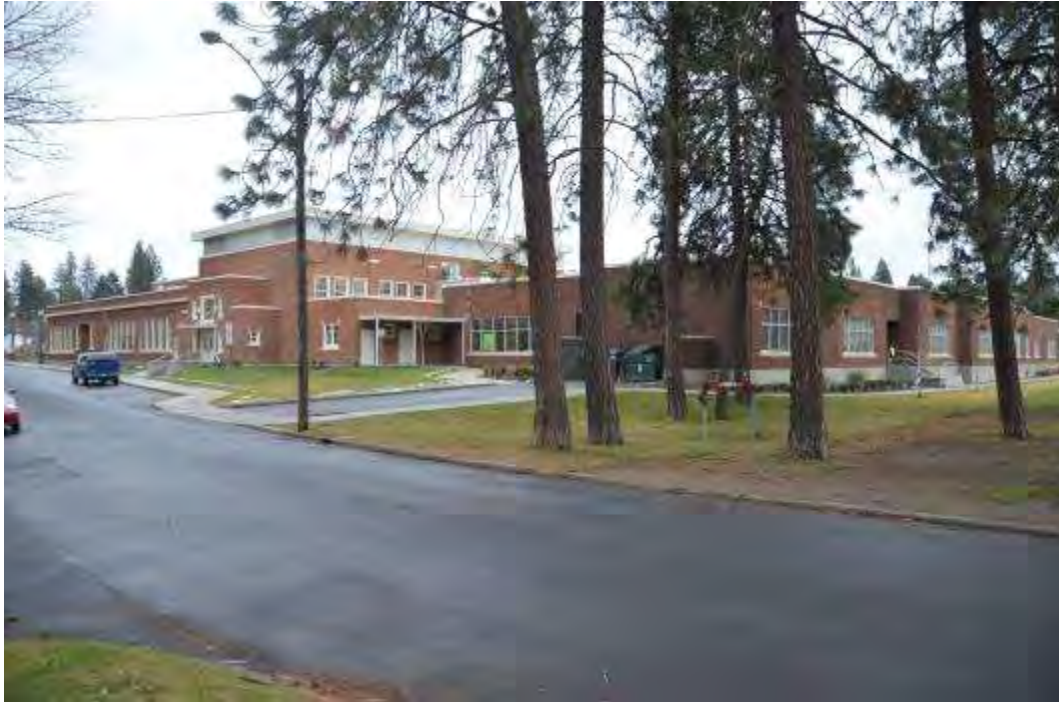
Photo 3 - NW Corner - Looking SE
