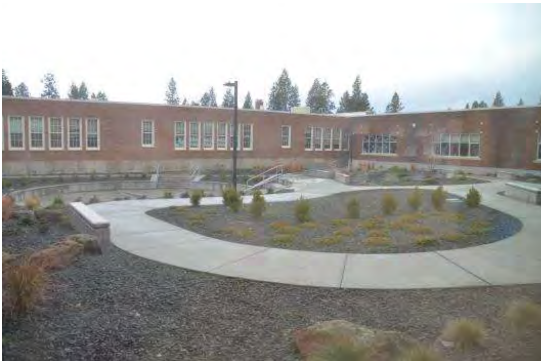
Photo 28 - Courtyard - Looking Southwest - Historic Wing and West Addition
