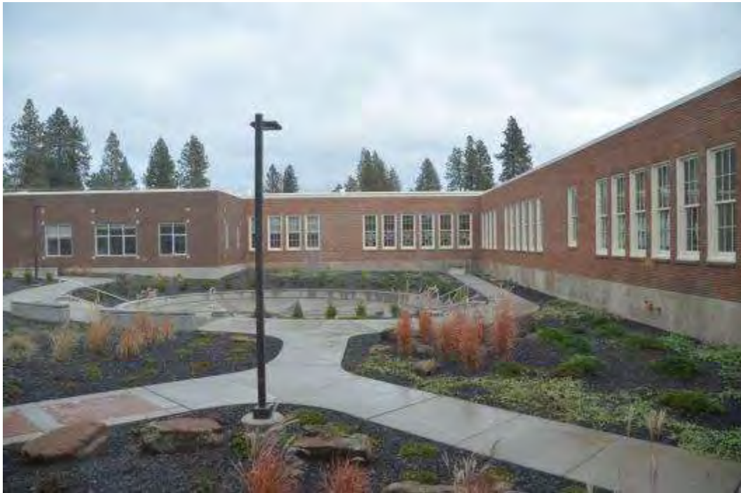
Photo 27 - Courtyard - Looking East at Historic South & East Wings With 2014 Addition
