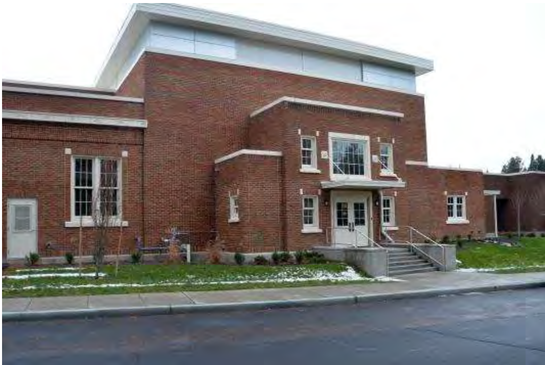
Photo 10 - Gymnasium & Entrance - Looking SW Toward New Addition
