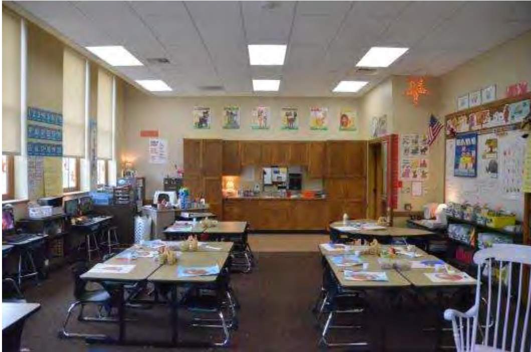
Photo 23 - Classroom 120 - Looking West
