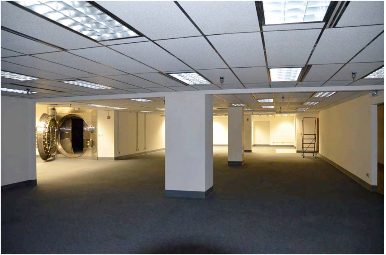
Photo 7– View to of Basement Looking to North and Toward Vault
