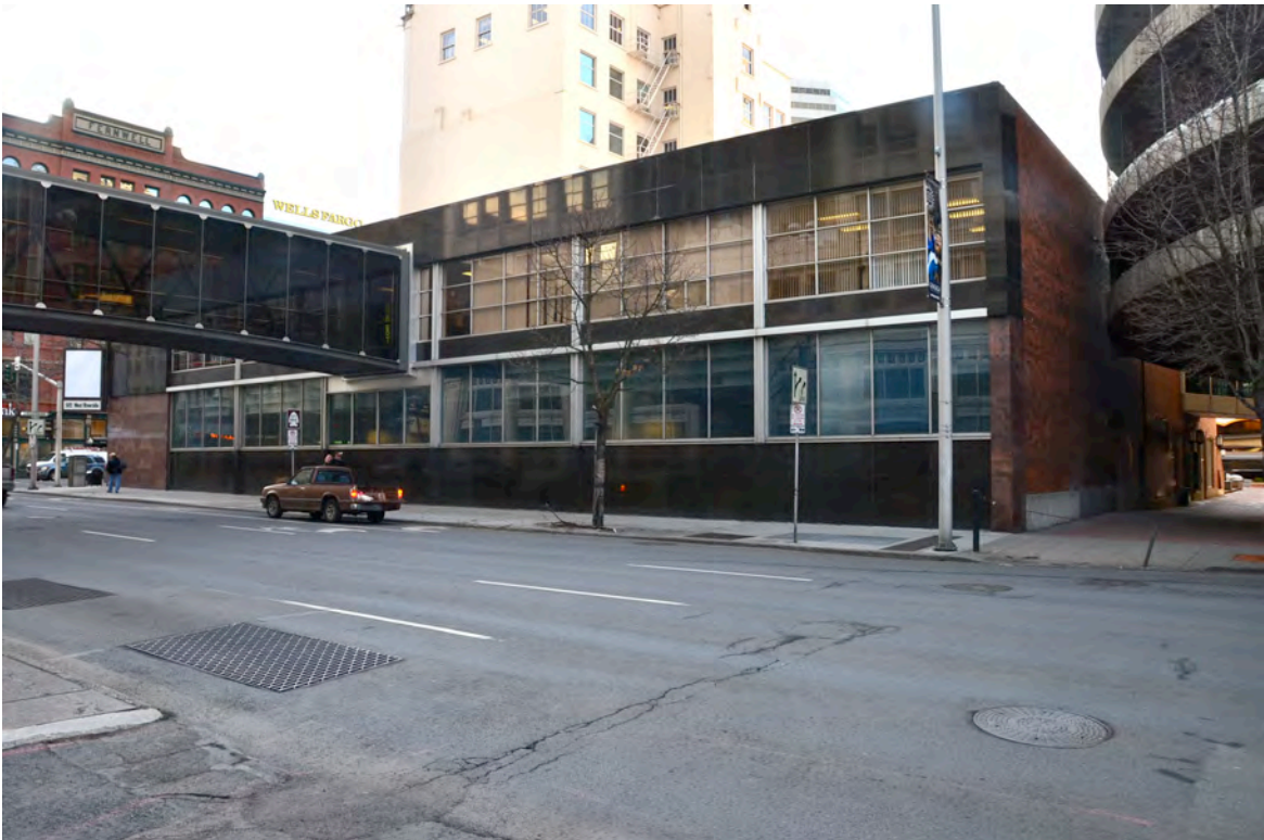
Photo 6 – View to Northwest Showing Northeast Corner and Skywalk
