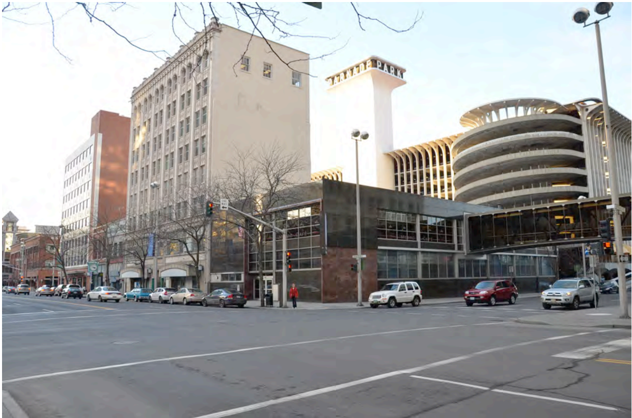
Photo 2 – View to Northwest Showing Site Context From Stevens and Riverside
