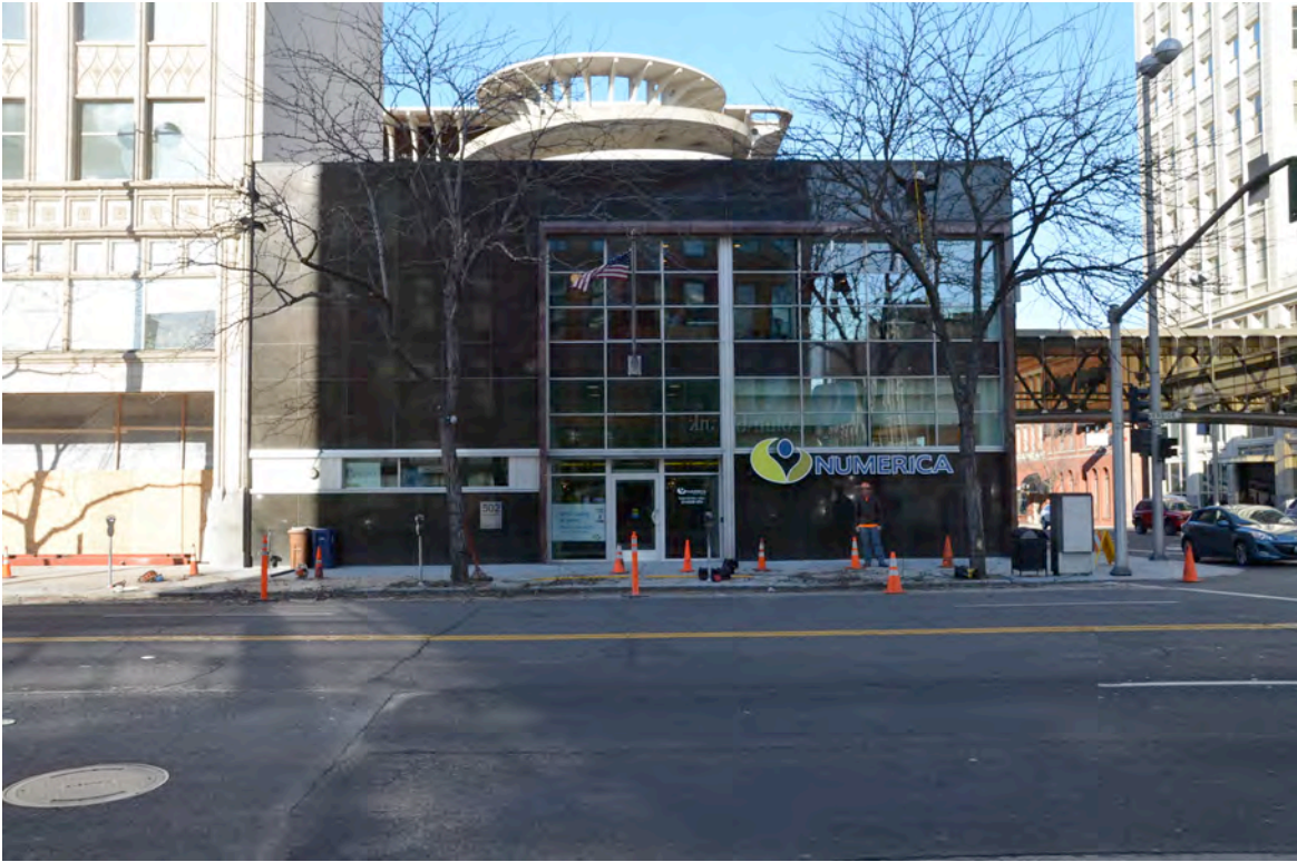
Photo 4 – View to North Showing Front of FNB Along Riverside Avenue
