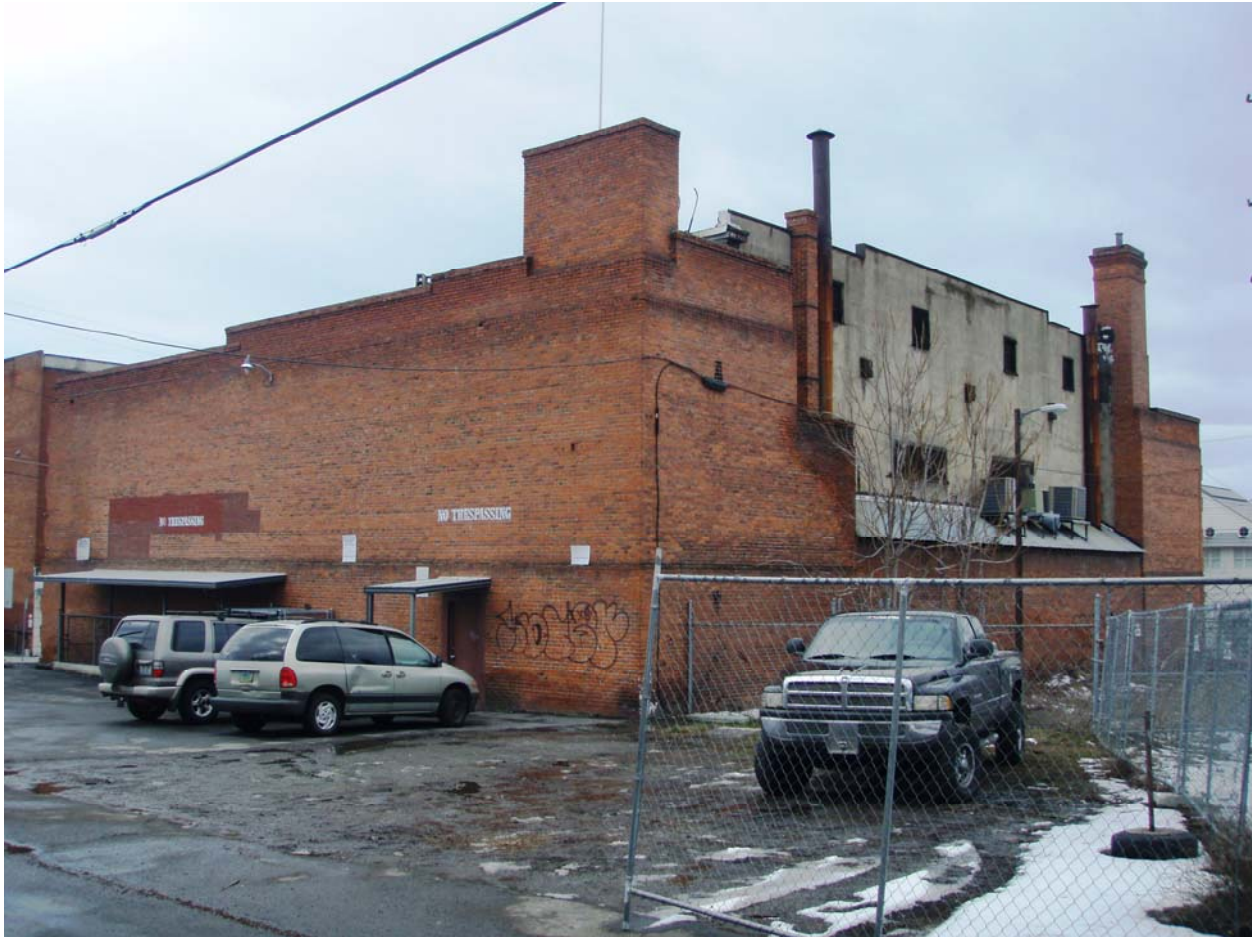
Photo #5 [View: NW; Oblique of South and East elevations] March 14, 2011
