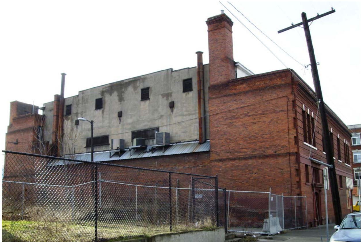
Photo #6 [View: SW; Oblique of North and East elevations] March 14, 2011
