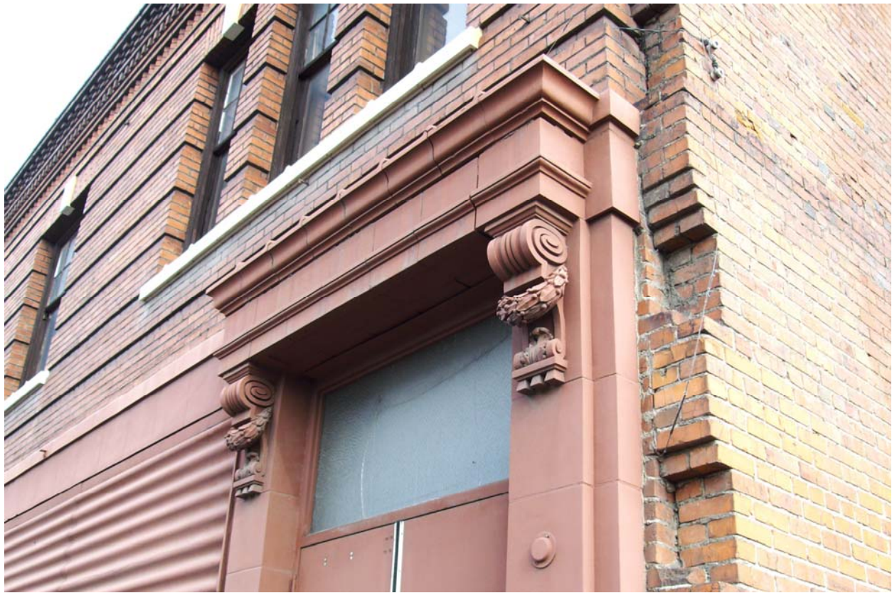
Photo #10 [View: NE; Detail of entrance on Browne] March 14, 2011
