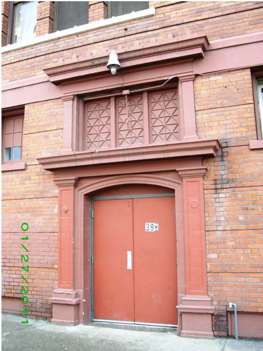
Photo #8 [View: SE; North elevation primary entrance] January 27, 2011
