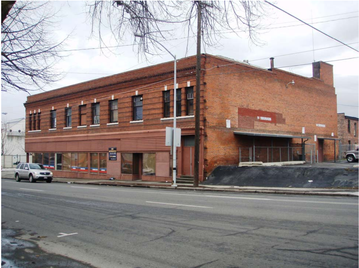
Photo #3 [View: NE; Oblique of South and West elevations from Browne] March 14, 2011
