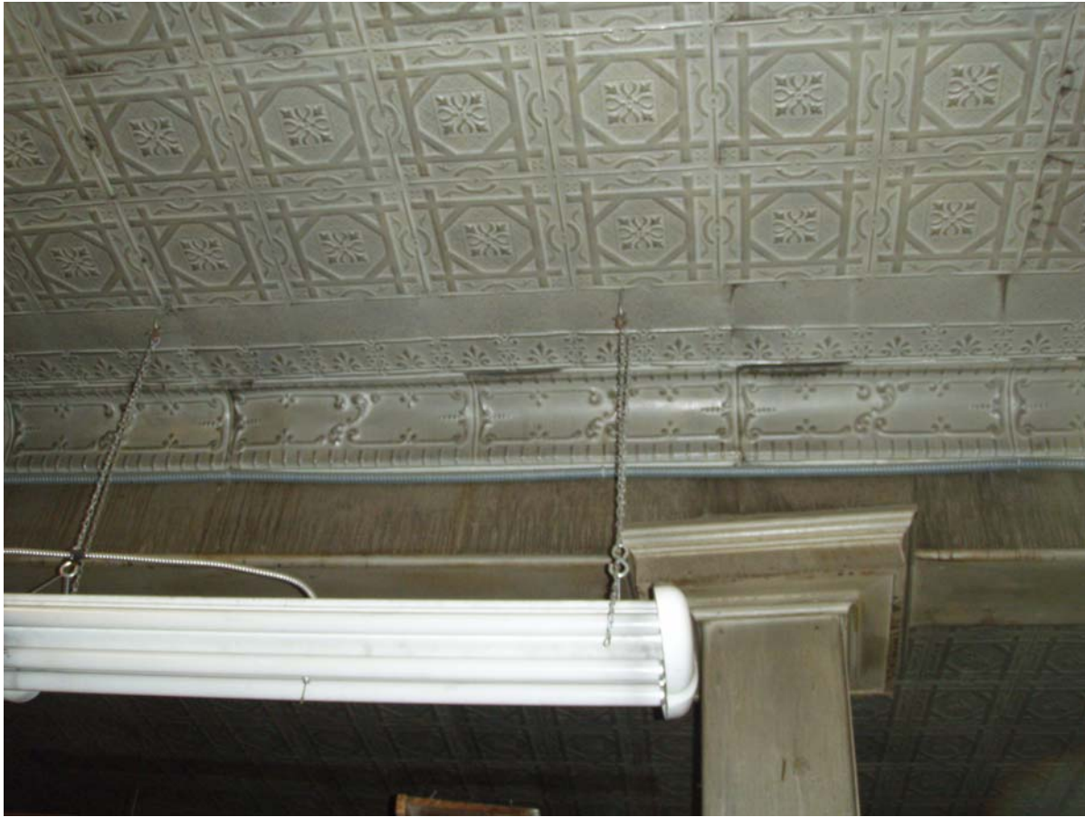
Photo #16: [Original cast tin ceiling detail and column on first floor] March 14, 2011
