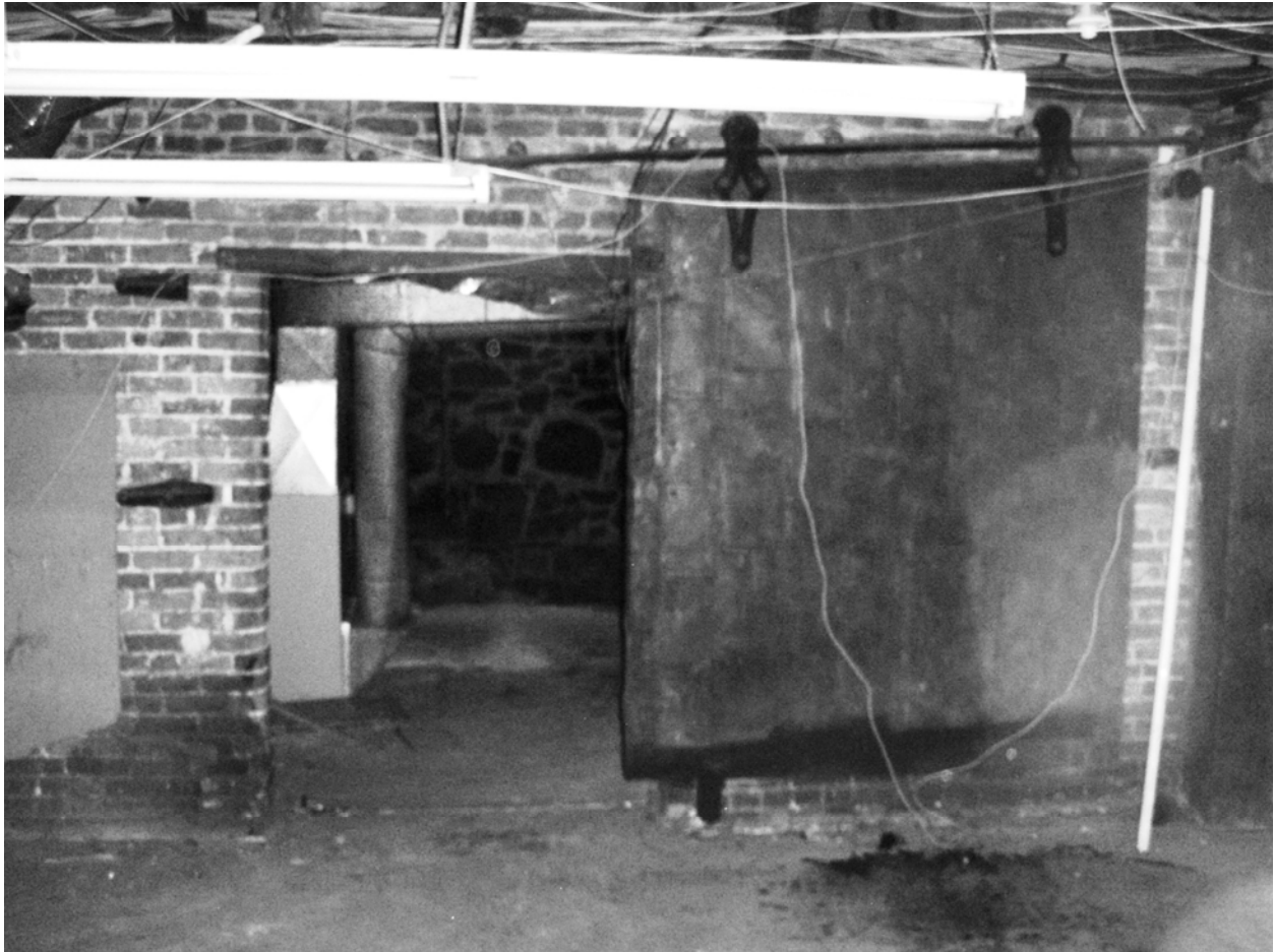
Photo #19 [Basement sliding door with original hardware and exposed brick walls] March 14, 2011
