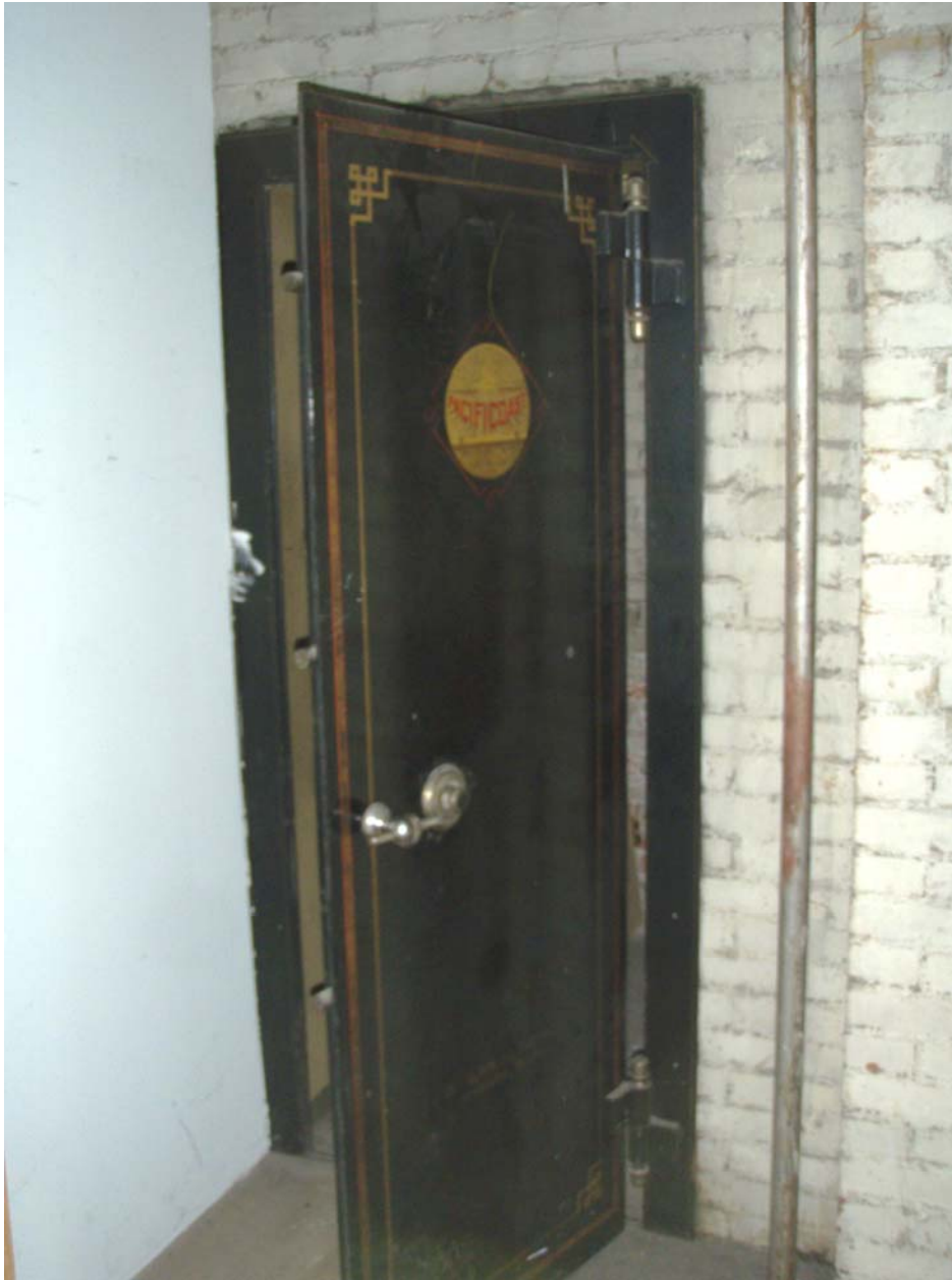
Photo #17 [Original safe on first floor] March 14, 2011
