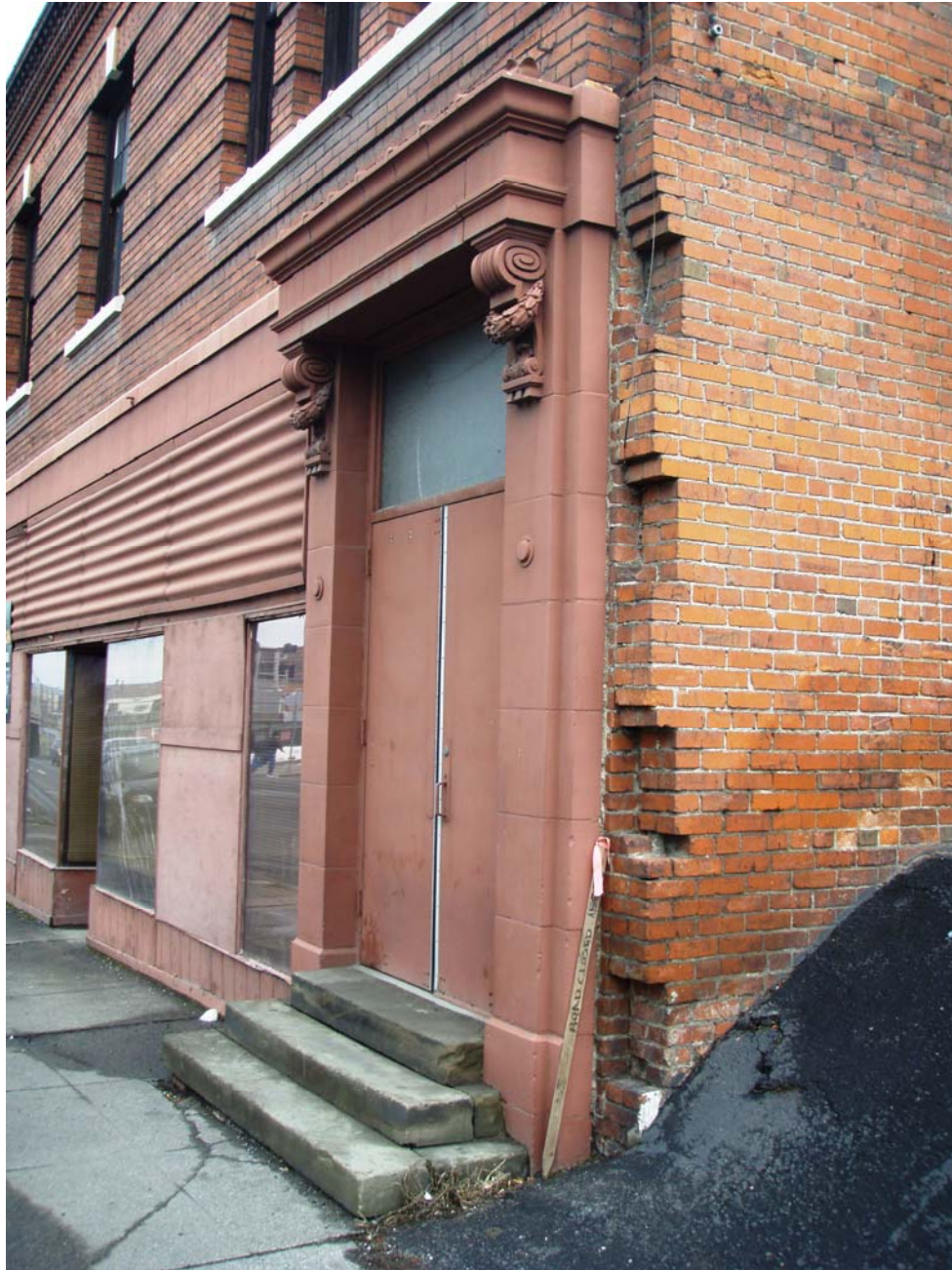
Photo #9 [View: NE; Oblique of South and West elevations and entrance on Browne] March 14, 2011
