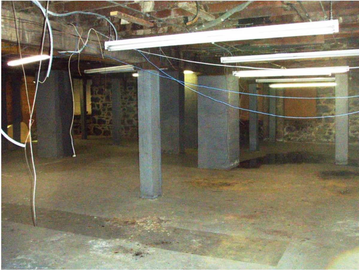
Photo #18 [Basement with structural supports, ceiling beams, exposed stone walls] March 14, 2011
