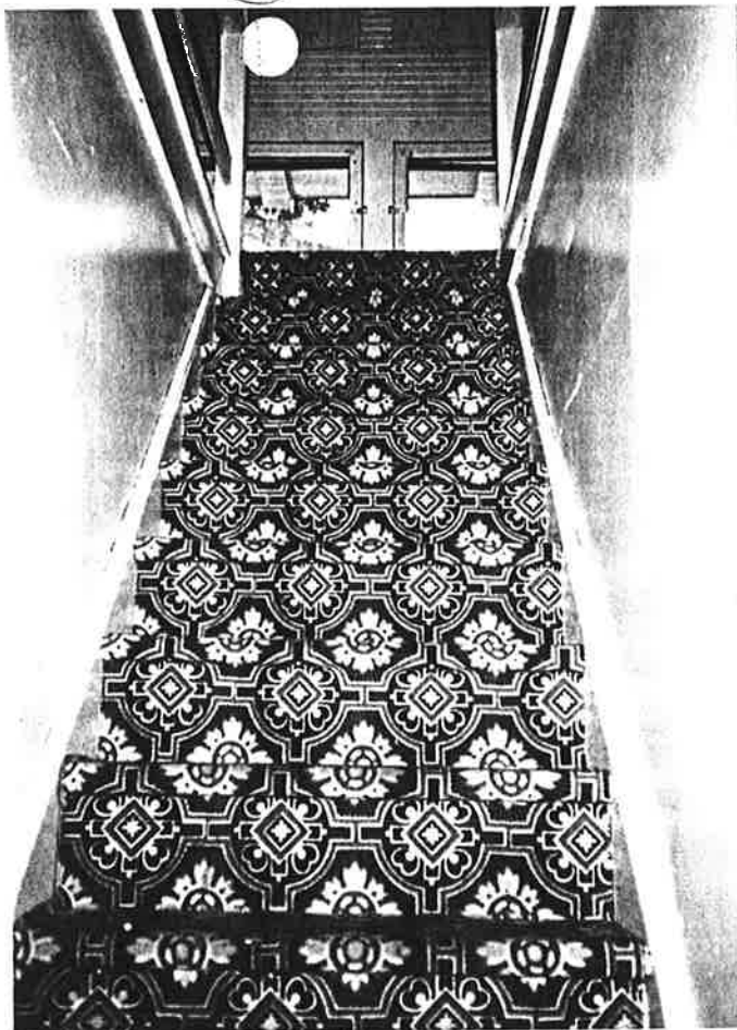
Stairway to 3rd Floor (looking S, 2/96)
