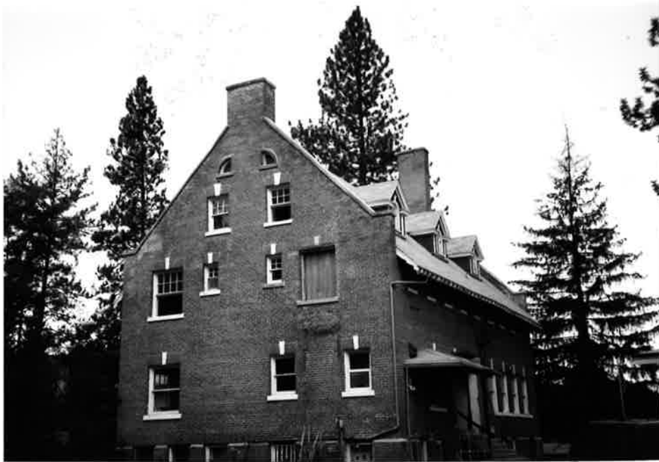
Photos 8 and 9 SW elevation.
