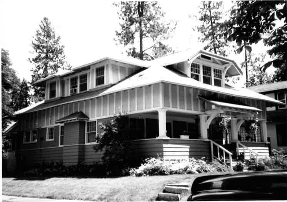
Photos 3 and 4 North elevation of house and rear, east elevation in 2006.
