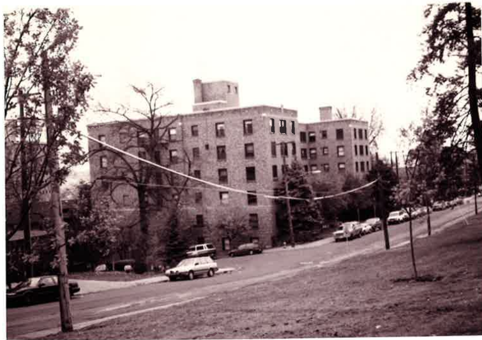
Photos 3 and 4: South facade and west elevation of building; 1999 photos.
