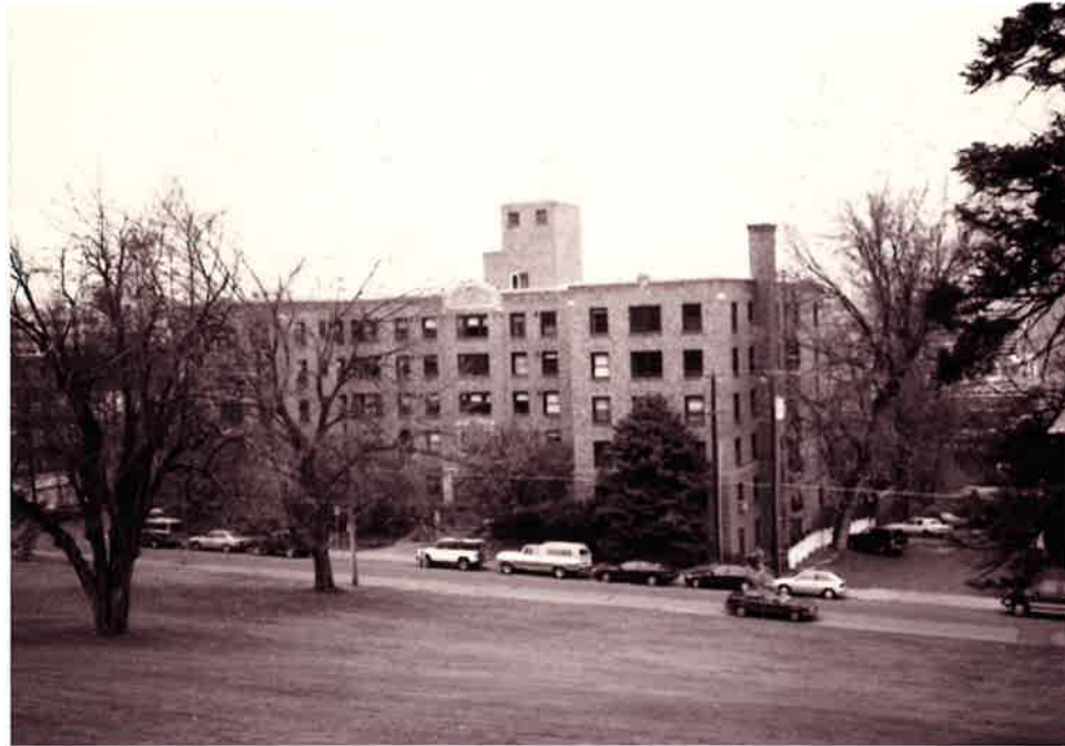
Photos 1 and 2: South facade of building; 1999 photos.
