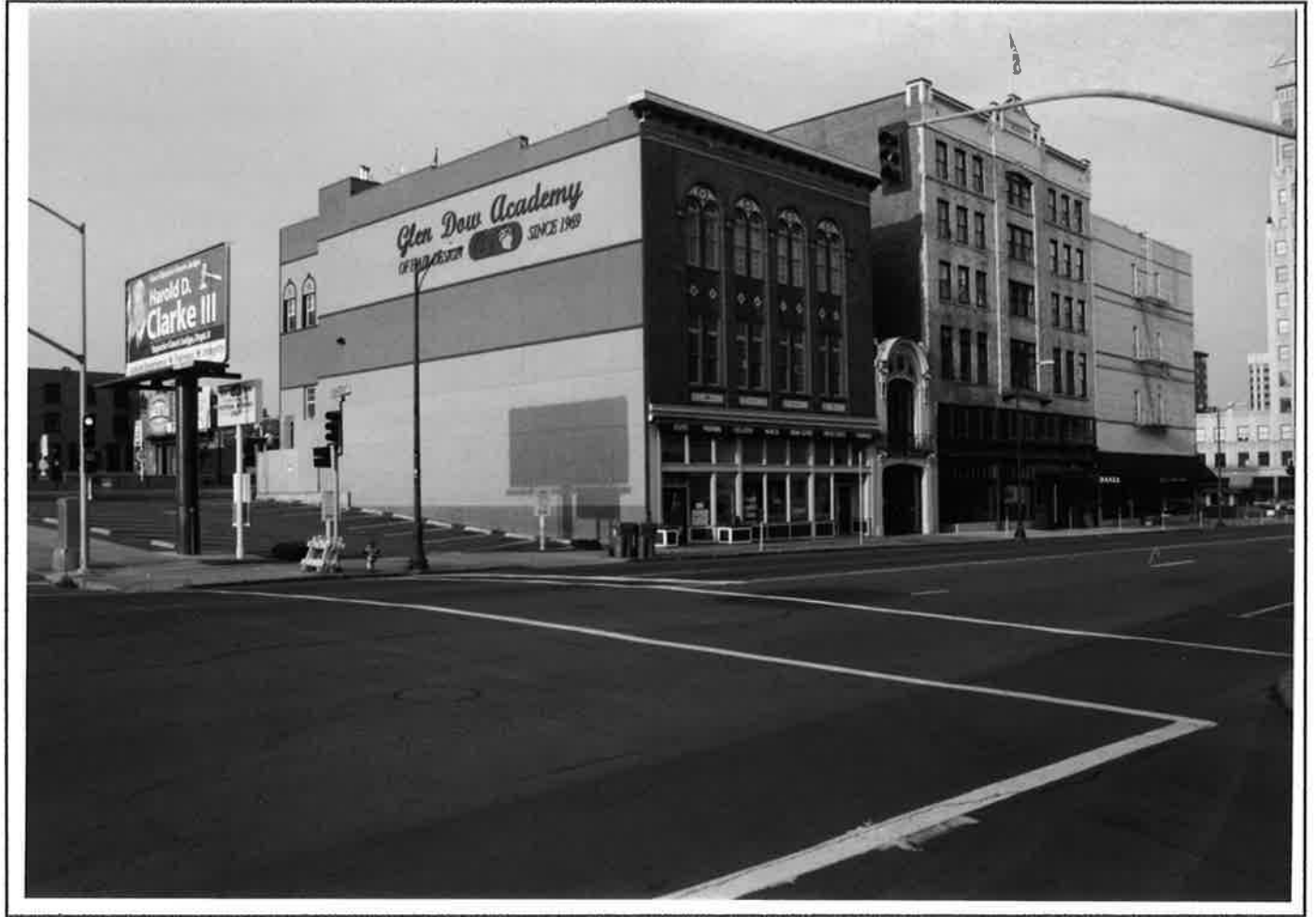
View to Southwest Showing Streetscape East of Glen Dow Buildings
