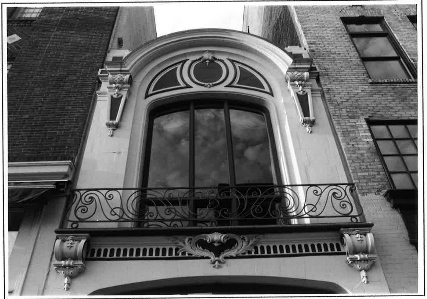
View to South Showing Front Facade Detail of Raznik Building
