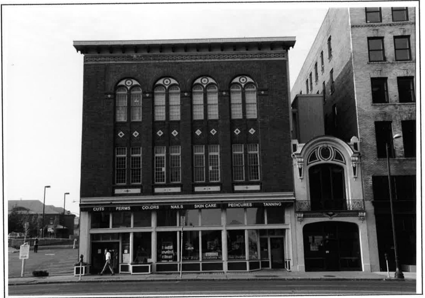
View to South Showing Front Facades of Glen Dow Buildings F.C. Robertson Building and Raznik Building
