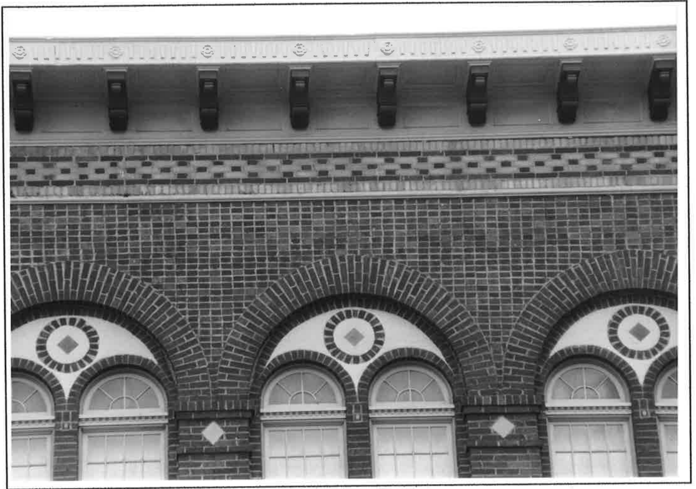
View to South Showing Front Facade Detail of F.C. Robertson Building
