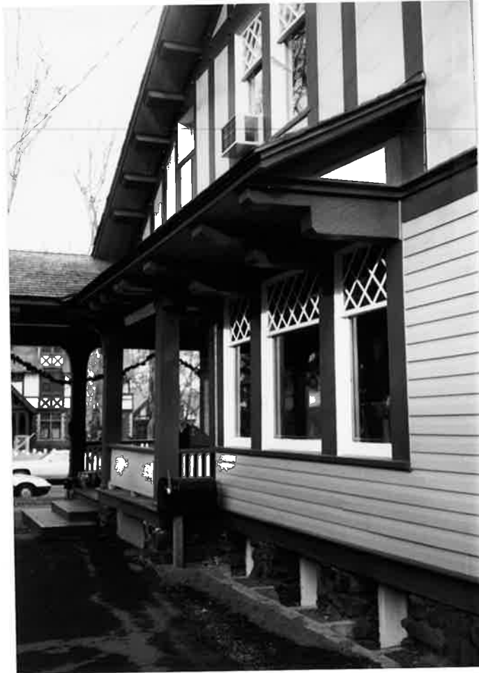
Photos 9 and 10: West elevation of house.
