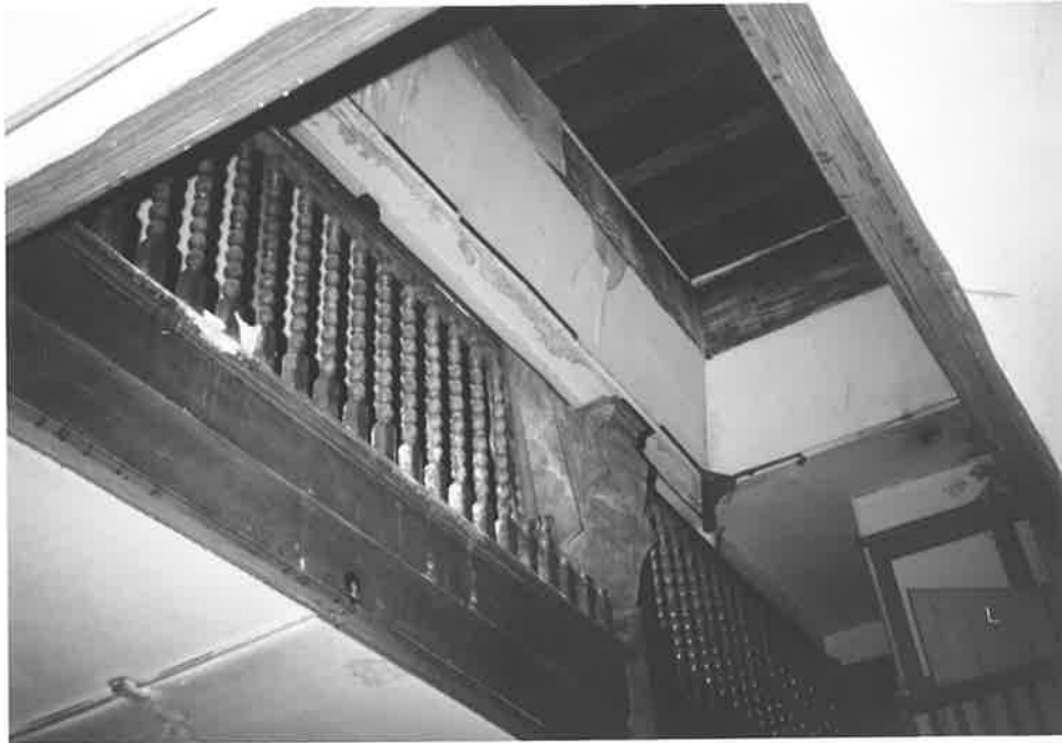
Stairwell to third floor.
