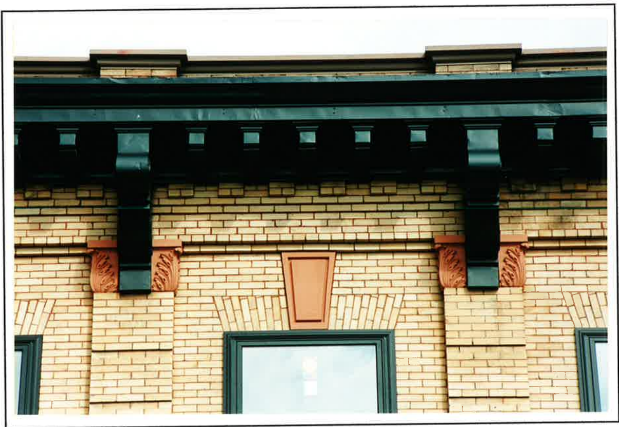
View to North, Front Facade Window Head, Capitals, Brackets, Cornice
