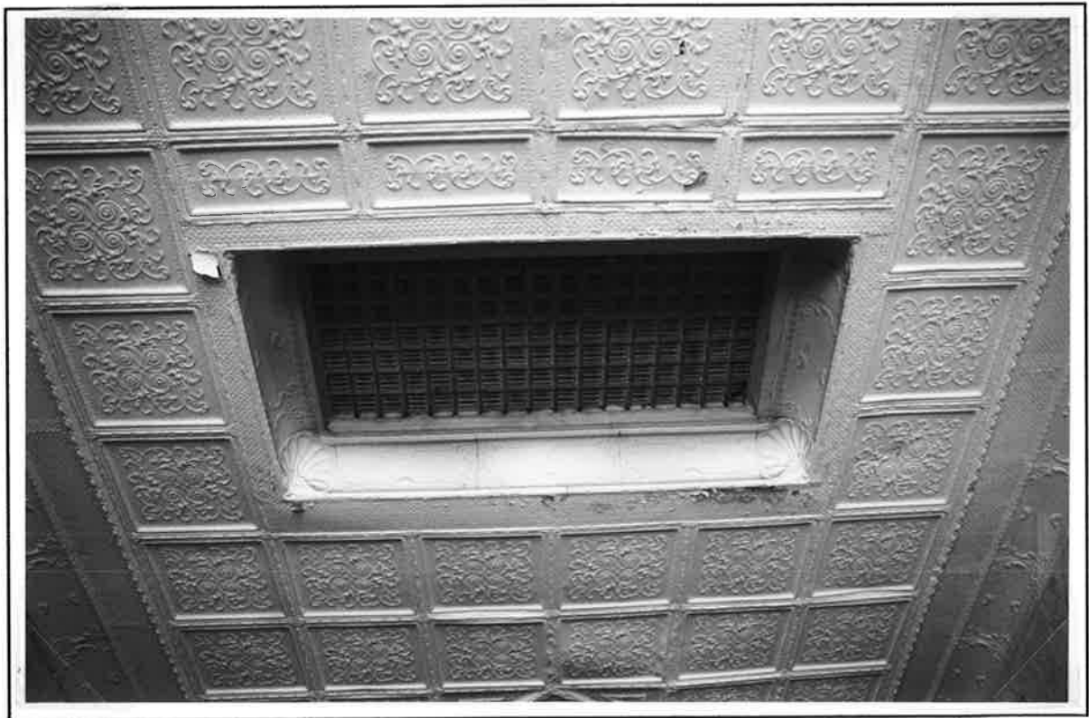
Detail of Pressed Tin Ceiling in West 1st Floor Bay - Sky Light
