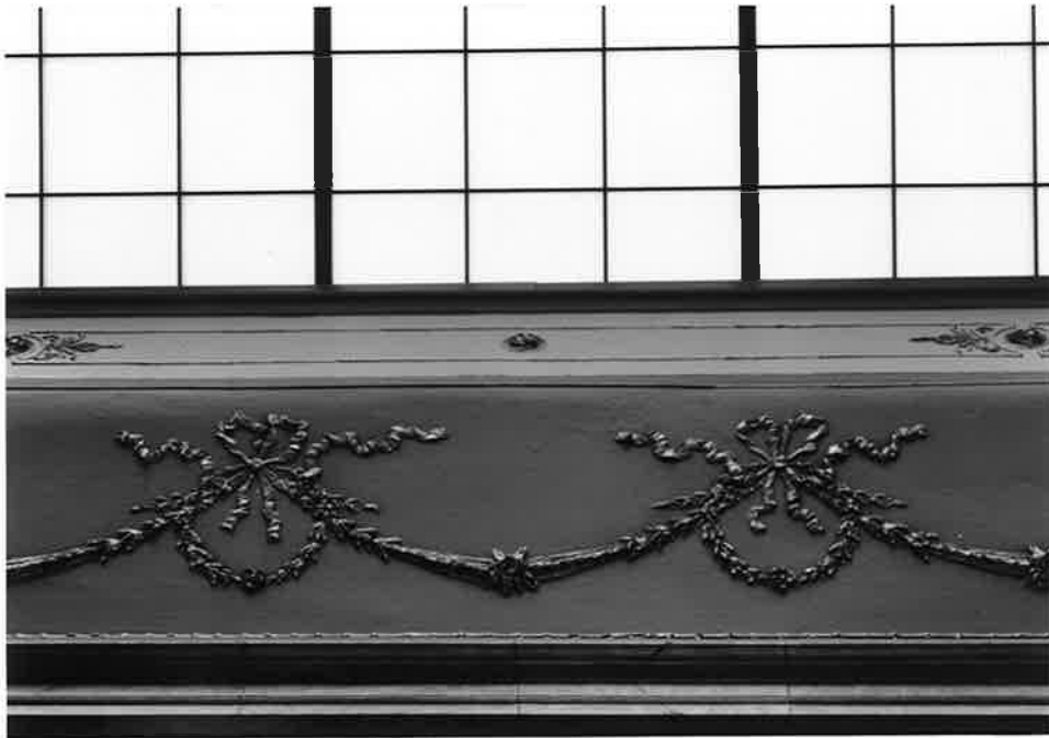
Photos 15 and 16 Interior hallways on second and third floors; photos taken in 2003.
