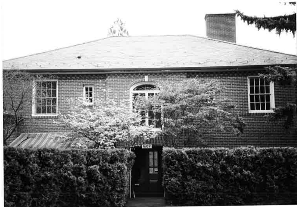
Photos 3, 4, 5 West facade of Jensen House.
