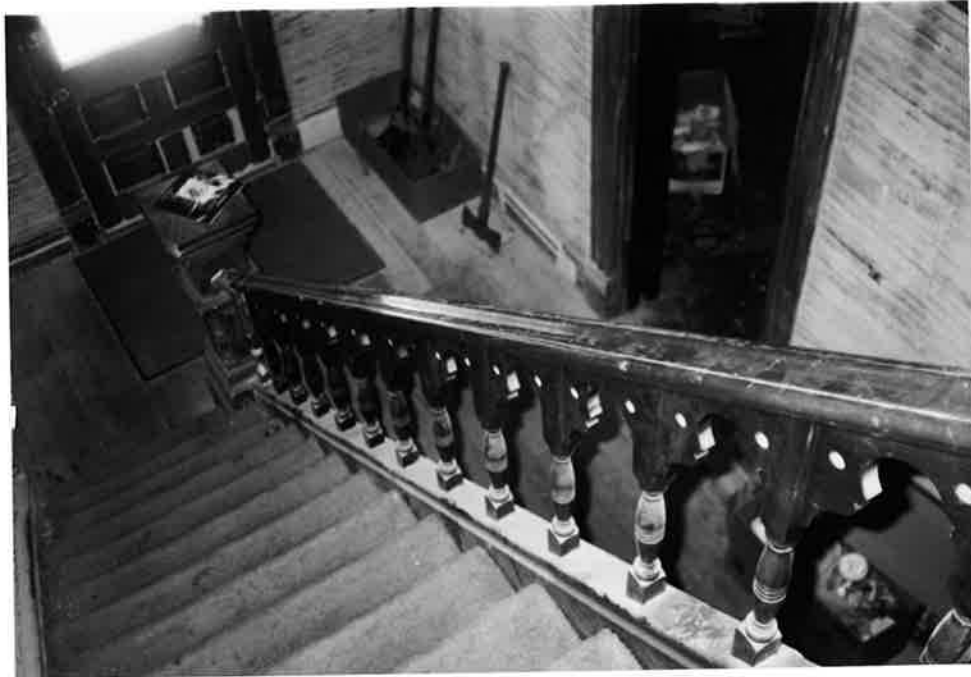
Photos 7, 8 and 9: Front entry on first floor--staircase and newel post.
