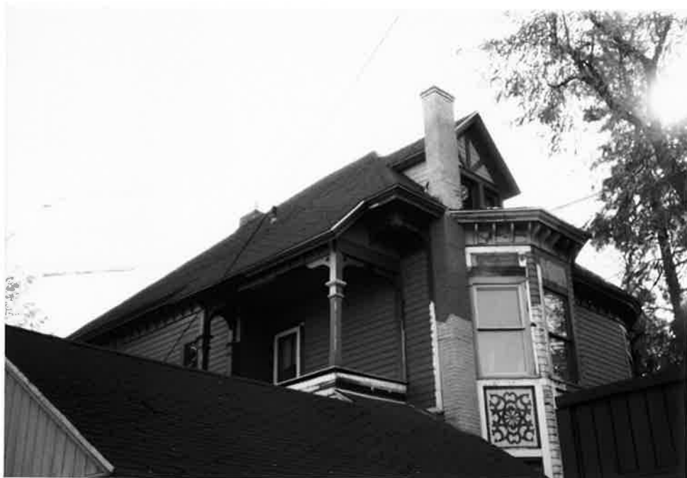
Photos 5 and 6: North, rear elevation of house (1999 photos).
