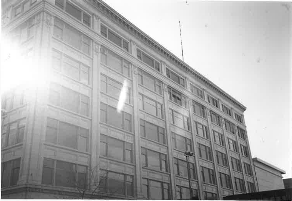
NORTHEAST CORNER - CRESCENT COURT
