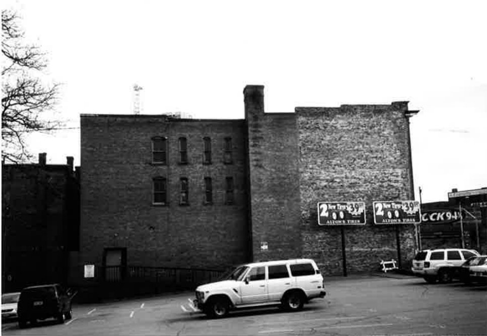
Photos 10 and 11 West elevation (rear of building).
