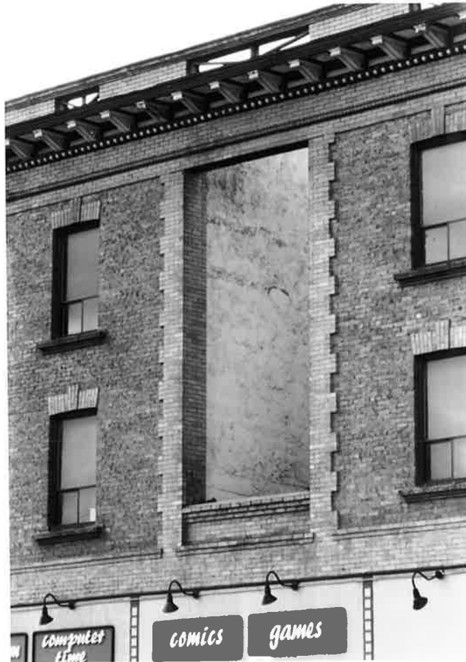
Photos 3 and 4 East facade; second and third floors.
