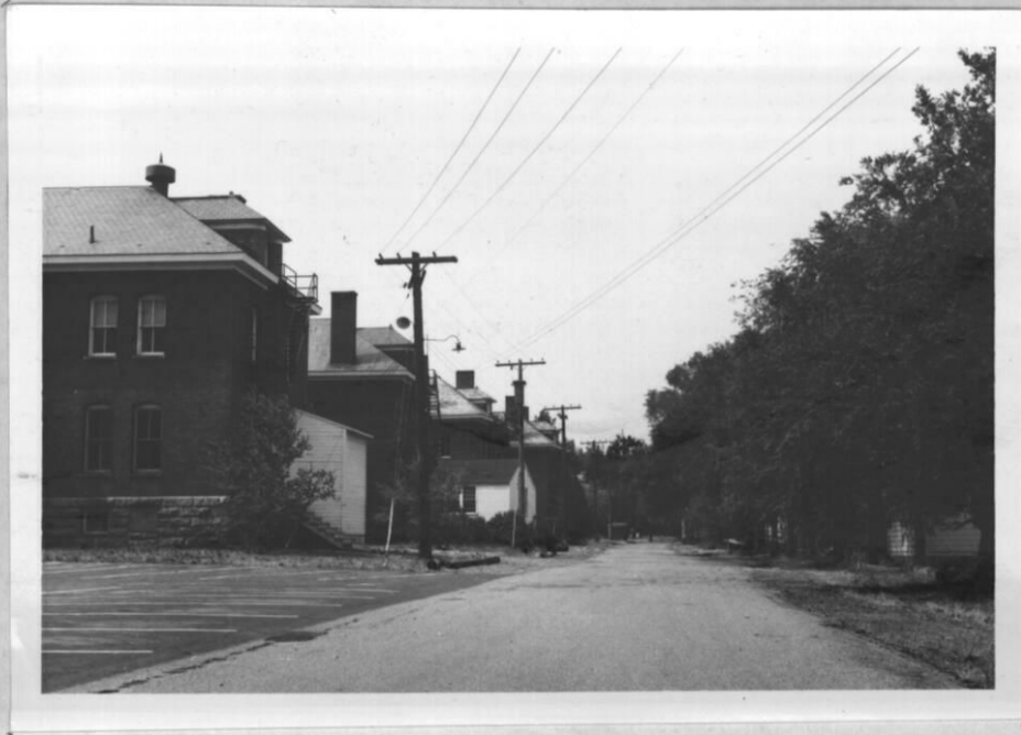
A view of the rear of Barracks buildings (Buildings 25 and 27) on left. On the right, in between the trees, are temporary structures (Buildings T 31, 32, 33).
