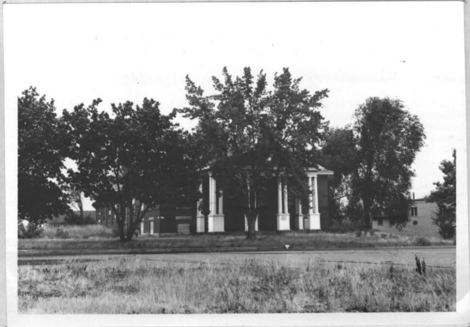
The Post Exchange (Building 100) which we would plan to redecorate on the interior and use as a museum interpreting the history of this area.
