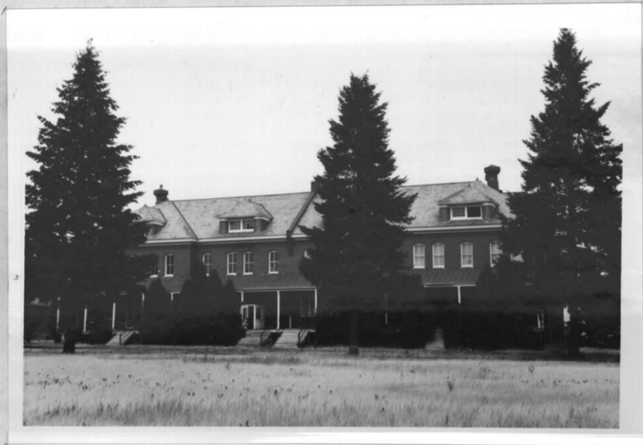
Photograph of the Barracks Building (Building 27)
