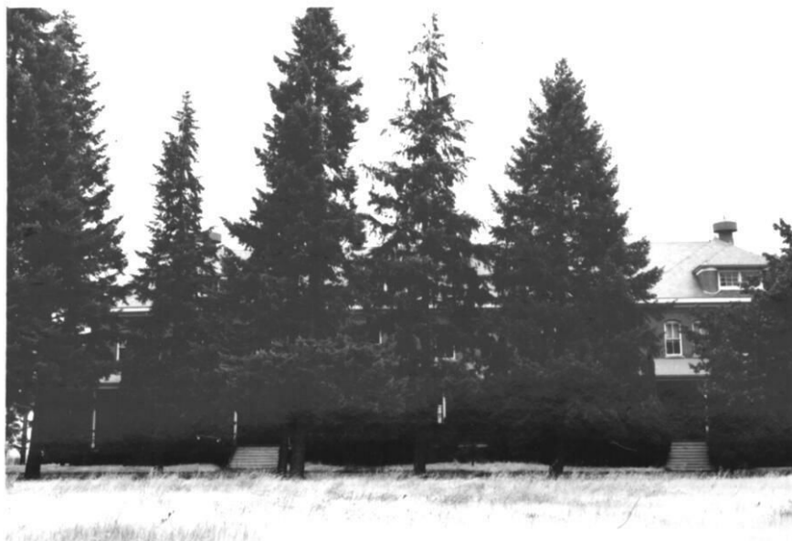
Photograph of the Barracks structures (Building 25)
